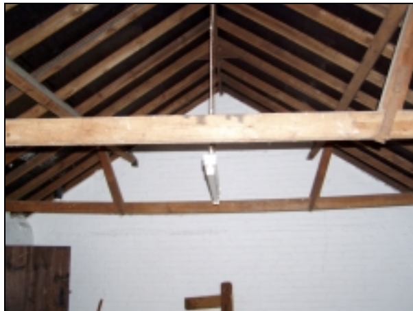
Plate 19: Roof, Room 1F10
