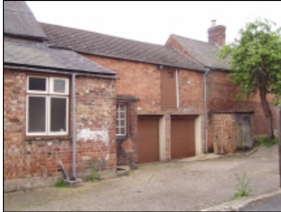
Plate 17: Rear of complex, looking southwest
