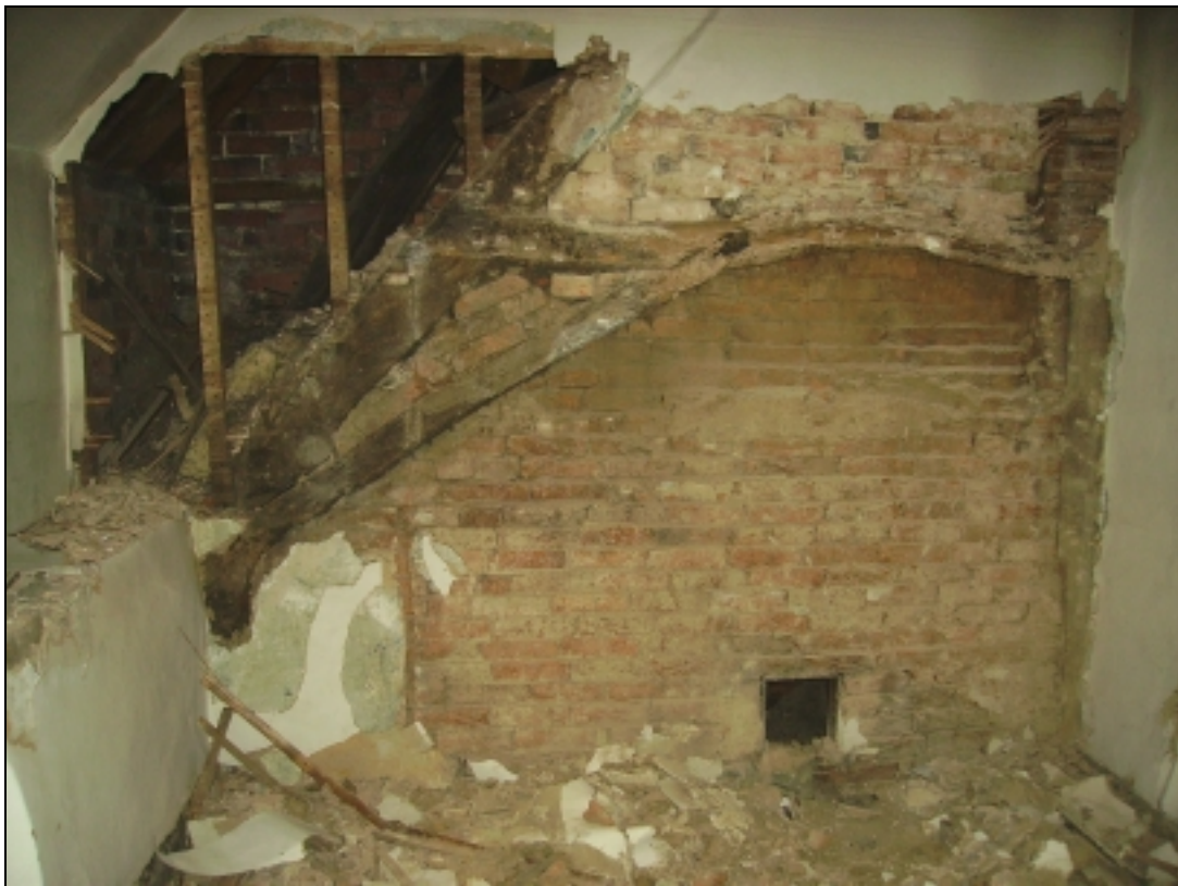
Plate 11: Blocked fireplace and original roof line, Room 1F1
