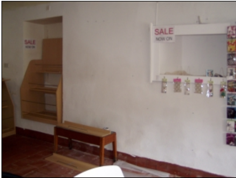
Plate 6: Blocked door and window, north wall of 2, Church Street. Looking northwest
