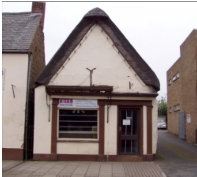
Plate 4, Front of 4, Church Street, looking west
