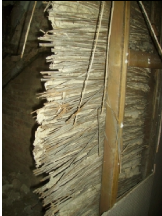
Plate 10: sample of reed and plaster walling
