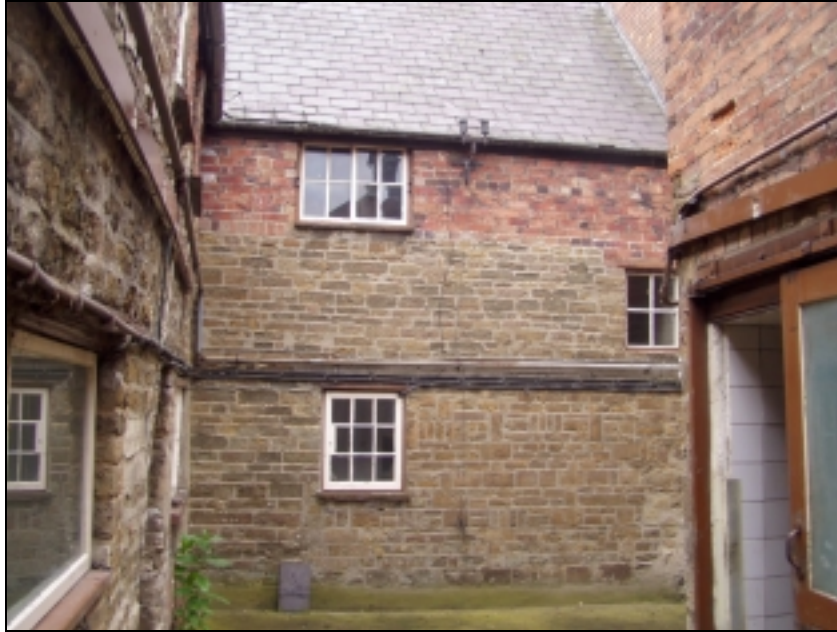
Plate 8: Rear of Cottage, 4, Church Street
