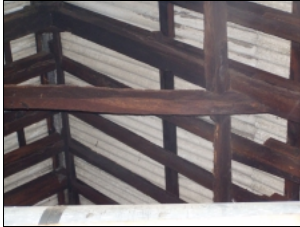
Plate 14: Roof of old bakehouse, Room 1F8
