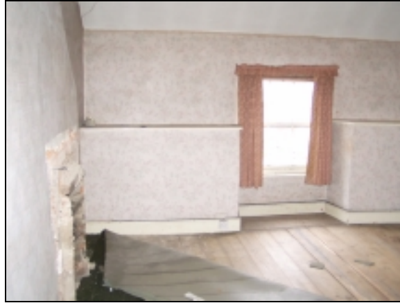
Plate 12: first floor, cottage, Room 1F2
