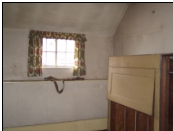
Plate 16: First floor of the Link Building; Room 1F6
