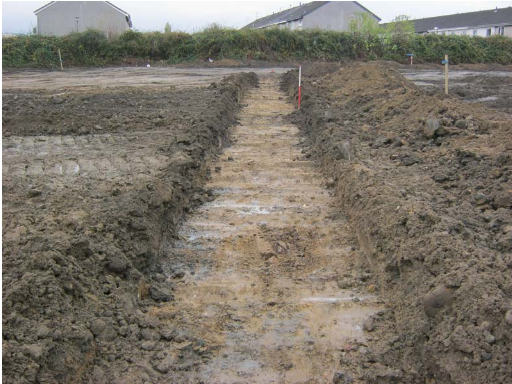
Plate3 Trench 5 post excavation from north-east
