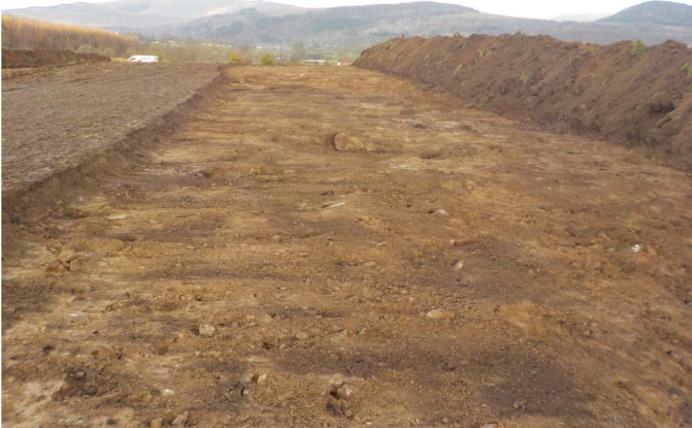
Plate 2 - General view of eastern edge of stripped area
