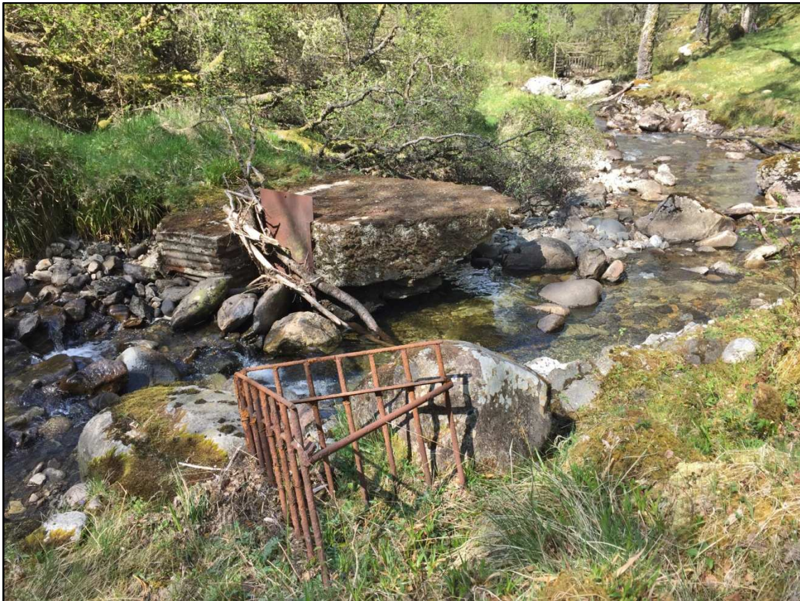
Plate 9 NW view over disused weir, Site 13
