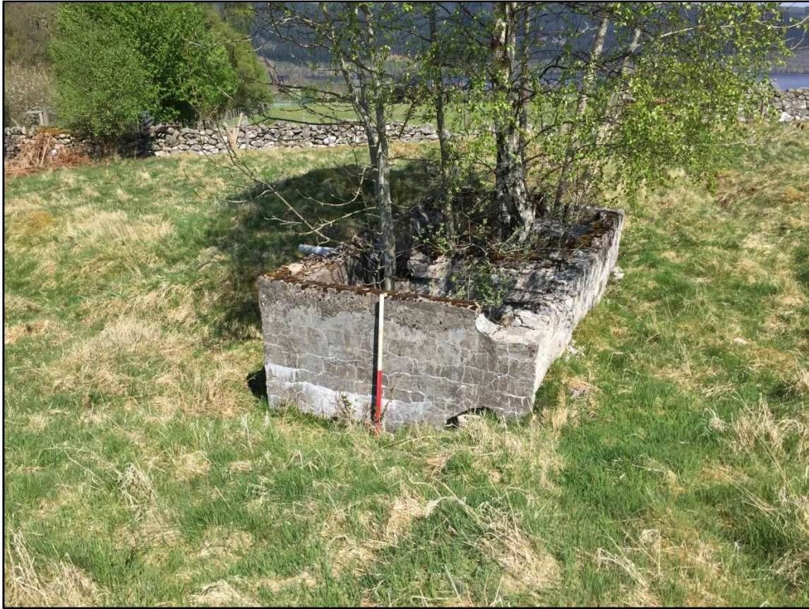
Plate 8 Looking S over concrete-built tank, Site 5
