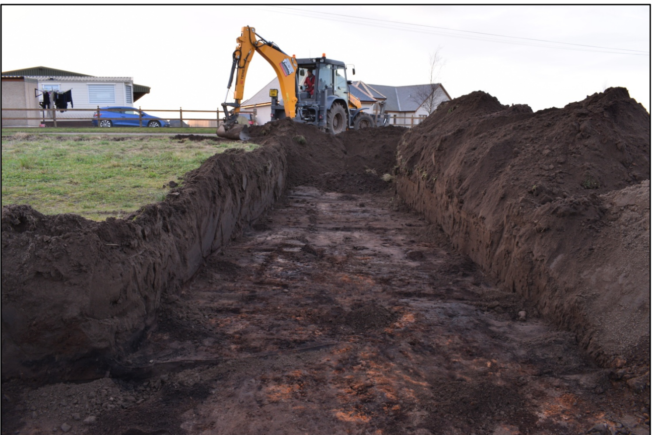
Plate 7: Stripping in progress over the access footprint, looking W
