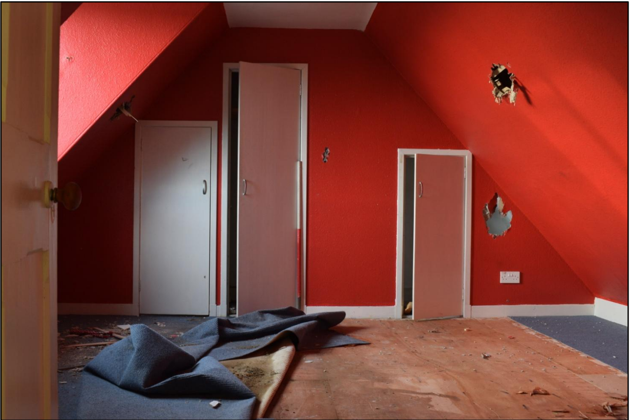
Plate 9: Room in the roof space, W cottage
