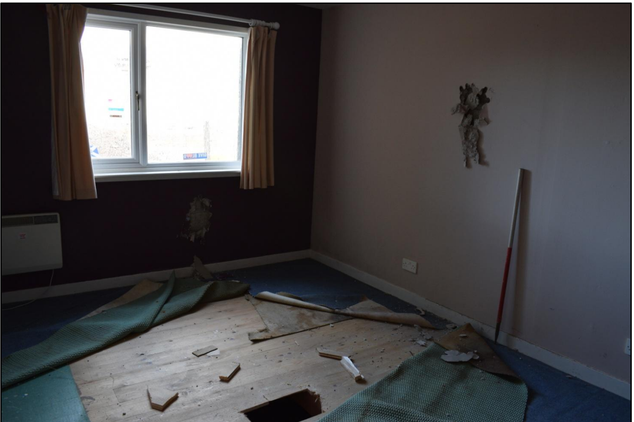
Plate 12: Rear bedroom, W cottage
