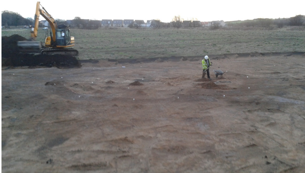
Plate 1 The Barrow [06] being cleaned before excavation
