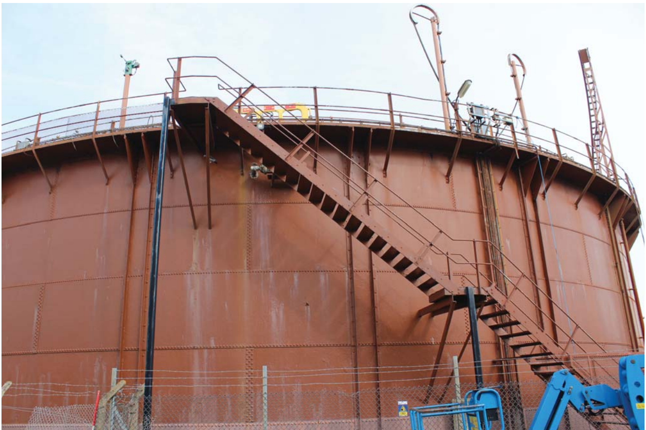
Plate 16: Sea Street, Herne Bay, detail of the stairs from the south
