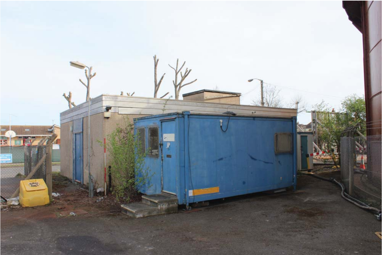
Plate 25: Sea Street, Herne Bay, general view of additional ancillary gasworks buildings to the north-west of the gasholder, from the south-west
