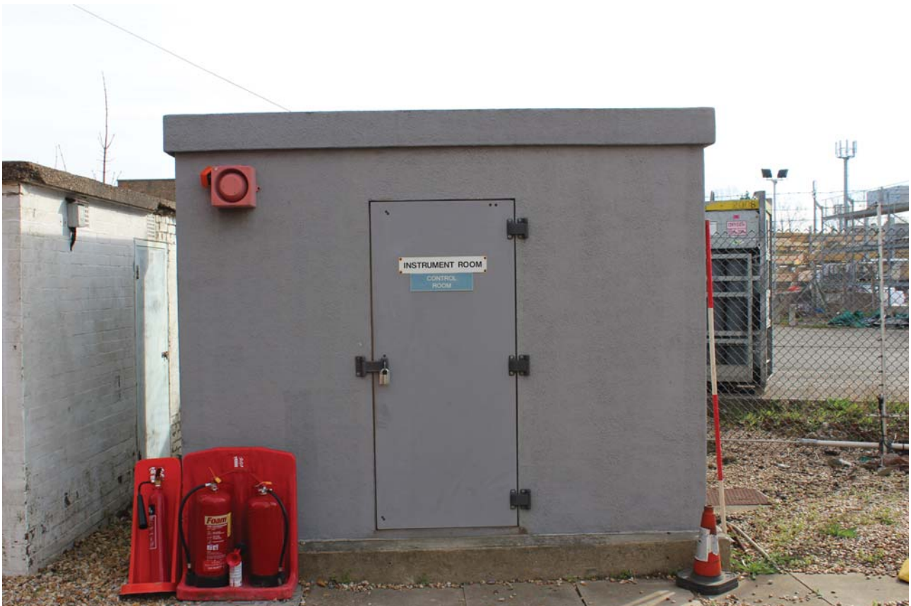
Plate 20: Sea Street, Herne Bay, general view of the Instrument Room/Control Room from the SWW
