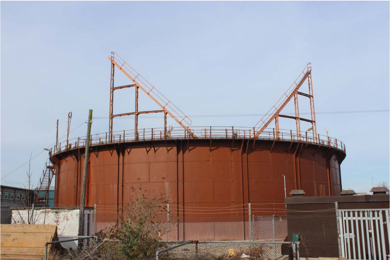
Plate 3: Sea Street, Herne Bay, general view of the gasholder from the east
