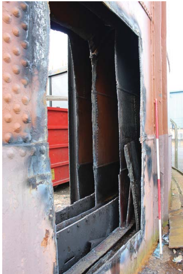
Plate 10: Sea Street, Herne Bay, detail of the section cut through the side of the gasholder from the NNW
