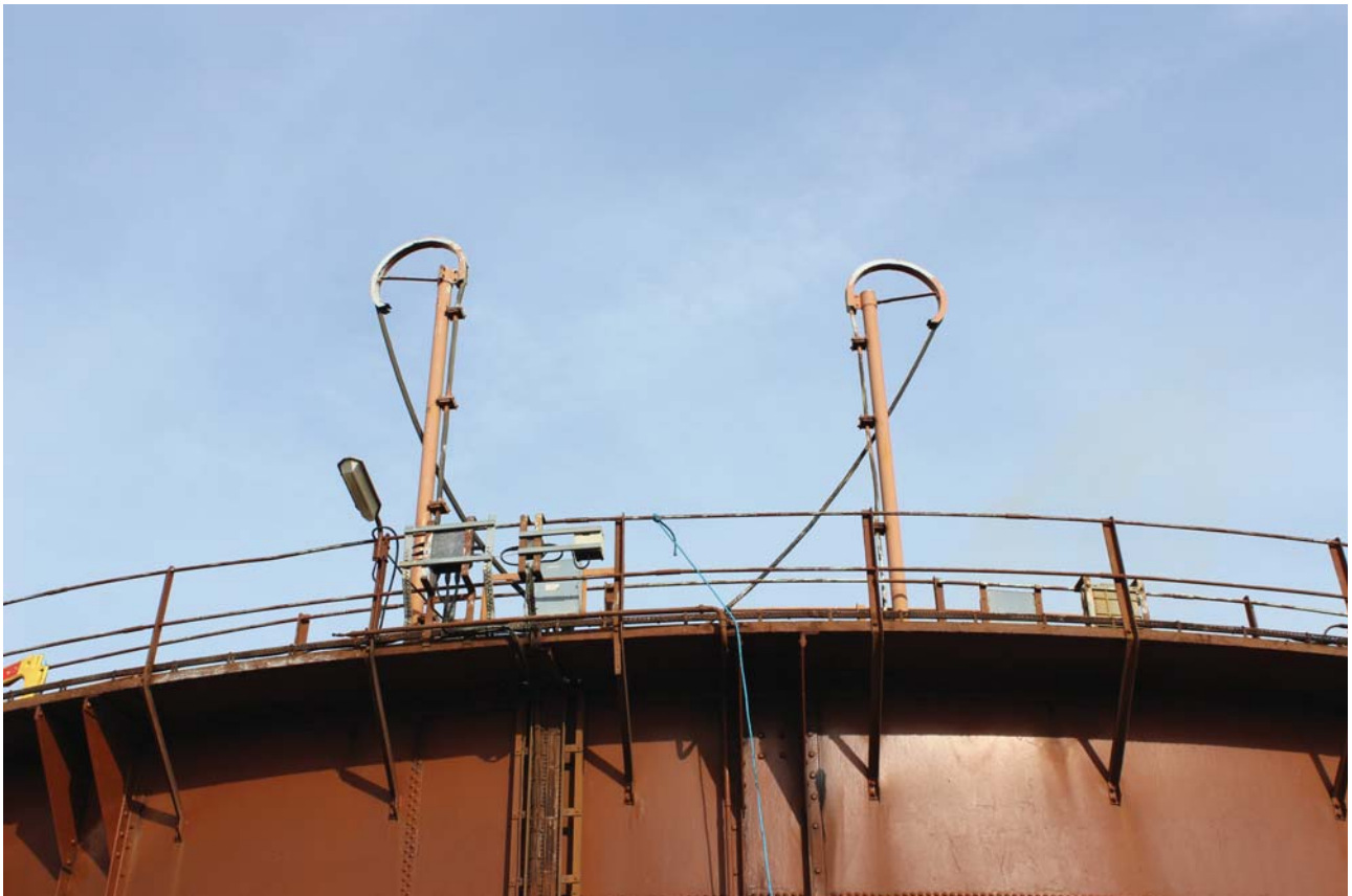
Plate 12: Sea Street, Herne Bay, detail of the upper walkway from the south-east
