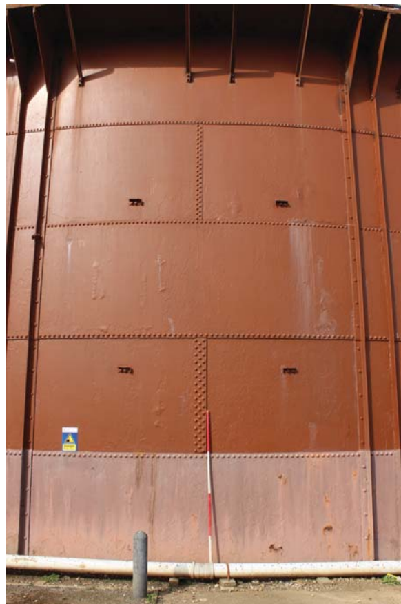
Plate 6: Sea Street, Herne Bay, detail of the gasholder showing the riveted plates, from the SEE
