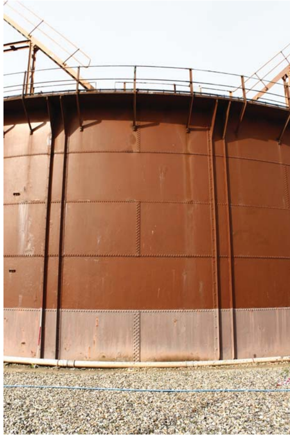
Plate 11: Sea Street, Herne Bay, general view showing the stanchions supporting the upper walkway, from the east
