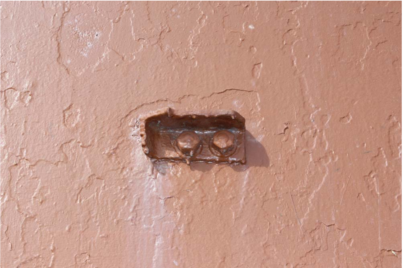
Plate 9: Sea Street, Herne Bay, close detail of the riveted bracket from the east
