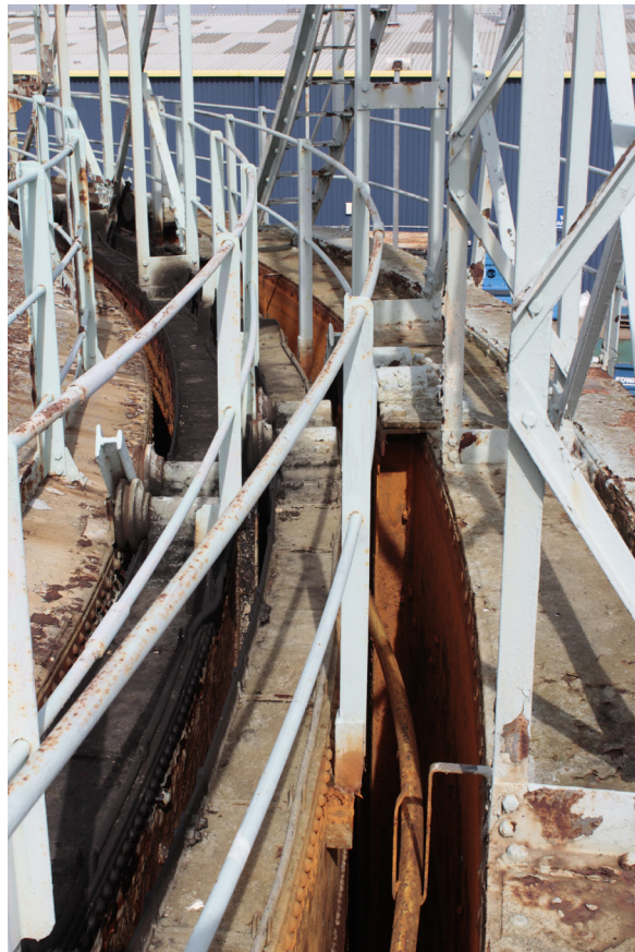
Plate 18: Gasholder No 4, detail of the lift mechanism from the SSW
