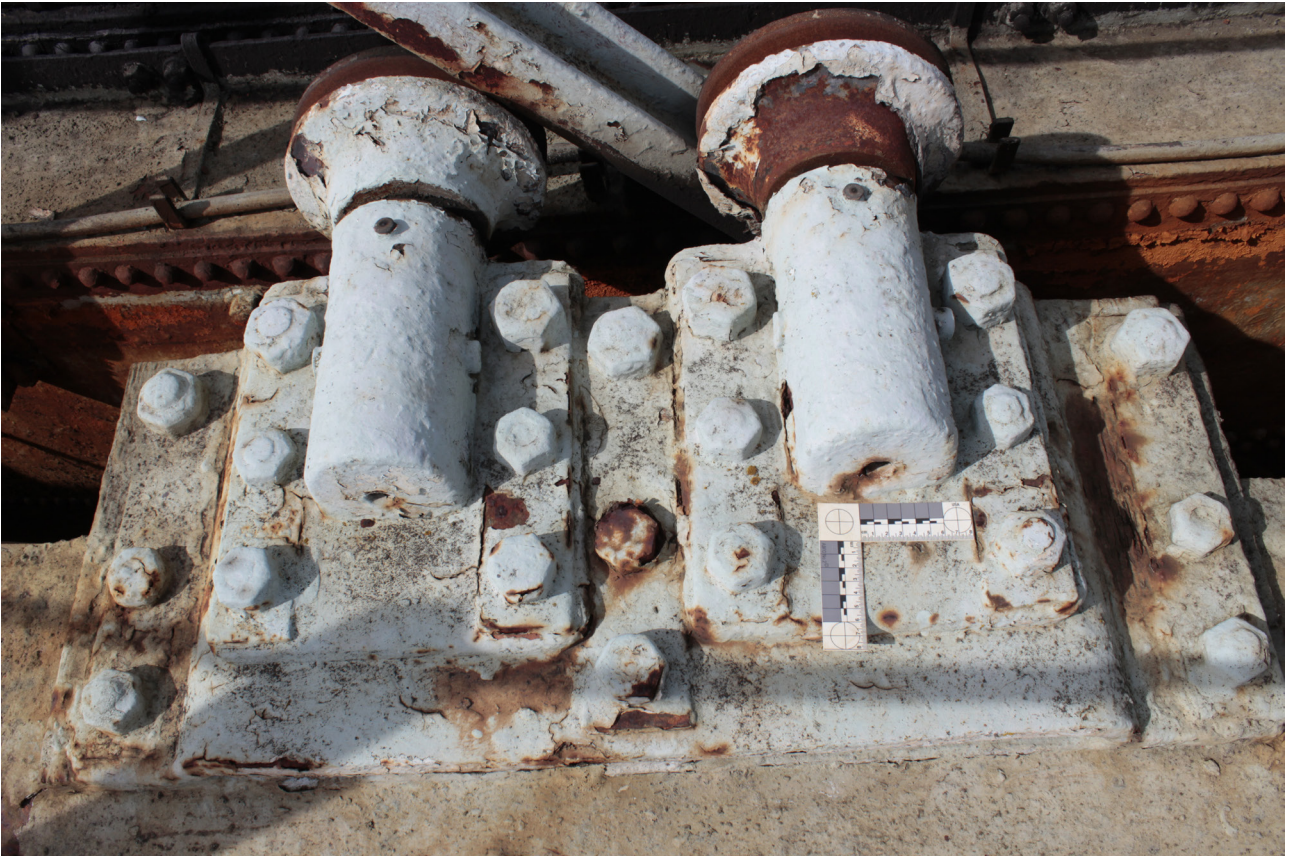
Plate 19: Gasholder No 4, detail of the lift mechanism from the south-east
