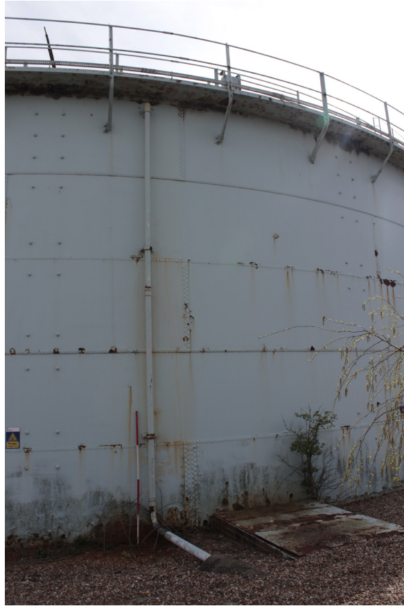
Plate 5: Gasholder No 4, general view from the NNW
