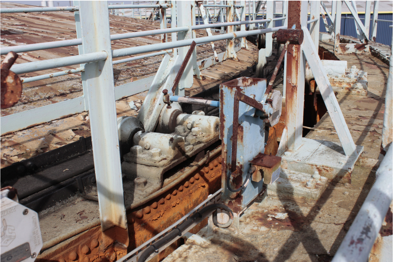
Plate 17: Gasholder No 4, detail of the lift mechanism from the south
