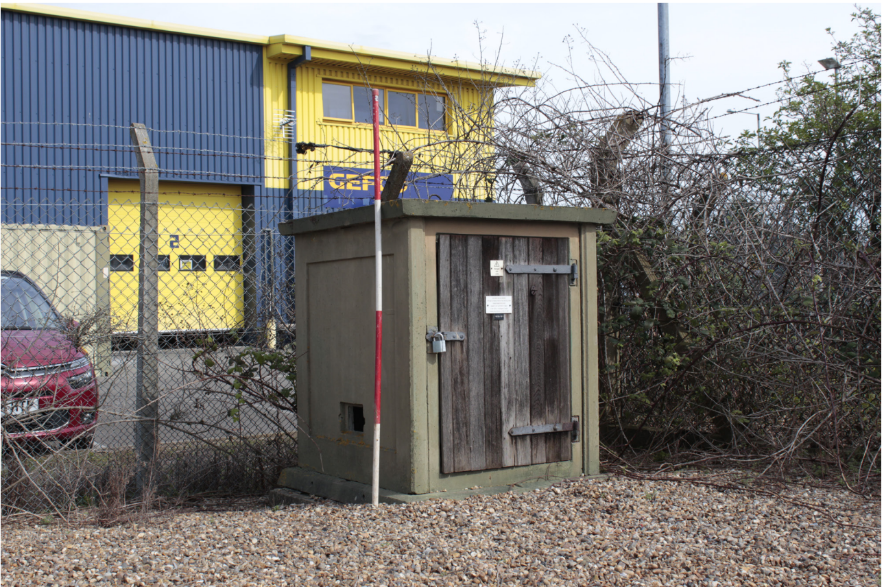
Plate 44: General view of gasworks building from the west
