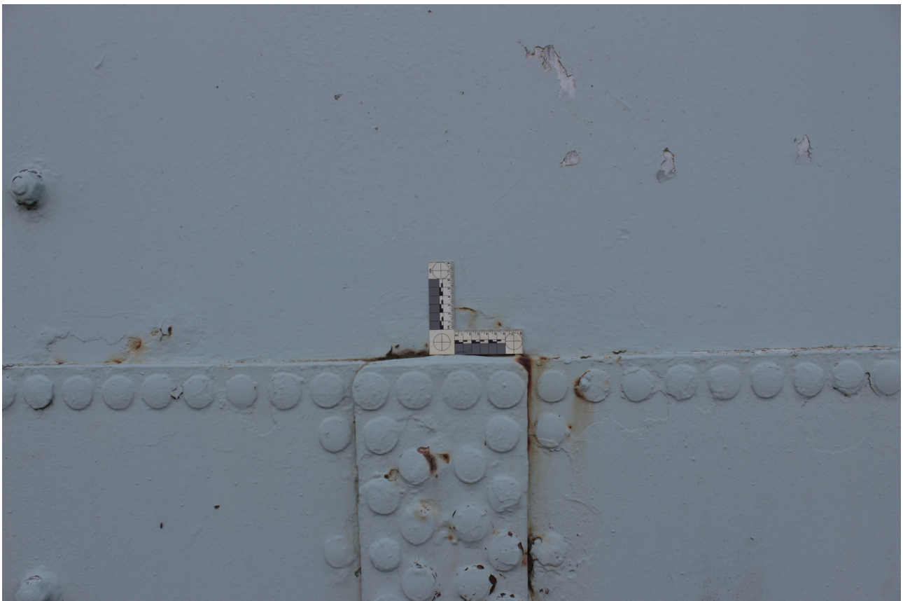
Plate 8: Gasholder No 4, close detail of steel plate from the north
