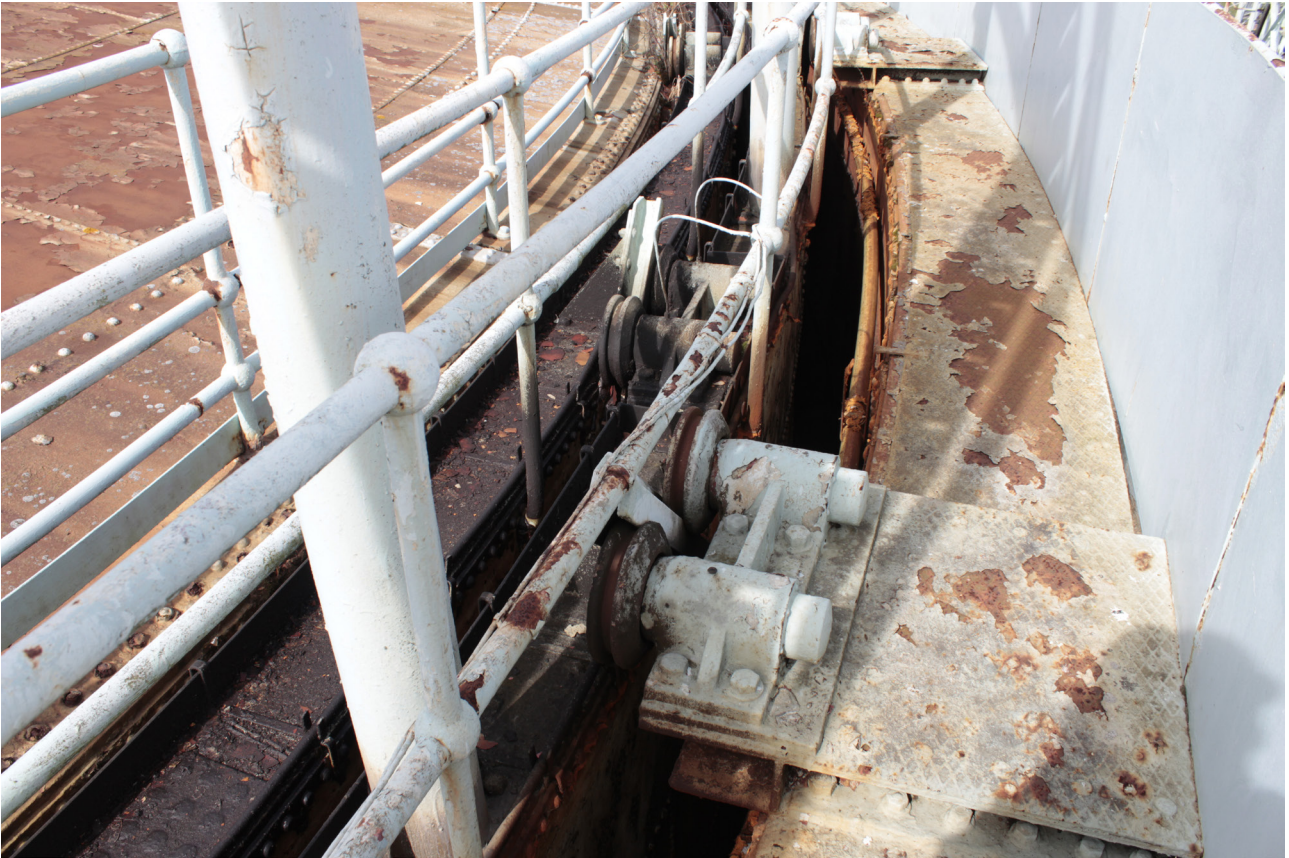
Plate 37: Gasholder No 5, detail of the lift mechanism from the south
