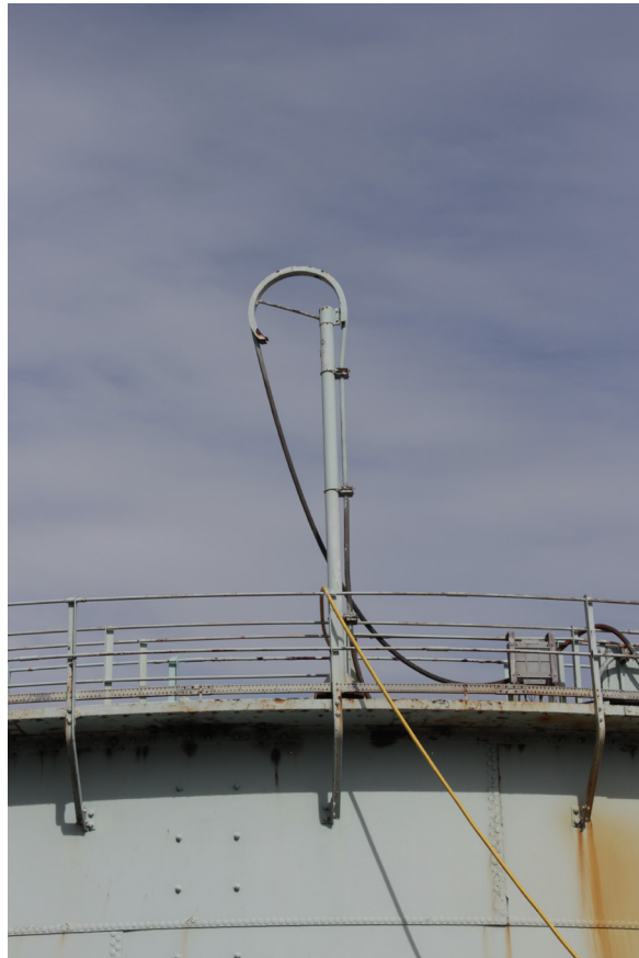
Plate 9: Gasholder No 4, detail of upper walkway from the south
