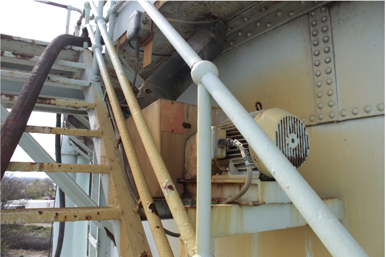
Plate 31: Gasholder No 5, detail of electric motor and pump at the top of the stair from the NNE
