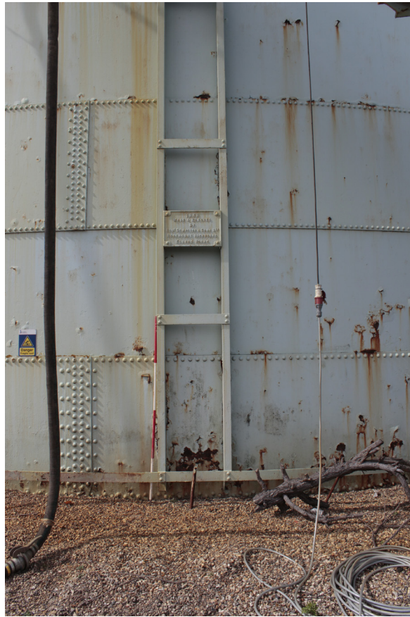
Plate 23: Gasholder No 5, detail of stanchion from the east
