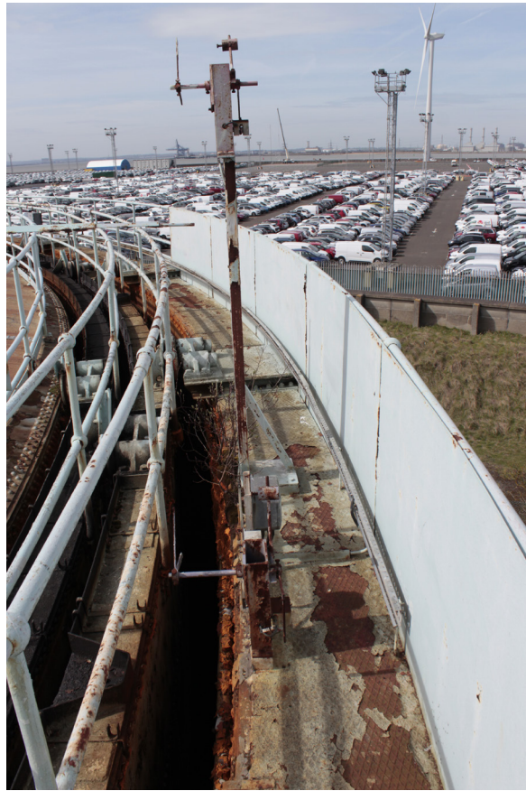
Plate 35: Gasholder No 5, detail of the lift mechanism from the west
