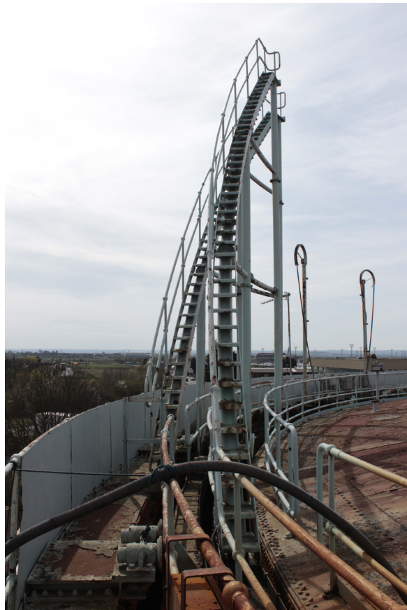
Plate 34: Gasholder No 5, detail of the lift mechanism from the NNE
