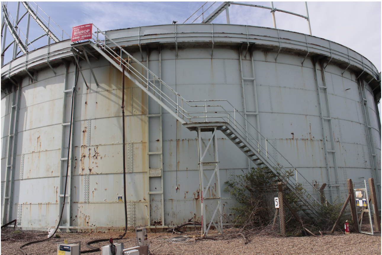
Plate 29: Gasholder No 5, general view showing stair from the east
