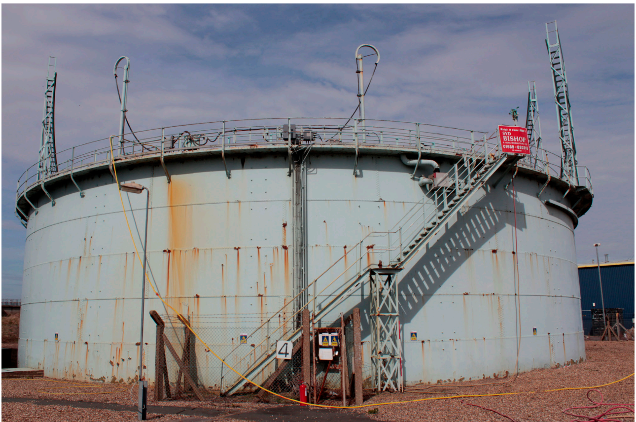
Plate 10: Gasholder No 4, general view showing the stair from the south
