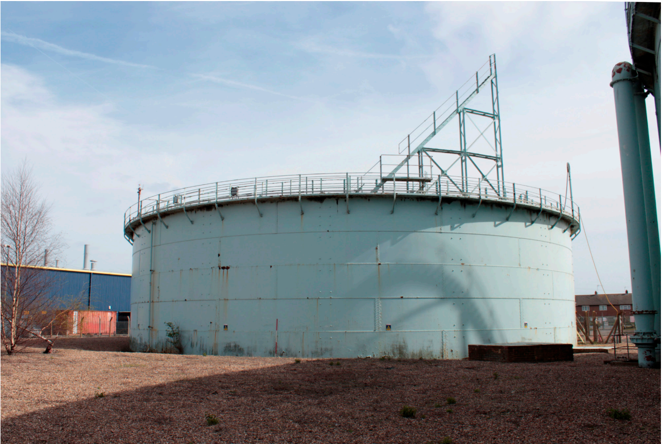
Plate 3: Gasholder No 4, general view from the west
