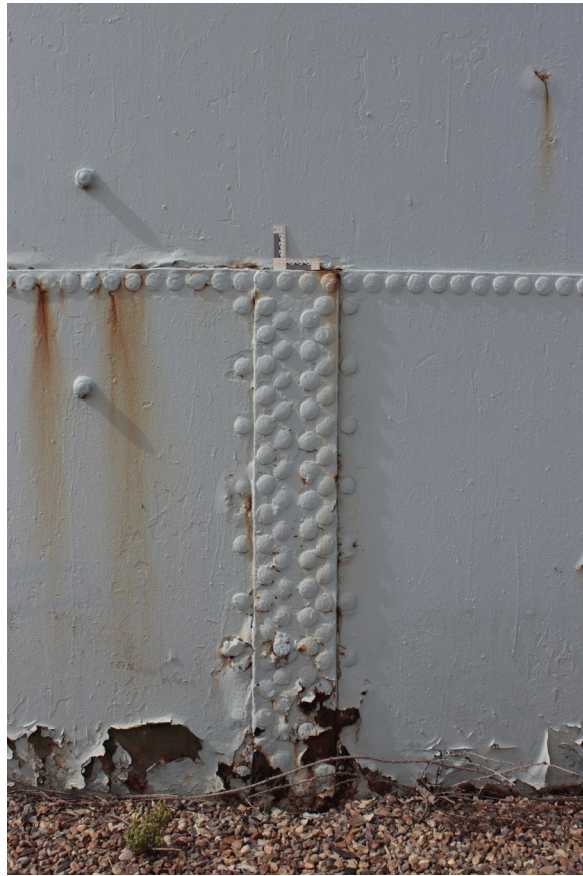
Plate 7: Gasholder No 4, detail of steel plate from the north
