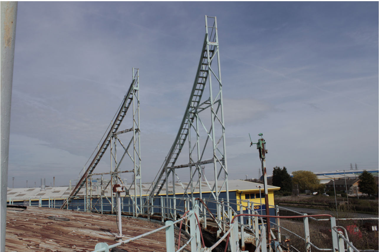
Plate 14: Gasholder No 4, general view of the top of the gasholder from the south-west
