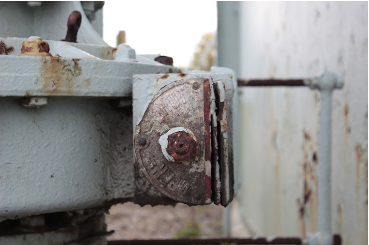
Plate 28: Gasholder No 5, detail of pipe from the north-west
