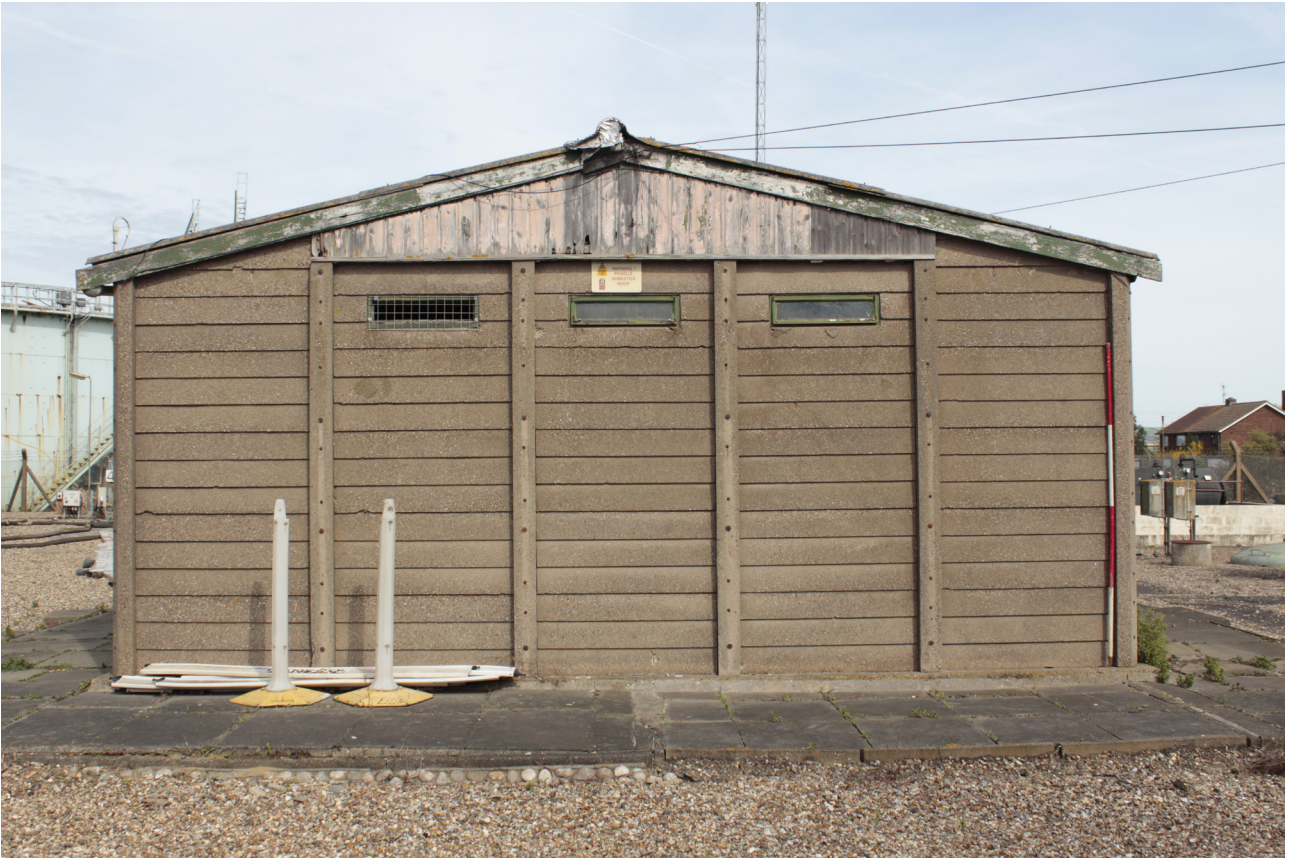
Plate 43: General view of gasworks building from the south-west
