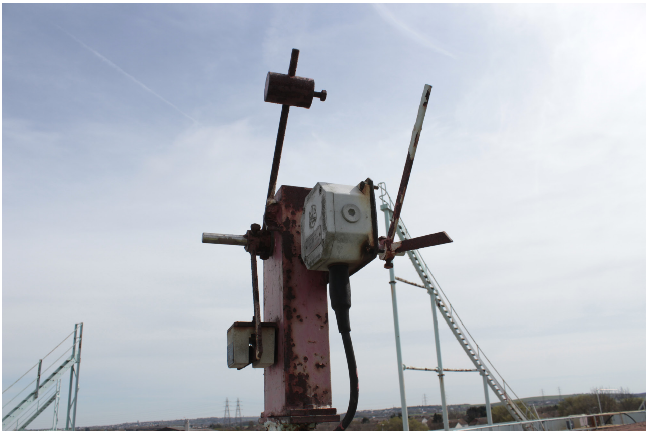
Plate 36: Gasholder No 5, detail of the lift mechanism from the NNW
