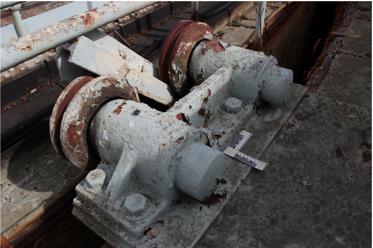
Plate 38: Gasholder No 5, detail of the lift mechanism from the west
