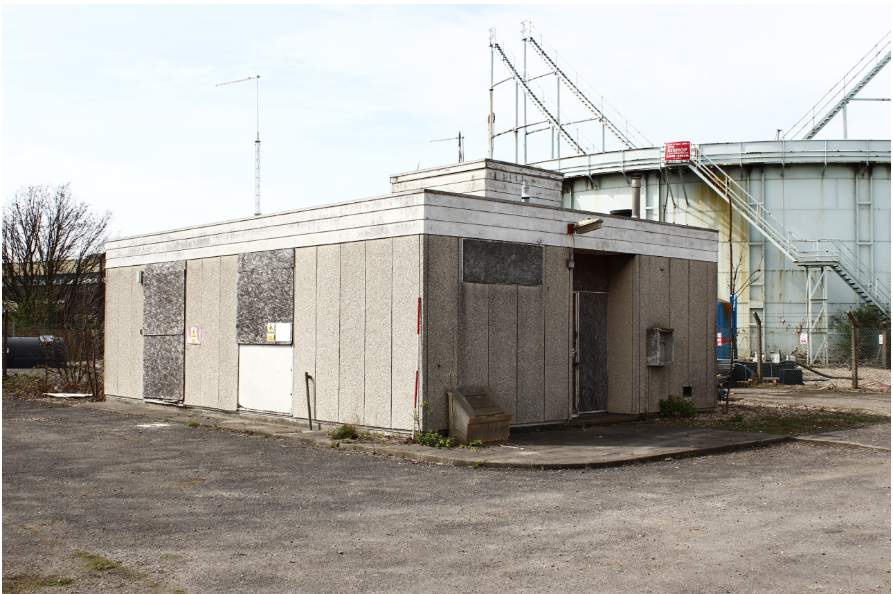
Plate 40: General view of gasworks building from the west
