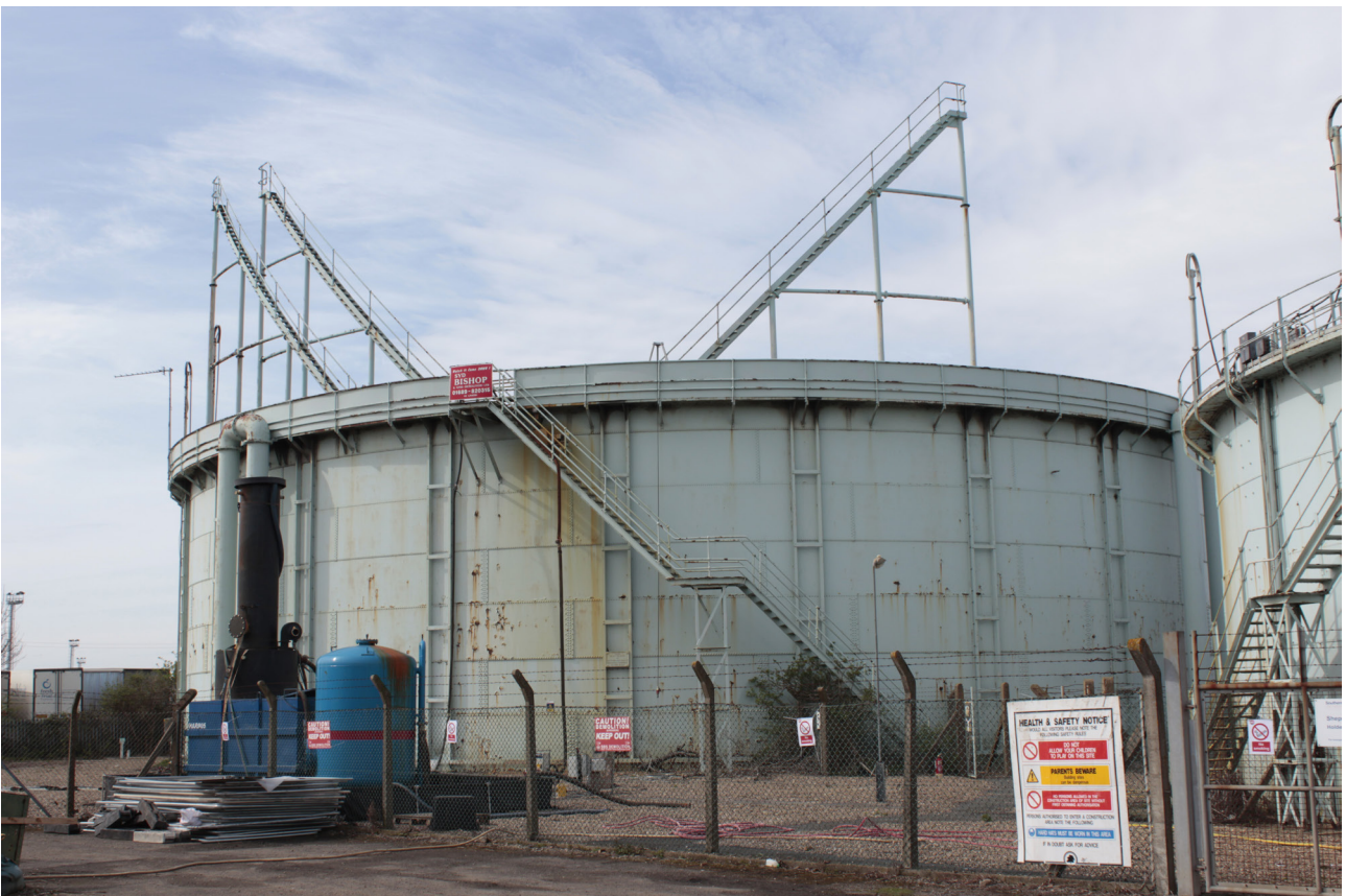
Plate 20: Gasholder No 5, general view from the east
