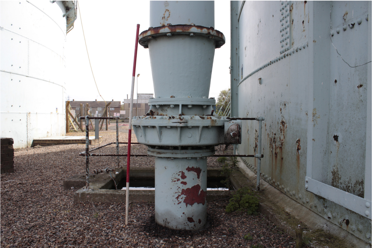
Plate 27: Gasholder No 5, detail of pipe from the north-west
