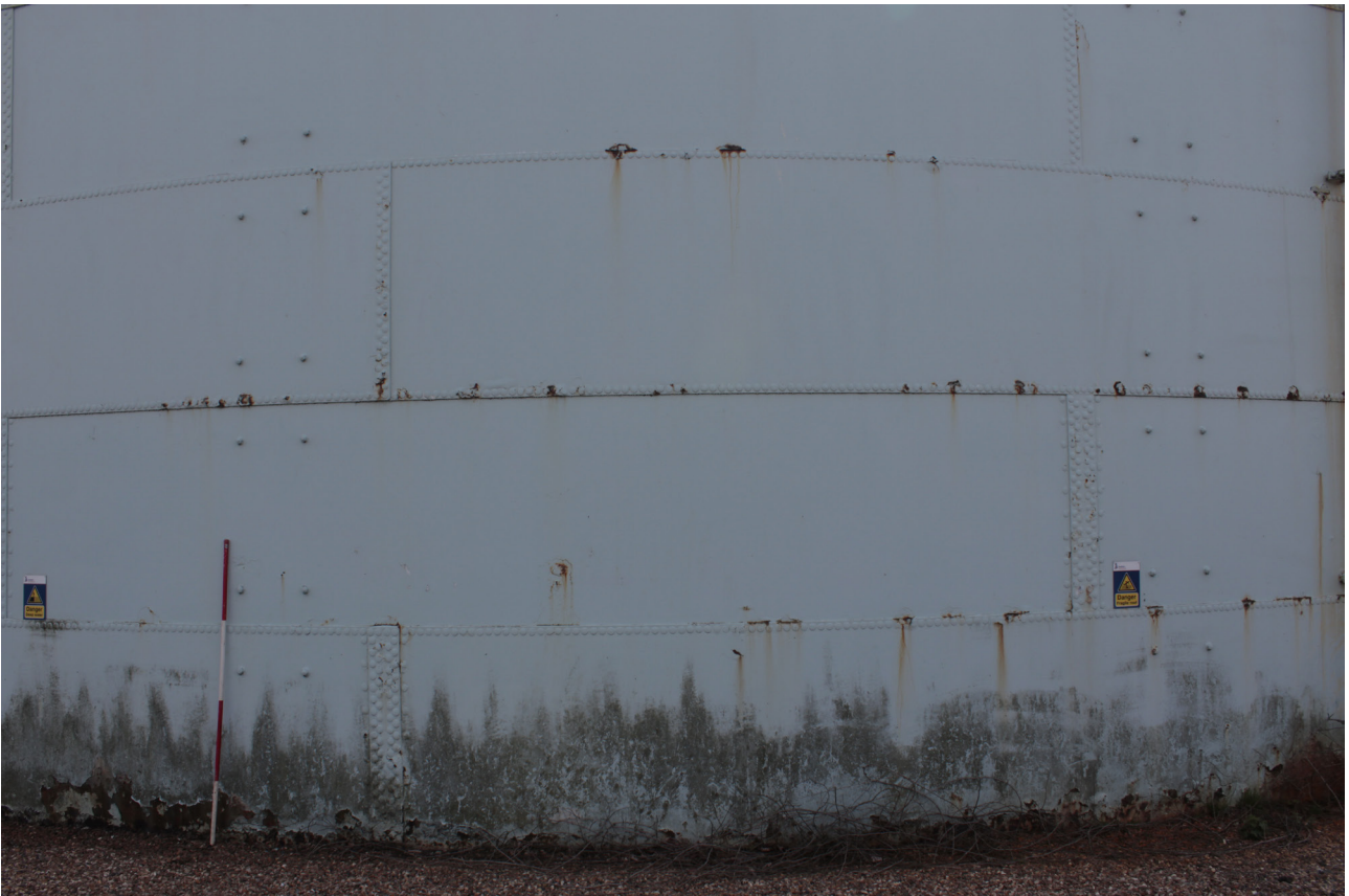
Plate 6: Gasholder No 4, detail of steel plate construction from the north
