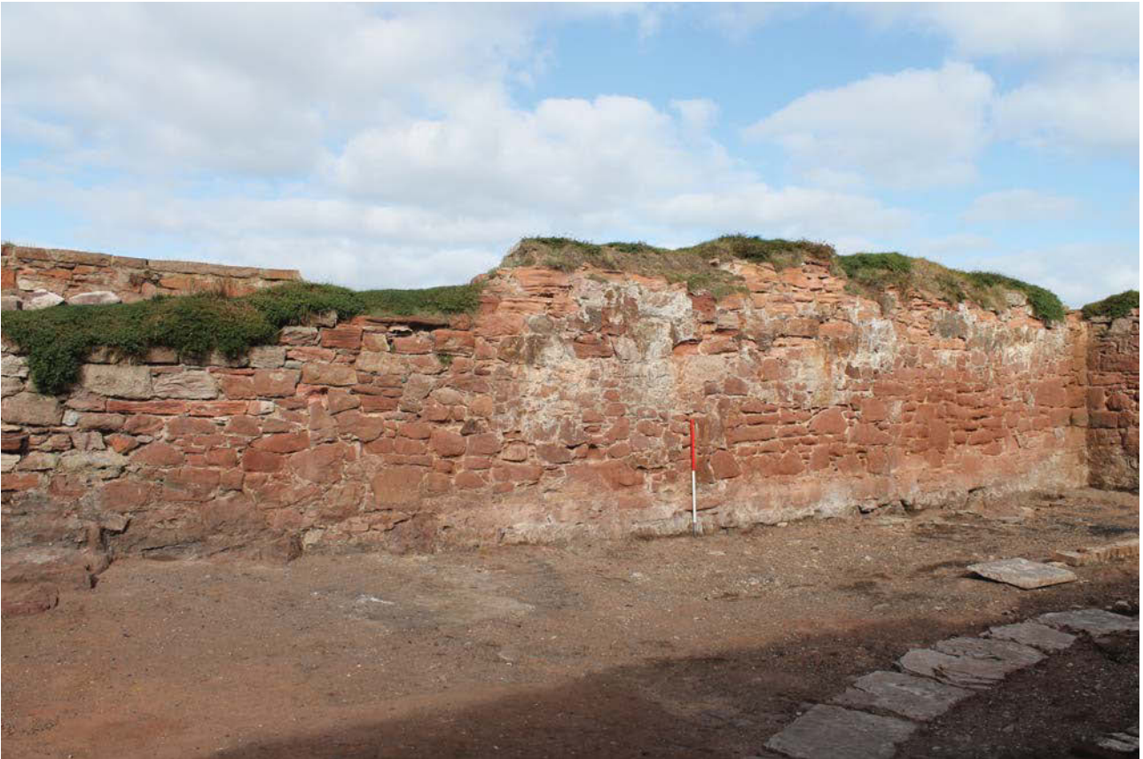
Plate 27: The Hospital building, north-west elevation from the south
