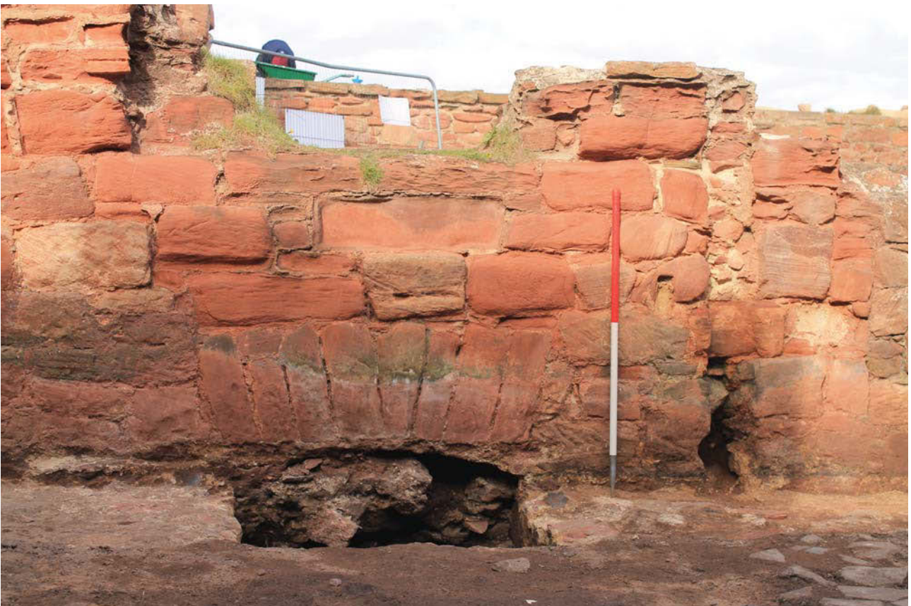
Plate 40: The Fumigation House, north-west elevation, detail of small drainage feature from the south-east
