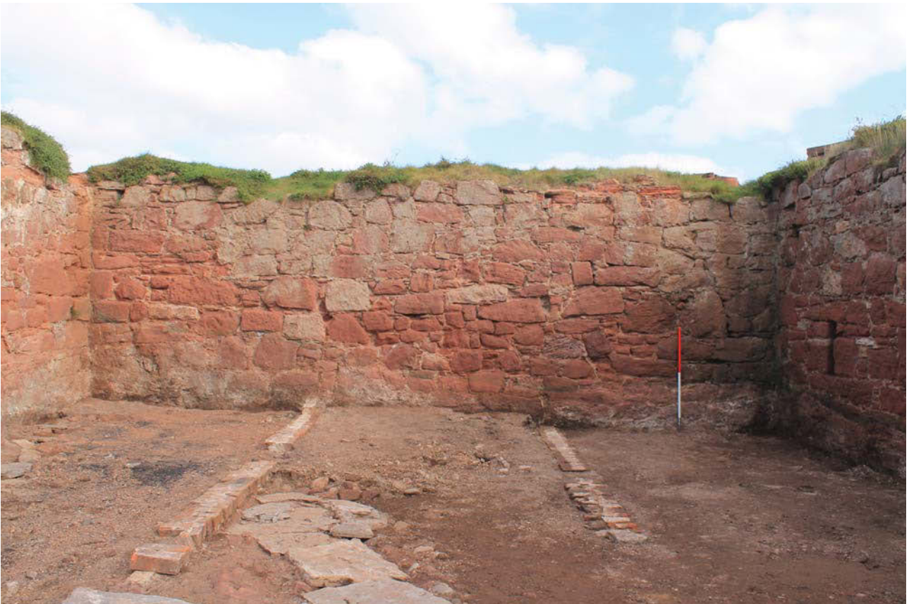
Plate 28: The Hospital building, north-east elevation, general view from the south-west
