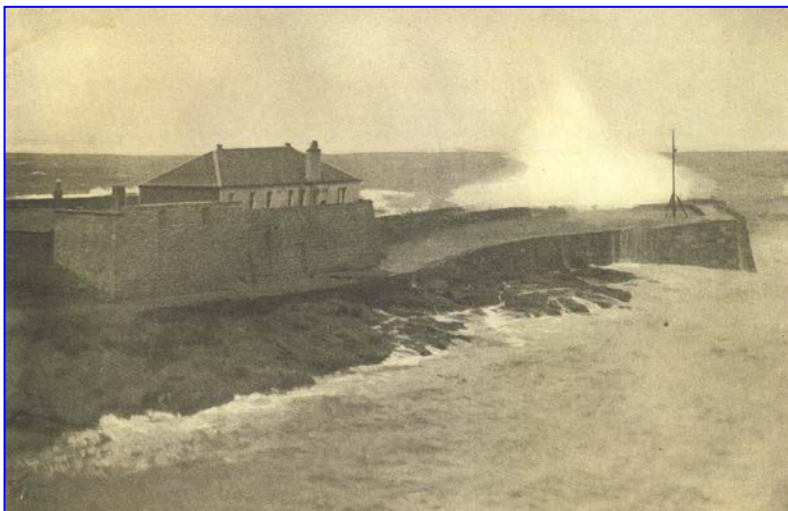
Figure 9b: Photograph of the 1872 hospital building from the south, 1914
