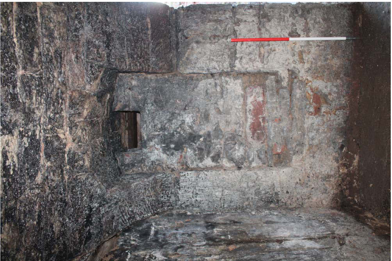
Plate 20: Vault 3, detail of the blocked doorway to the south-west side of the north-west wall from the south-east
