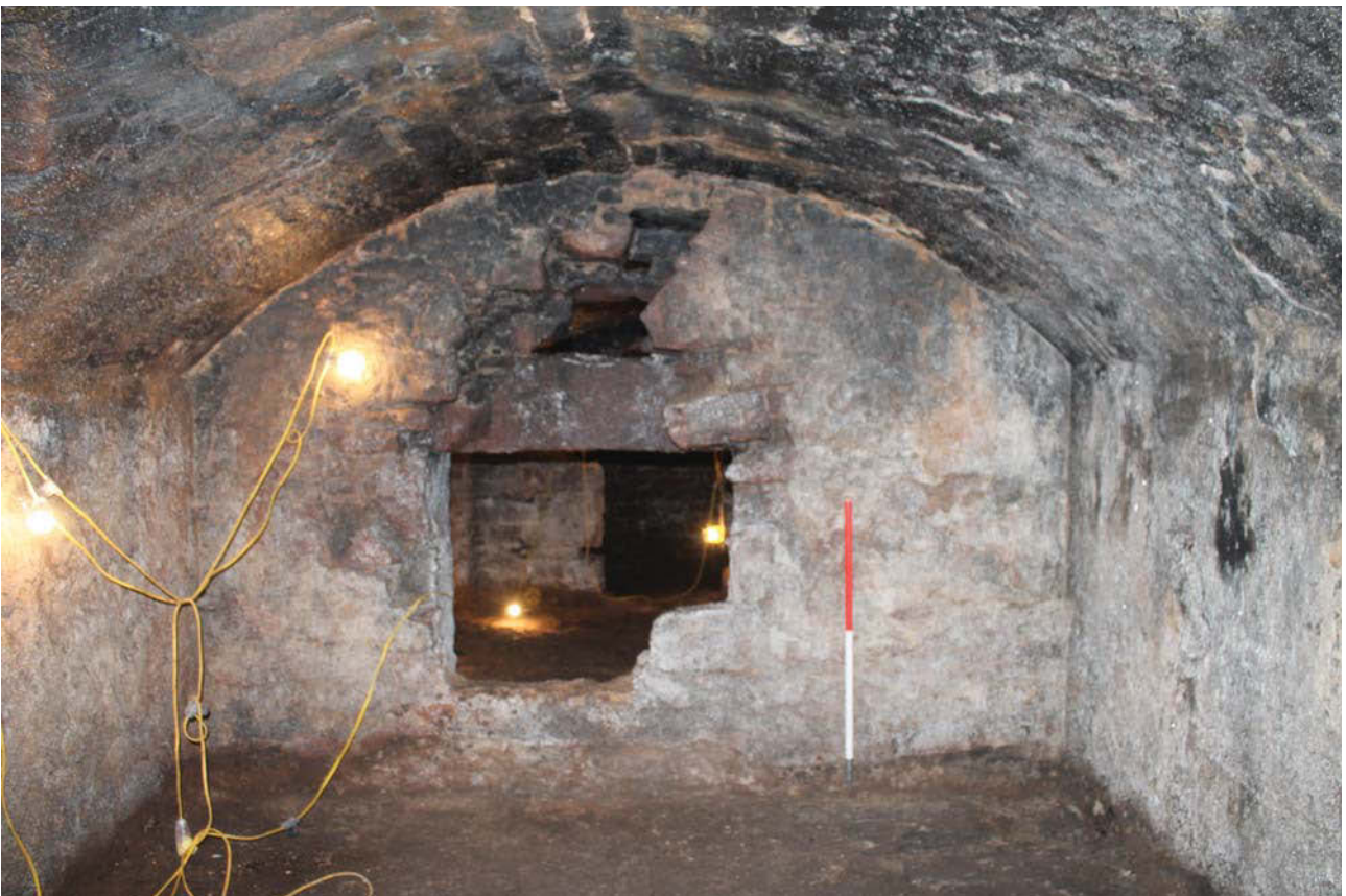
Plate 14: Vault 3, general view of the north-east wall showing the doorway to Vault 2, from the south-west
