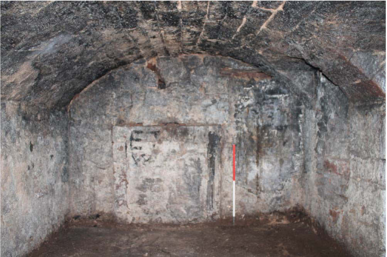
Plate 15: Vault 3, general view of the south-west wall from the north-east
