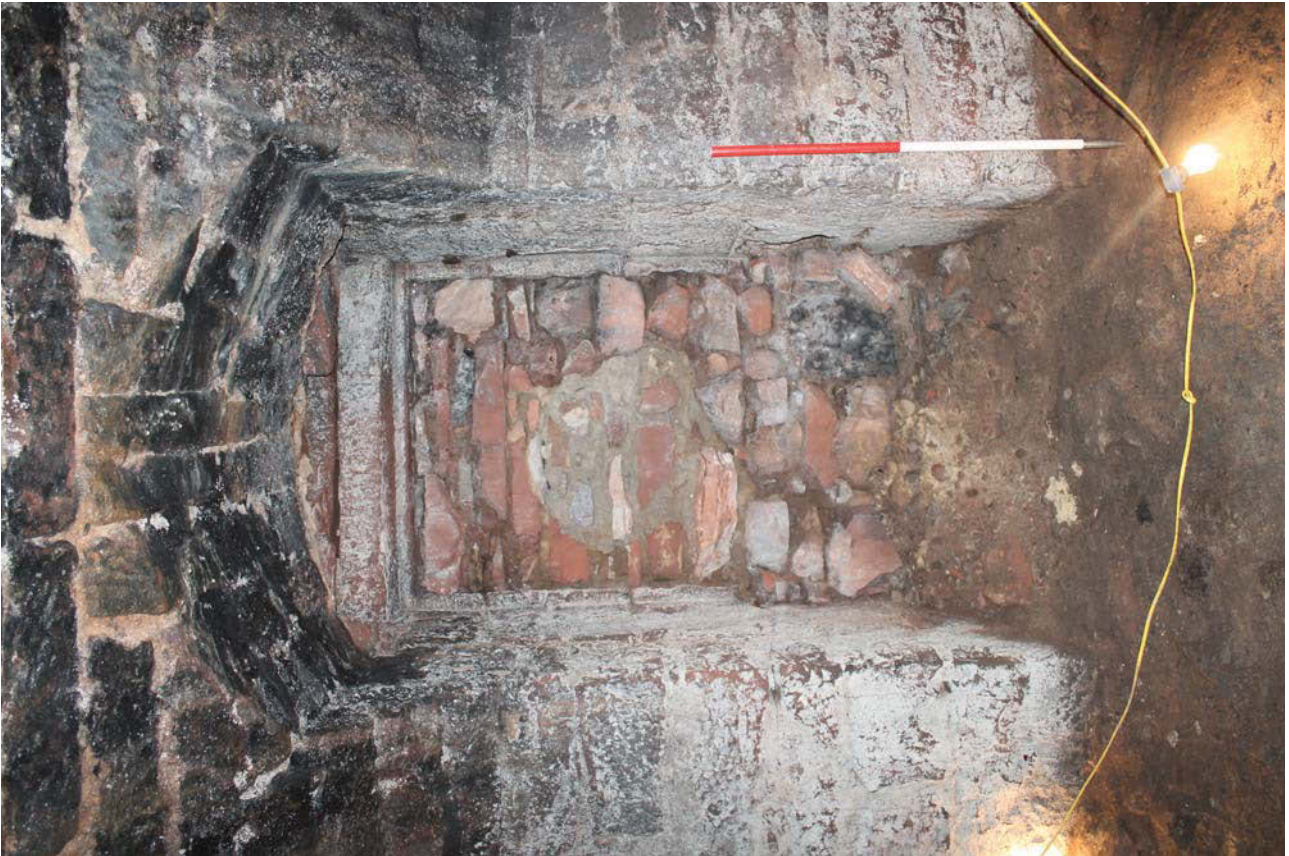
Plate 9: Vault 2, detail of the north-easternmost blocked doorway in the north-west wall, from the south-east
