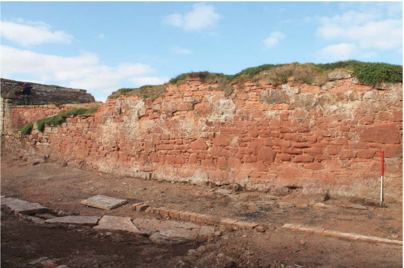
Plate 26: The Hospital building, north-west elevation, general view from the east
