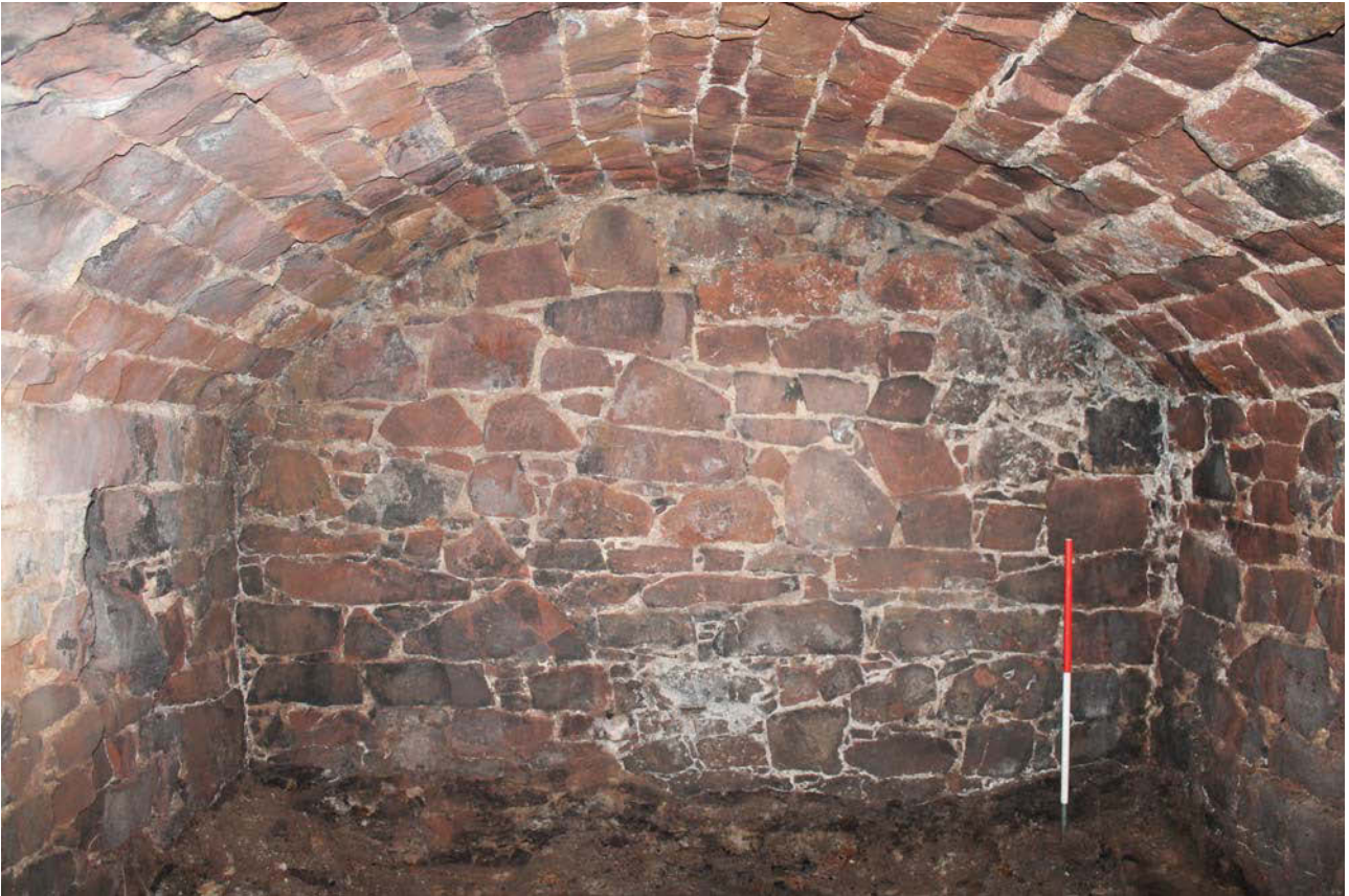
Plate 1: Vault 1, general view of the north-east wall from the south-west
