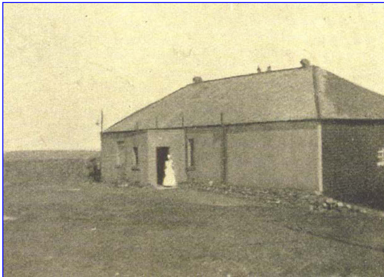
Figure 9a: Photograph of the 1872 hospital building from the west, showing the north-west elevation, 1914
