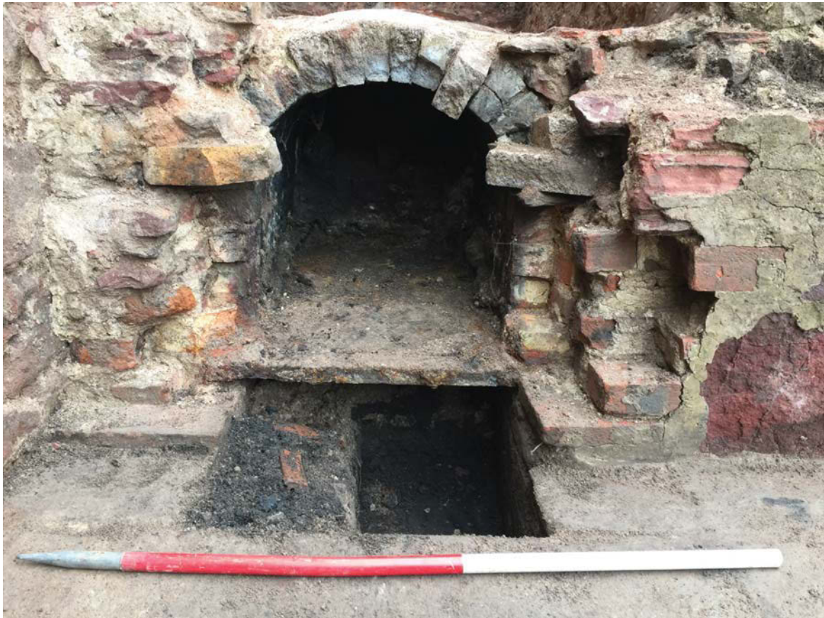
Plate 53: The Fumigation House, detail of the drain feature exposed after the excavation of the platform in the west corner, from the north-east
