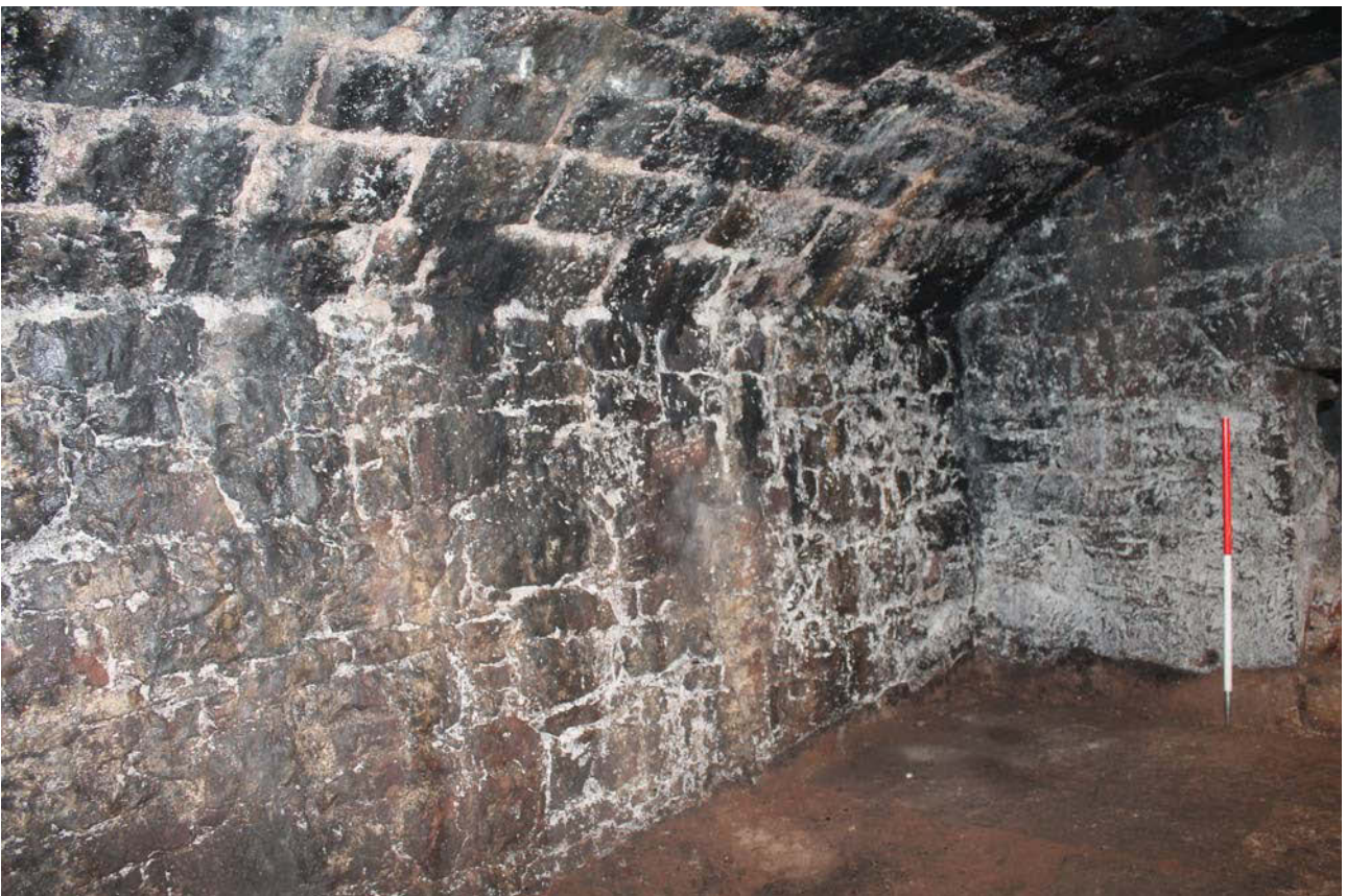
Plate 10: Vault 2, general view of the south-east wall from the north
