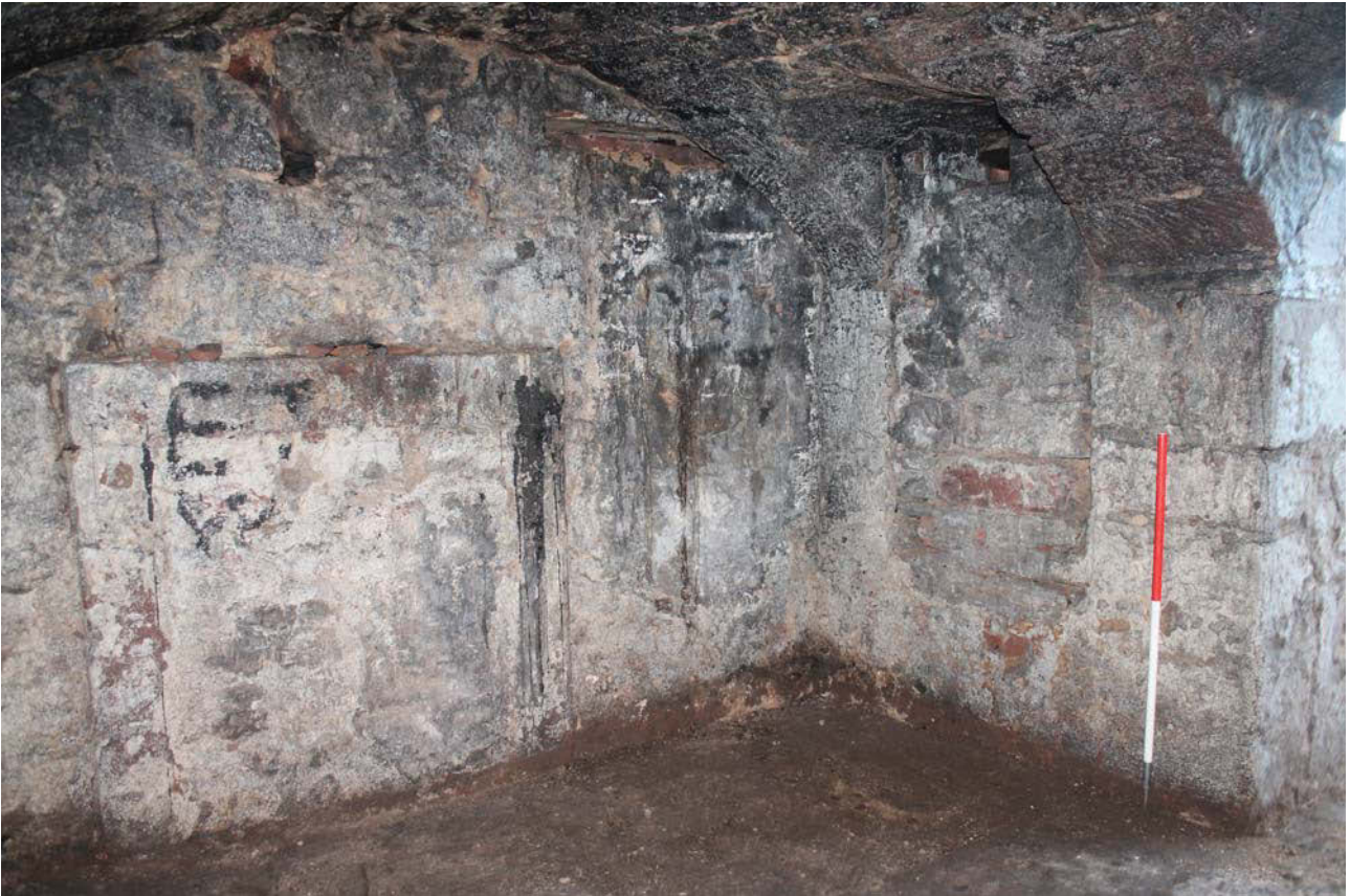
Plate 19: Vault 3, general view of the north corner from the south
