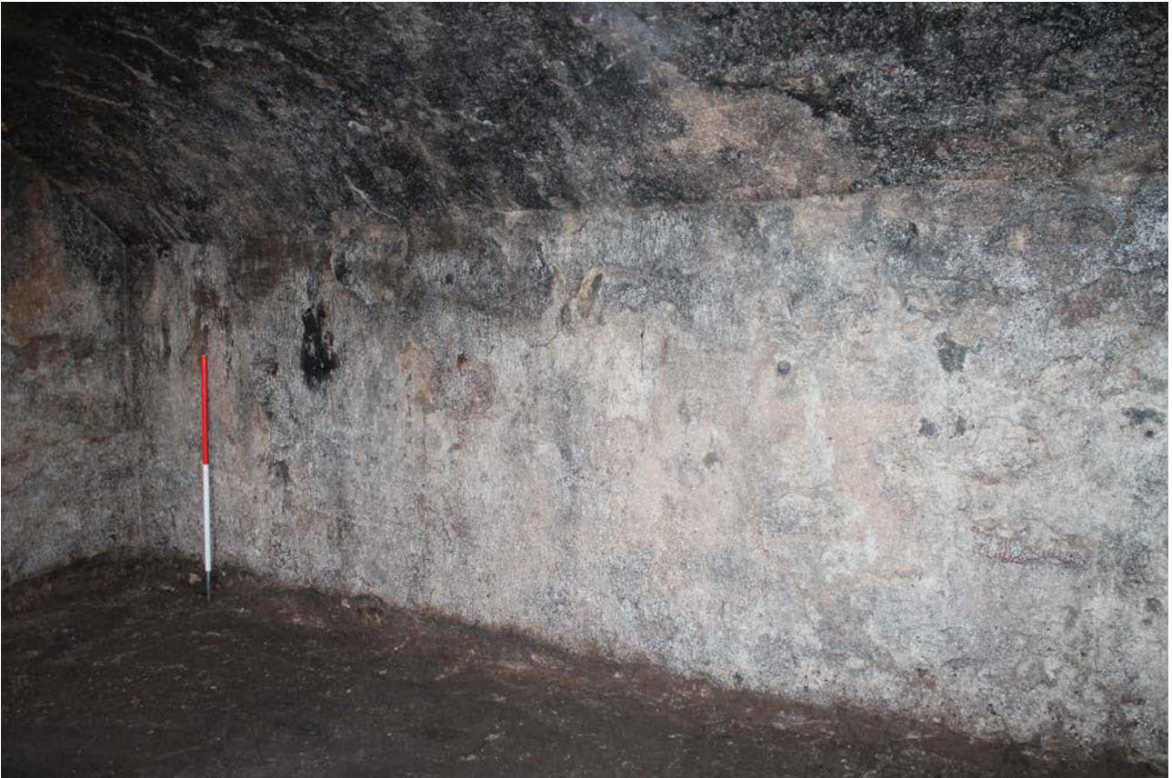
Plate 21: Vault 3, general view of the south-east wall from the north
