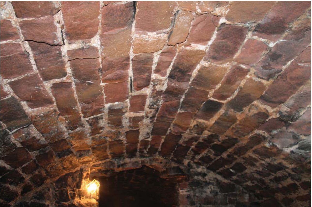
Plate 2: Vault 1, general view of the vaulted roof from the north-east
