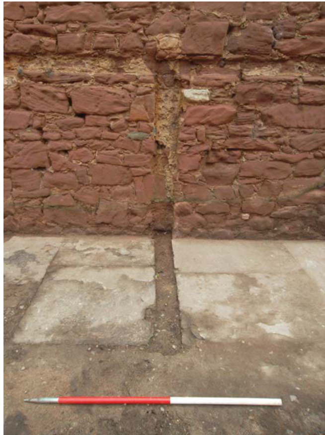
Plate 51: The Fumigation House, detail of linear recess [006]
