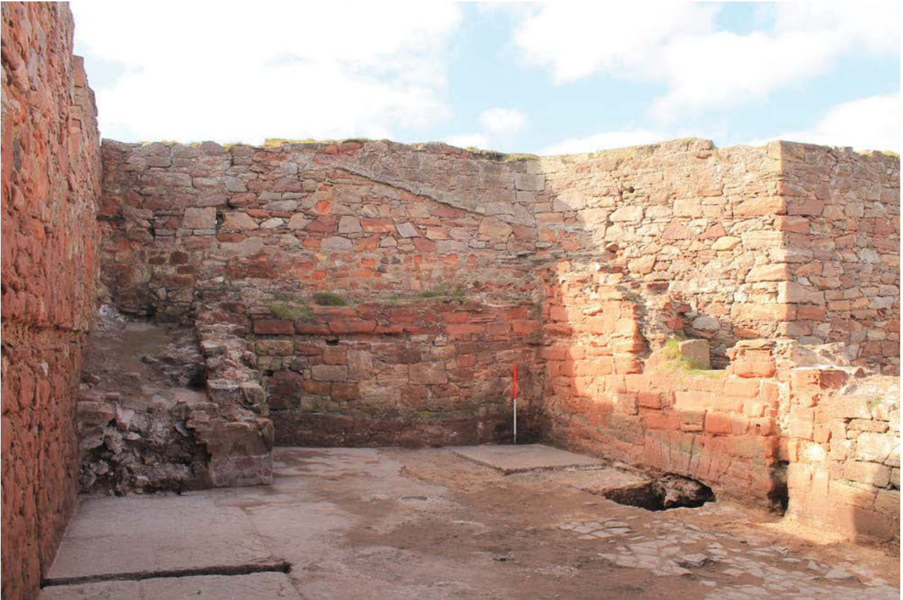
Plate 43: The Fumigation House, general view from the SEE
