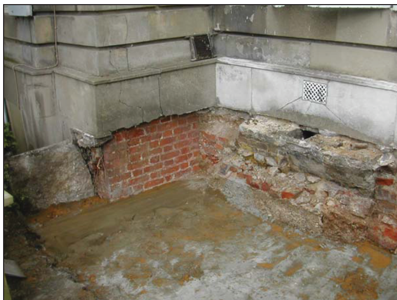
Plate 4: Concrete-filled lightwell, Trench 2
