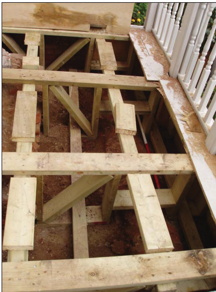
Plate 1: Early wall, obscured by current terrace platform.
