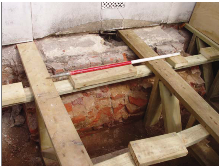
Plate 3: Remnant of Lightwell 1/004, Trench 1
