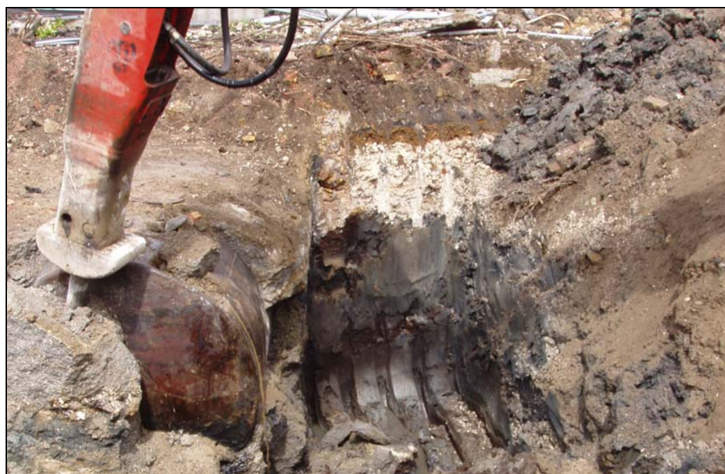
Plate 2: Removal of tanks, alluvial sequence in section behind.
