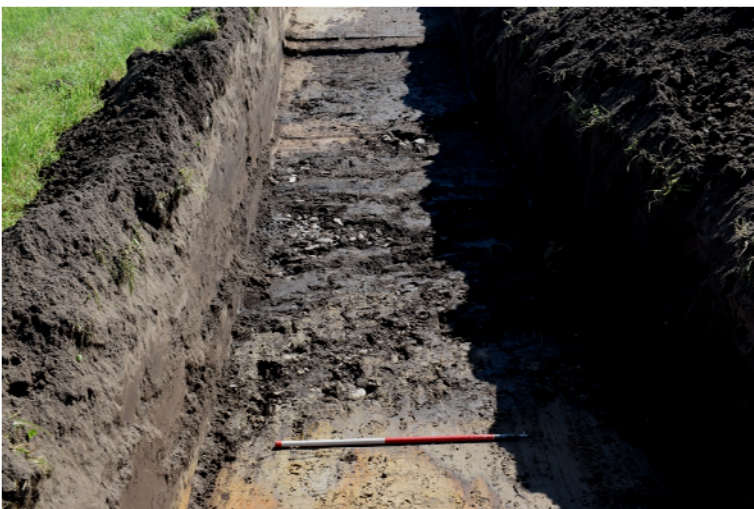
Plate 7: Looking southeast over drainage ditch [101/301]
