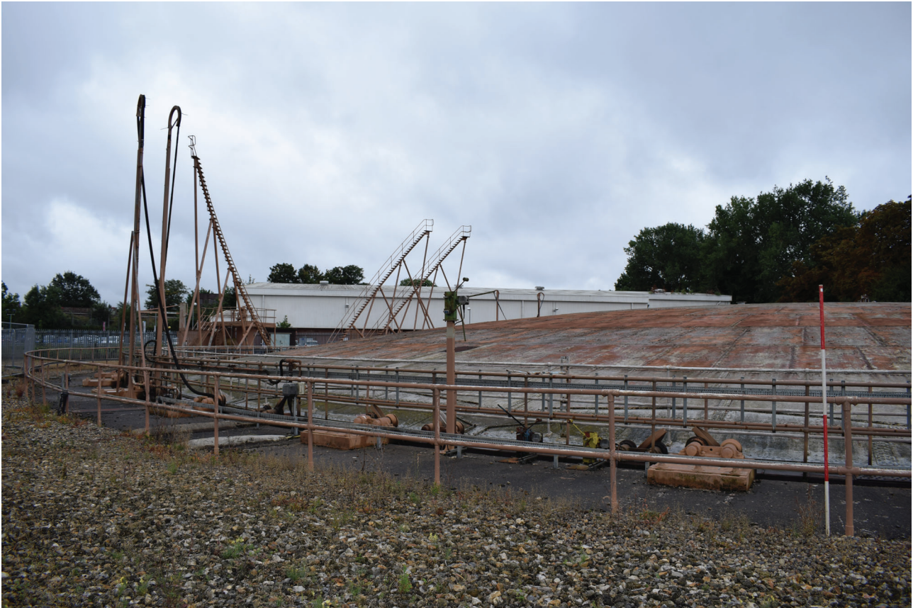
Plate 31: Gasholder No 4, general view of the north-east side of the gasholder from the NNW
