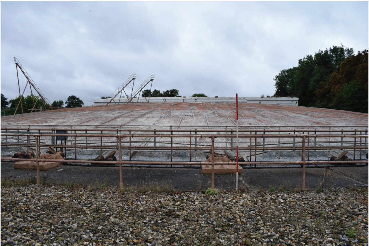
Plate 28: Gasholder No 4, general view from the north
