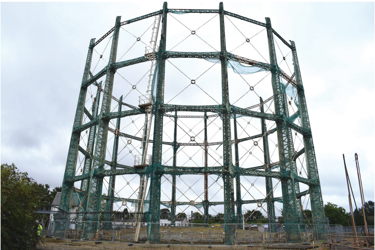
Plate 2: Gasholder No 5, general view from the north-west
