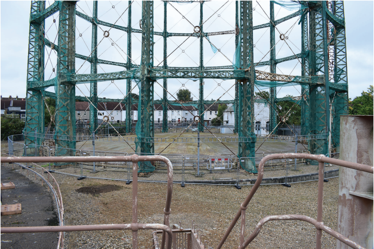
Plate 1: Gasholder No 5, general view from the south-west
