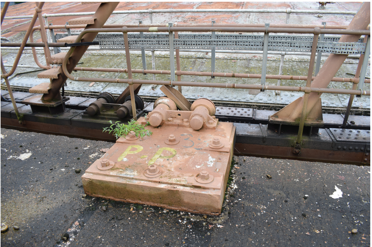
Plate 34: Gasholder No 4, detail of outer roller carriage from the south-east
