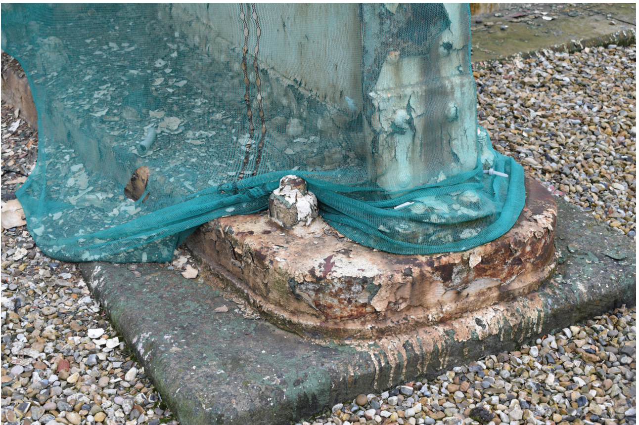
Plate 4: Gasholder No 5, detail of the guided frame footing from the north-west
