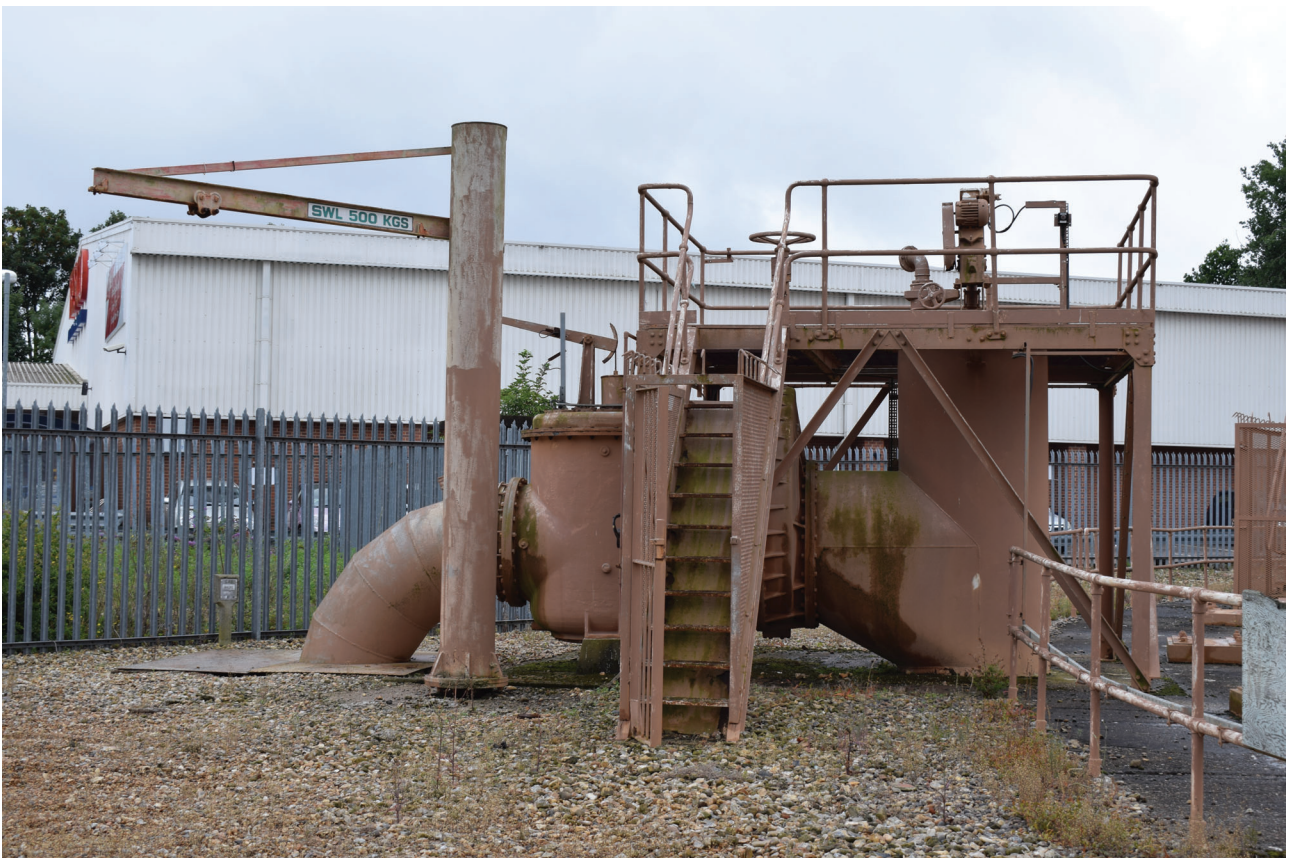
Plate 52: General view of pipe and gantry structure to the south of the gasholder complex, from the north
