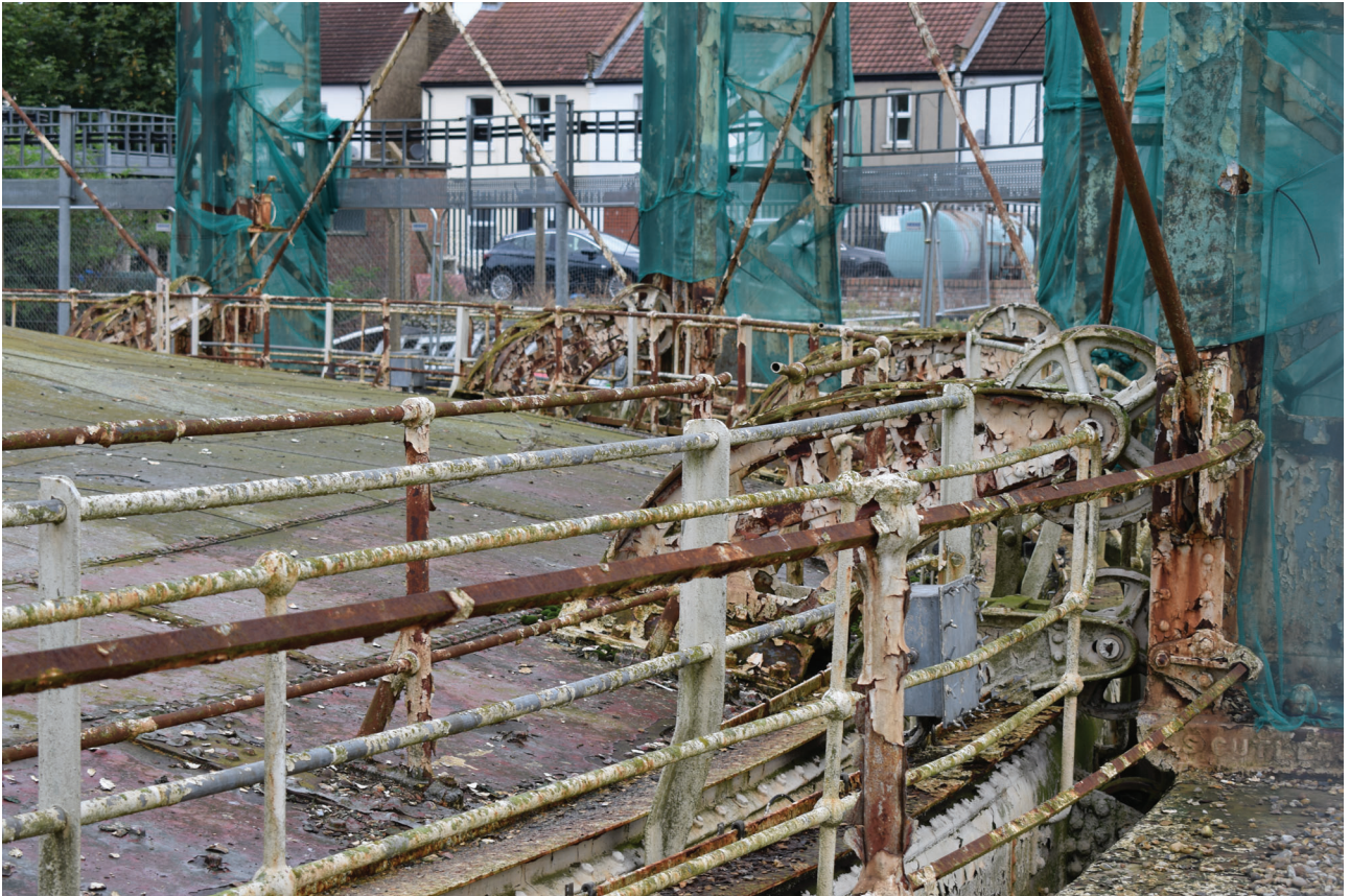
Plate 5: Gasholder No 5, detail of the guided rollers from the south
