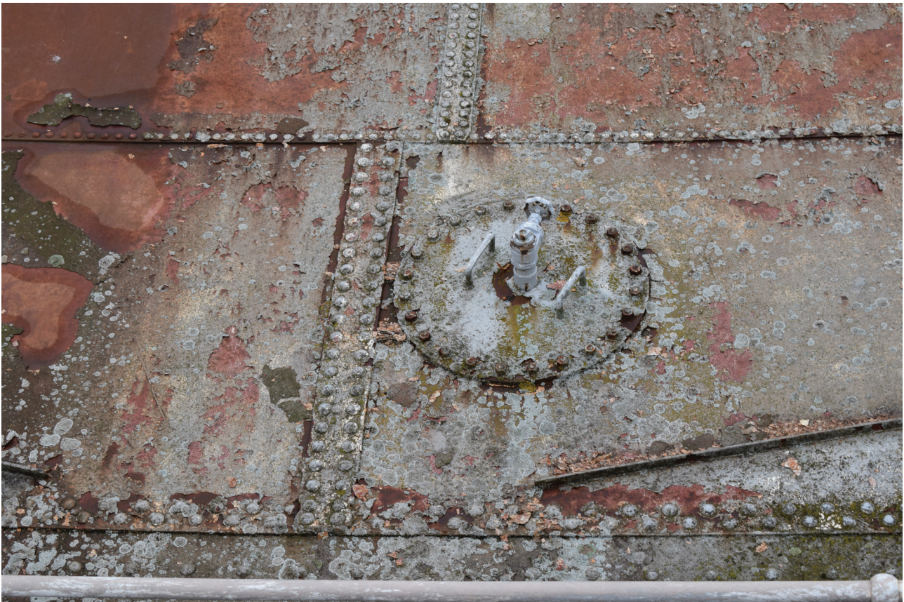
Plate 30: Gasholder No 4, detail of rounded riveted panel on the crown of the gasholder from the south-east
