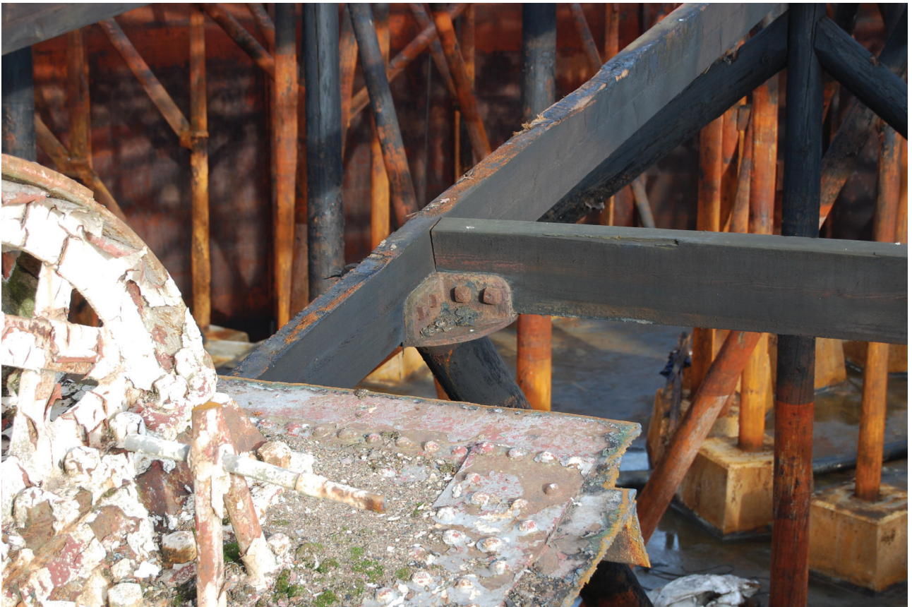
Plate 26: Gasholder No 5, close detail of the exposed timber crown framing, from the SSE
