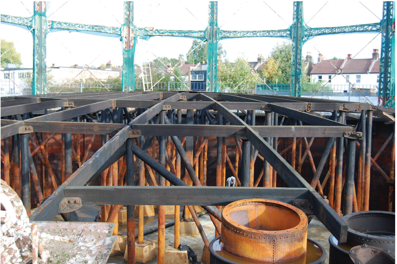
Plate 24: Gasholder No 5, close detail of the exposed timber crown framing, from the south
