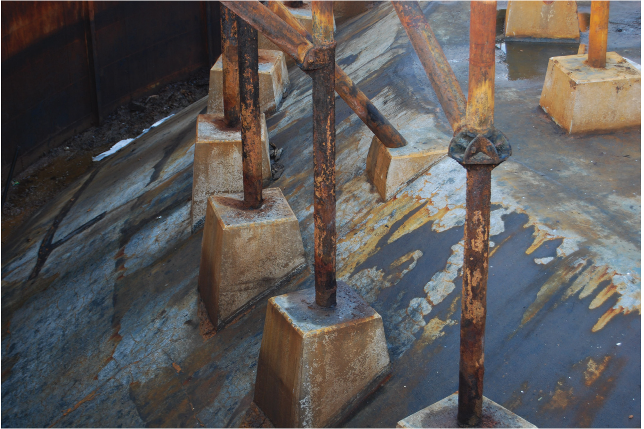
Plate 17: Gasholder No 5, close detail of the dumping and crown framing support, from the SSE
