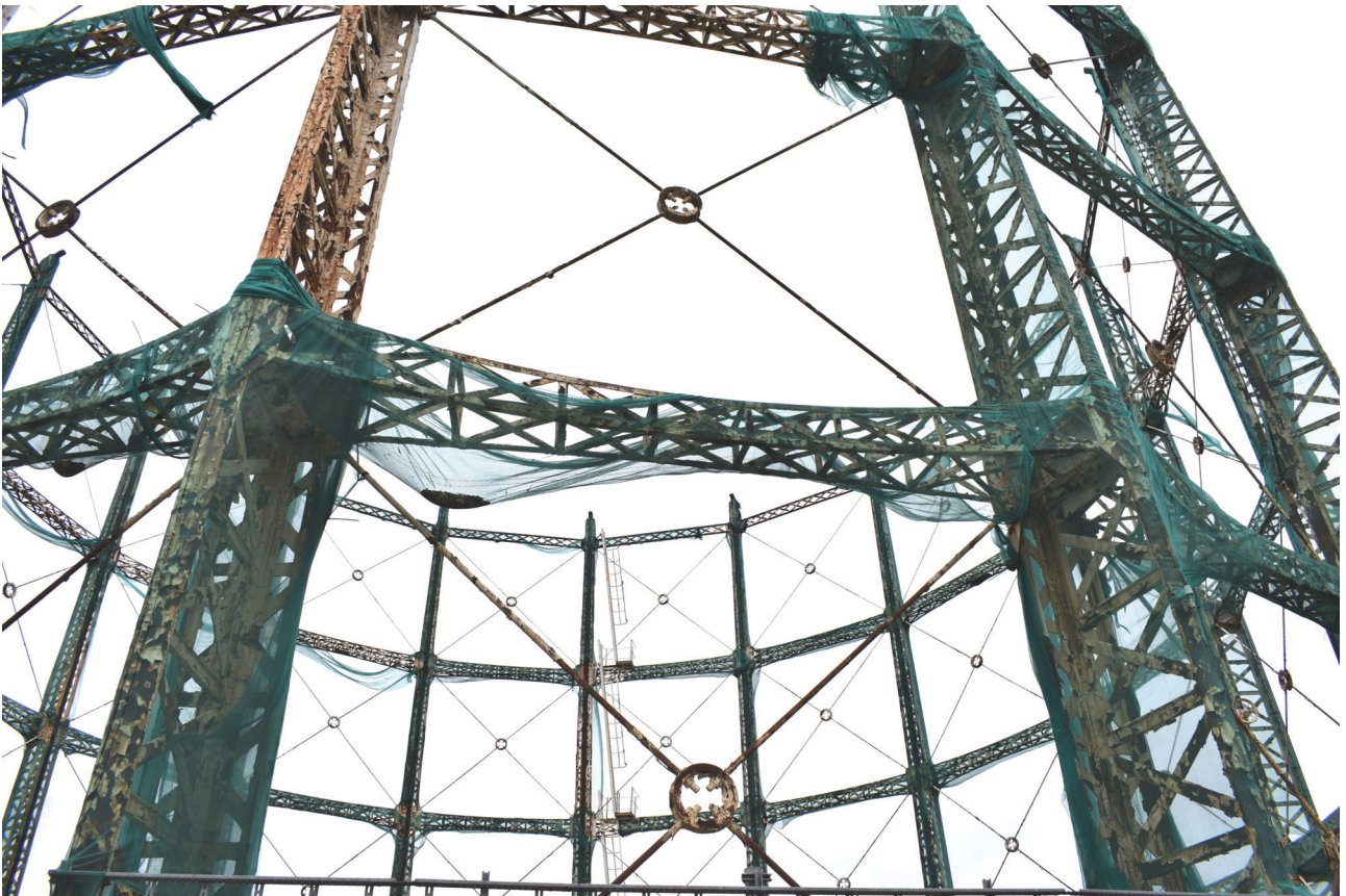
Plate 3: Gasholder No 5, detail of the guided frame from the south
