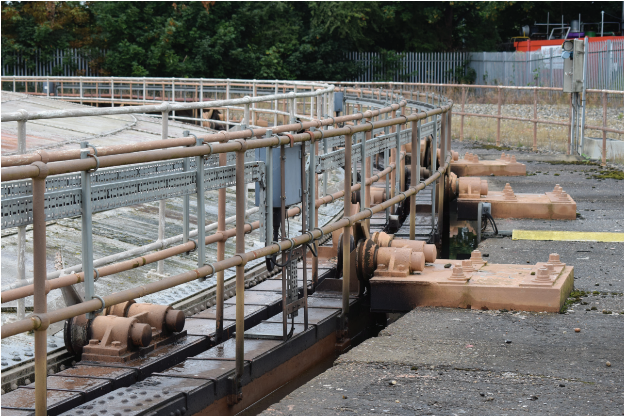
Plate 33: Gasholder No 4, detail of the roller carriages on the north-east side of the gasholder from the east
