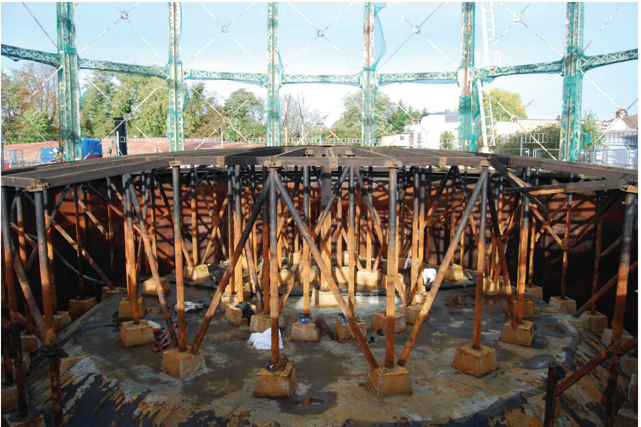
Plate 23: Gasholder No 5, close detail of the exposed timber crown framing, from the south
