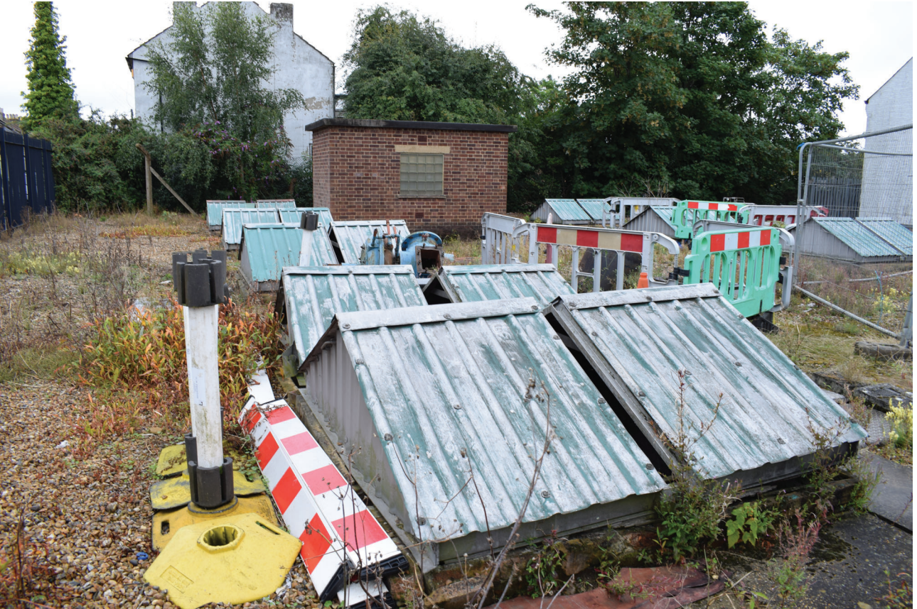
Plate 49: Building C, general view of timber covers for pipework with Building B in the background, from the north-west
