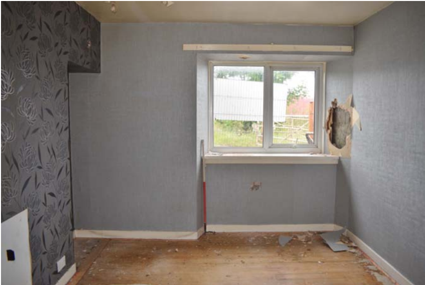
Plate 10: Image of northwest interior wall and window of room 3, A2
