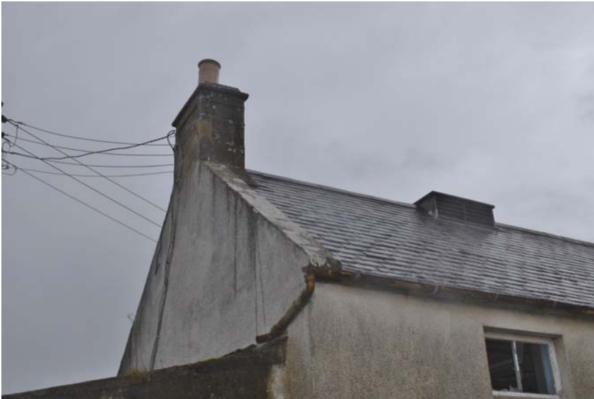
Plate 4: Image of chimney in north east gable of A1
