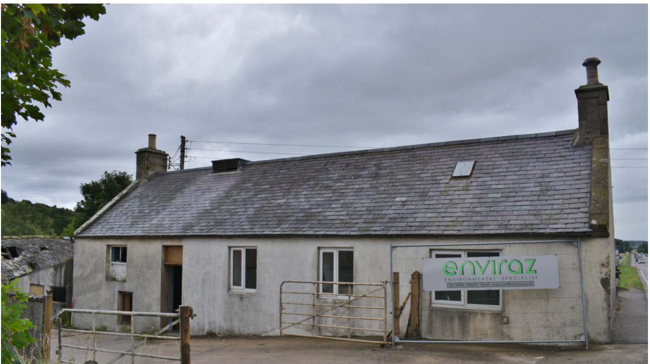
Plate 3: Oblique image of northwest elevation of D (left), A1 (centre) and A2 (right)
