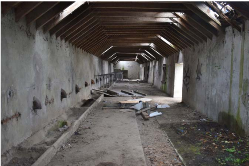
Plate 24: Image of northwest interior gable end of steading B2
