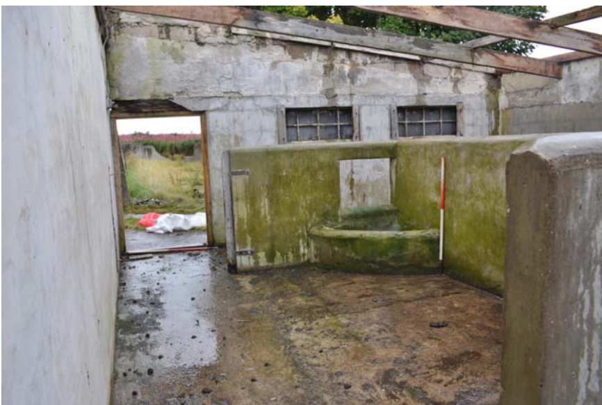
Plate 27: Image of northwest interior wall of B3 and stalls
