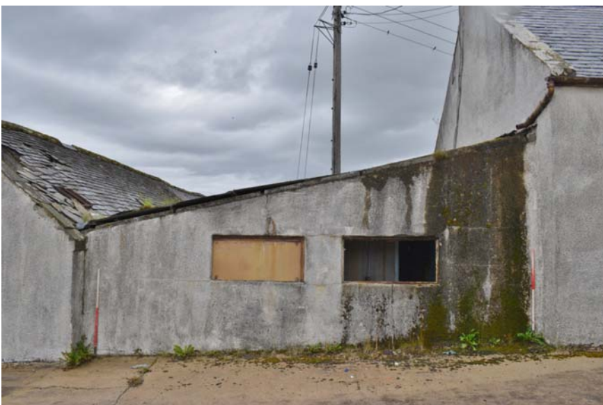
Plate 29: Image of northwest exterior wall of building (B2 left, A1 right)
