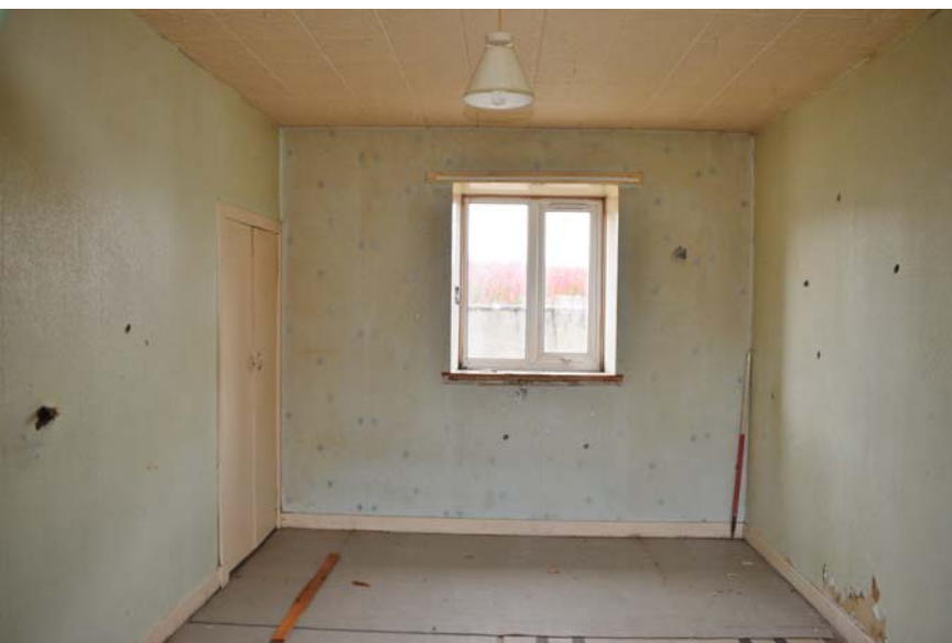
Plate 14: Image of northwest interior wall and window of room 3, A2
