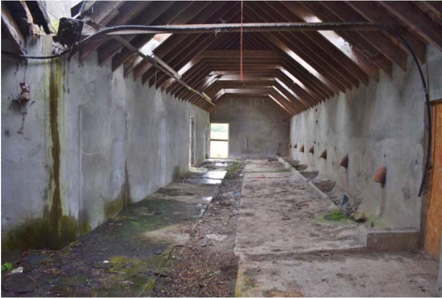
Plate 25: Image of northeast interior gable end of steading B2
