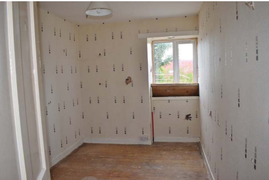
Plate 13: Image of northwest interior wall and window of room 2, A2
