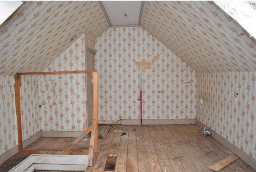
Plate 12: Image of southwest interior wall of attic, A2
