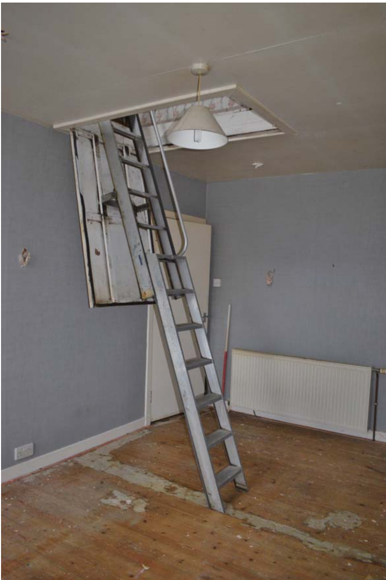
Plate 11: Image of northeast and southeast interior wall corner and attic access of room 3, A2
