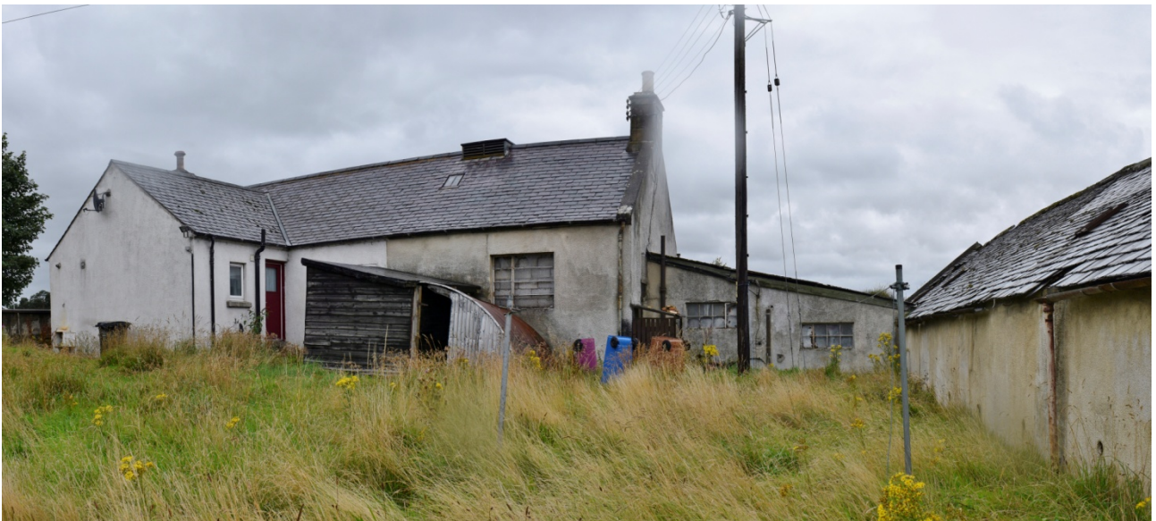
Plate 5: Image looking west southwest across house A (left) and steading B (right)
