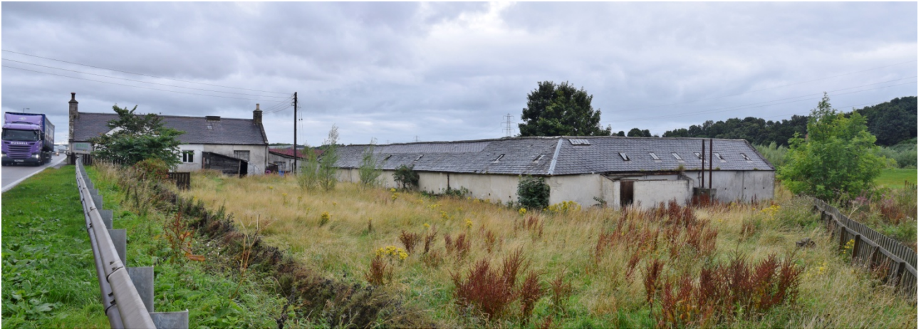
Plate 1: Image looking northwest across development site, house A (left) and steading B (right)
