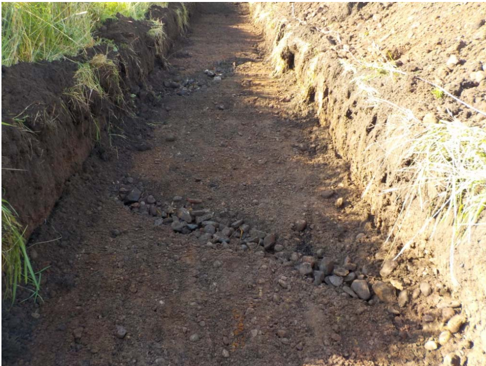
Plate 2: General view of rubble drains in Trench 8
