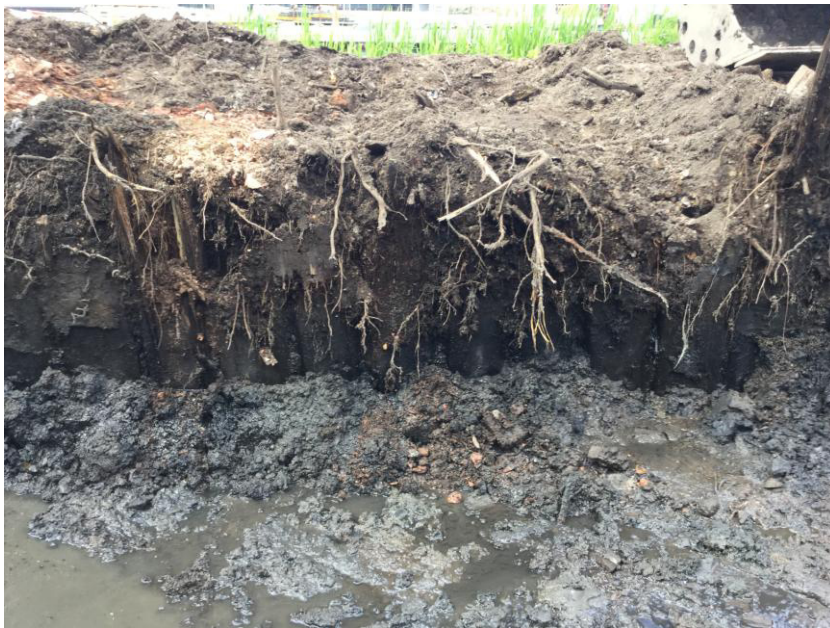
Plate 6 - W/centre of canal lining (007)
