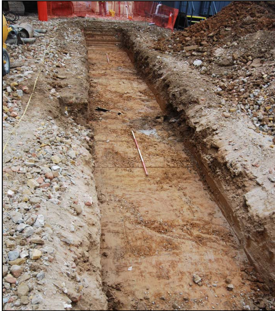
Plate 3: Trench 2 Overview Looking Northeast
