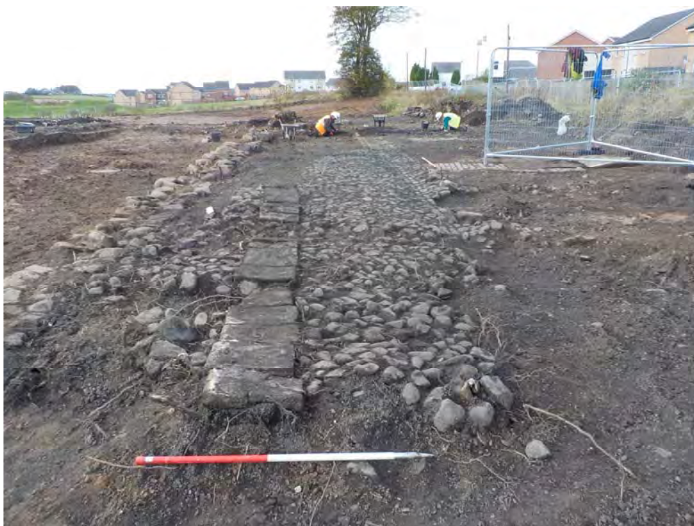
Plate 7: General view of cobbles [048] and modern drain base [049]
