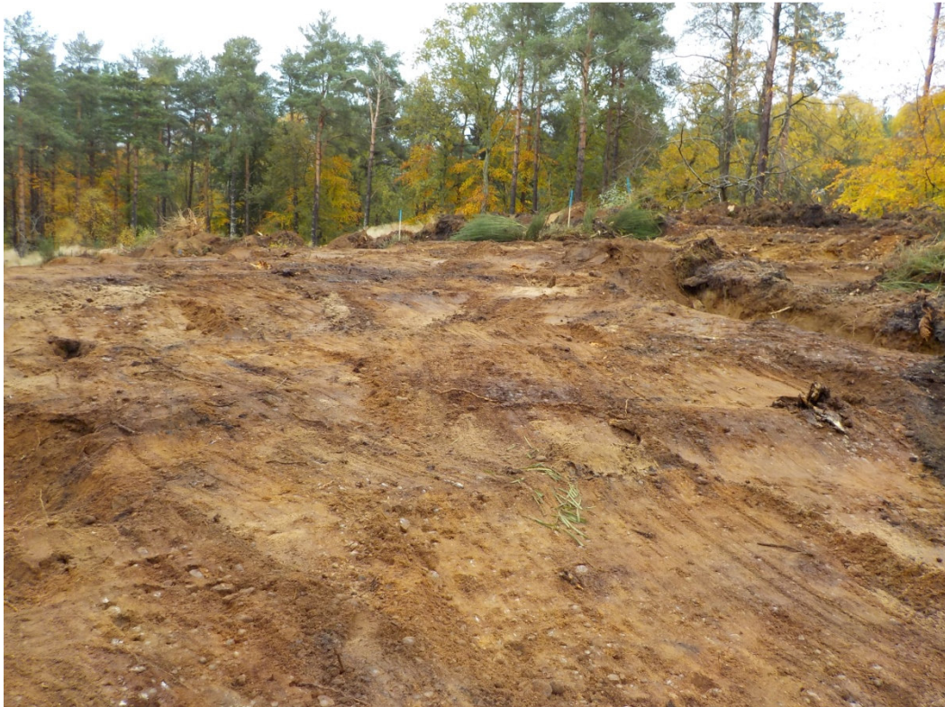
Plate 4 View of stripped area
