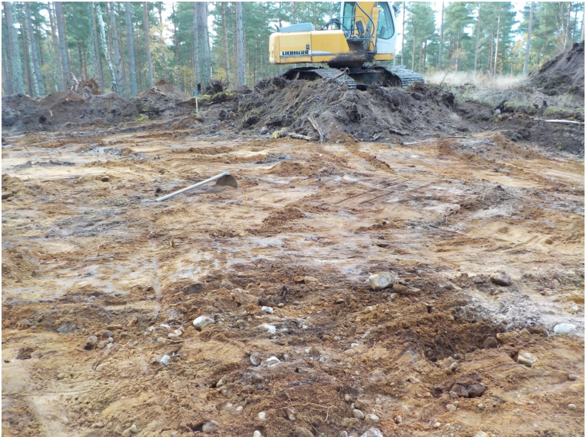
Plate 4 View of stripped area
