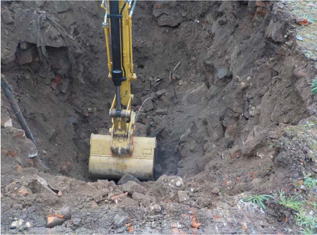
Plate 1: General view of Trench 4 excavations to 4m
