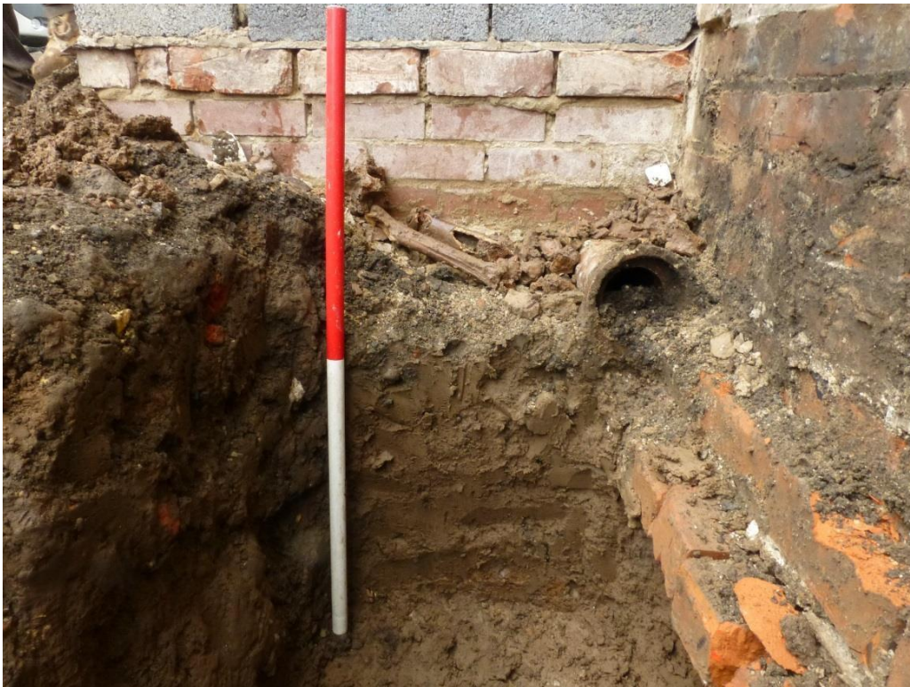
Plate 2: East facing view of context (1003) and foundations for (1002) and (1005)
