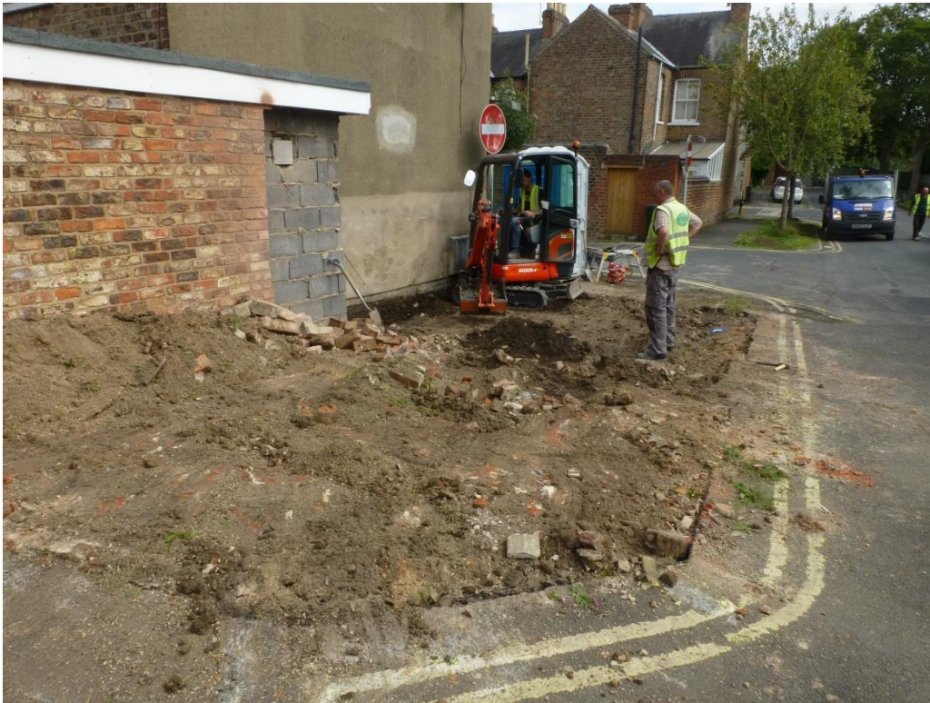
Plate 1: NE facing view of the development site during stripping
