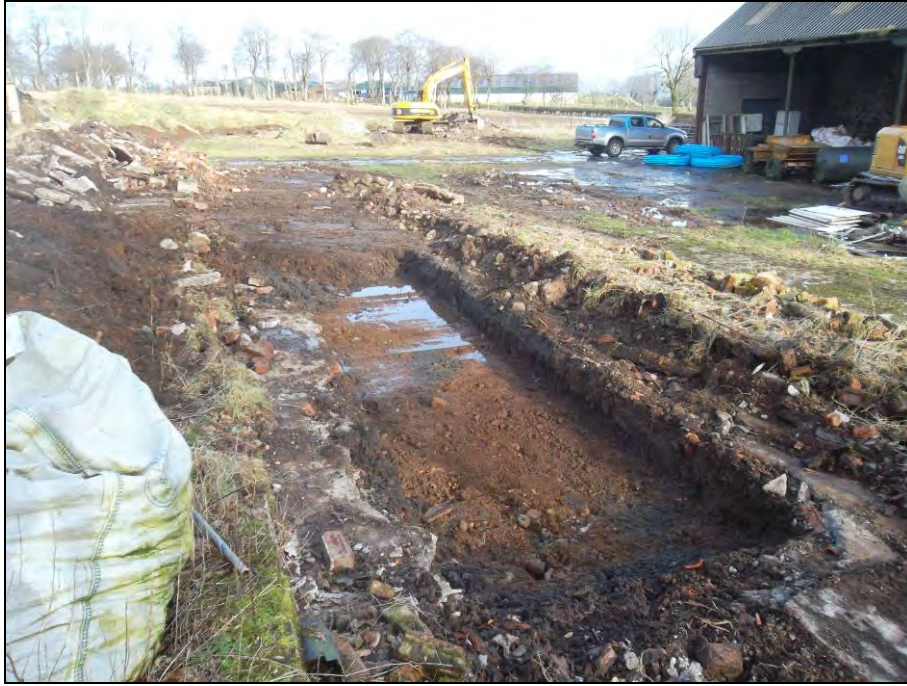
Plate 3: Trench 3 post excavation & partially backfilled to prevent flooding, from southwest
