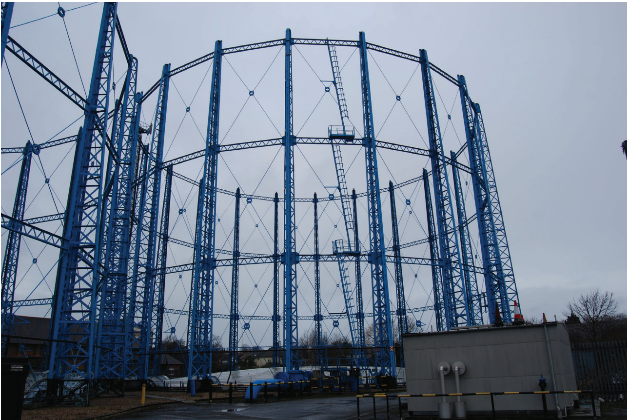
Plate 29: Bell Green, Sydenham, Gasholder No 8, general view of the gasholder frame from the SSE
