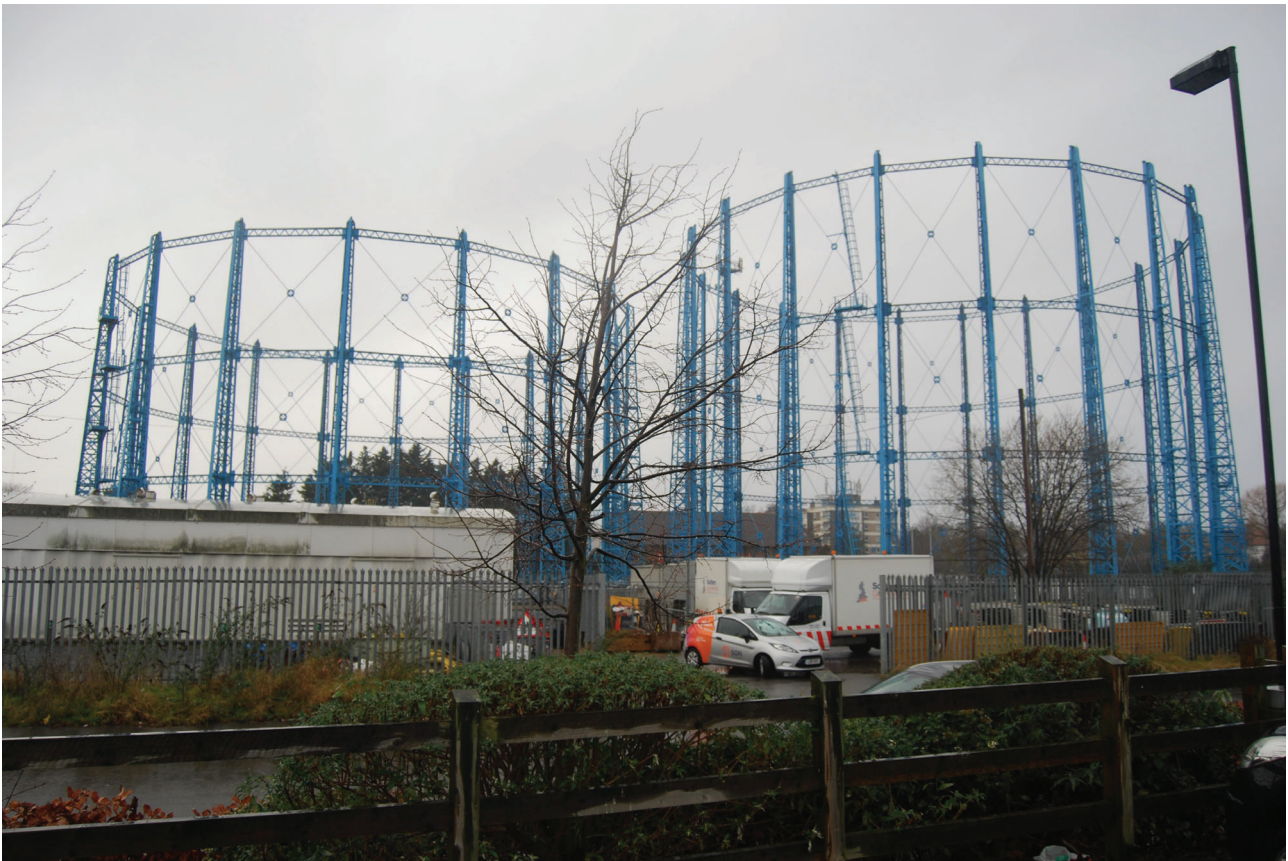
Plate 1: Bell Green, Sydenham, Gasholders No 7 & 8, general view from the south-east
