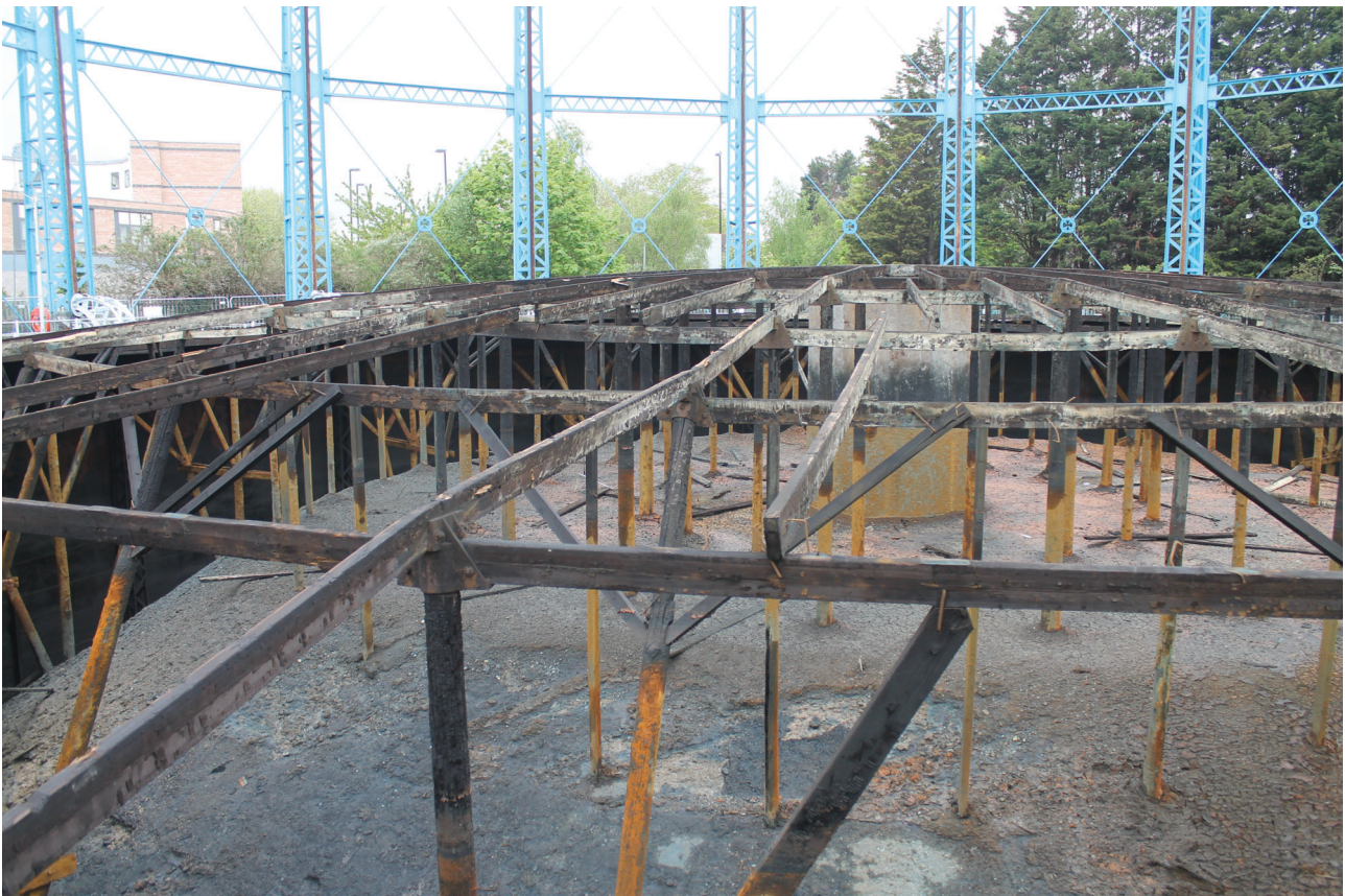
Plate 24: Bell Green, Sydenham, Gasholder No 7, general view of the dumping and support frame, from the east
