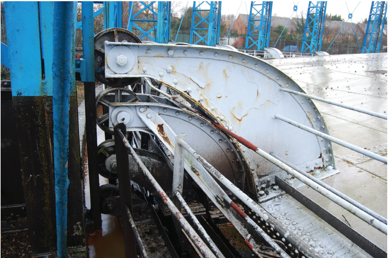
Plate 38: Bell Green, Sydenham, Gasholder No 8, detail of the guided rollers behind No 7 standard from the SSW
