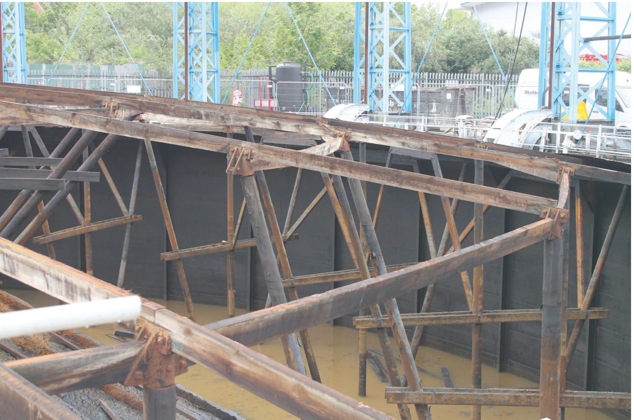
Plate 46: Bell Green, Sydenham, Gasholder No 8, general view of the outer ring of upright and leaning posts with metal bracket holding them together, from the south-west
