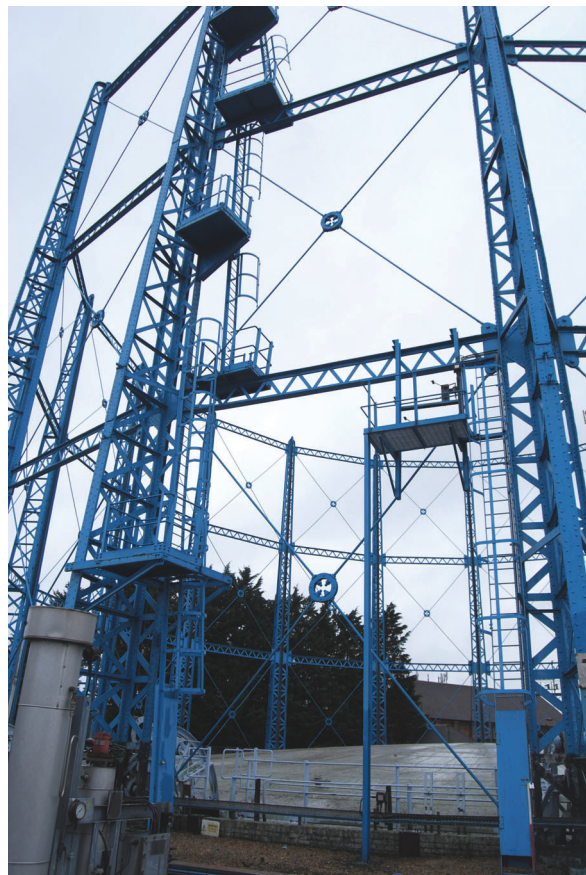
Plate 20: Bell Green, Sydenham, Gasholder No 7, general view looking up at access ladders and gantries between No 3 and No 4 standards from the SSE
