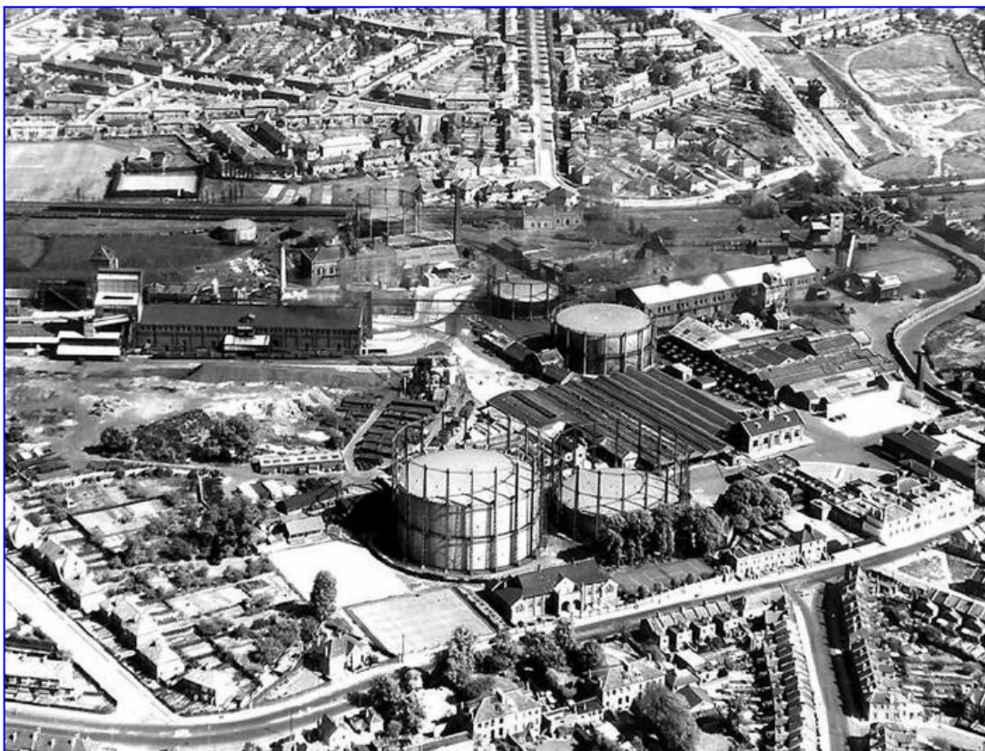
Figure 10: Undated aerial photograph of the Bell Green Gasworks, ca. mid-20 th century © National Gas Archive Gasholders No 7 and 8 can be seen in the foreground behind the 1911 Livesey Hall, with Gasholders No 4 and 5 in the background behind the purifiers. The large building to the centre-left of the photograph is one of the retort houses
