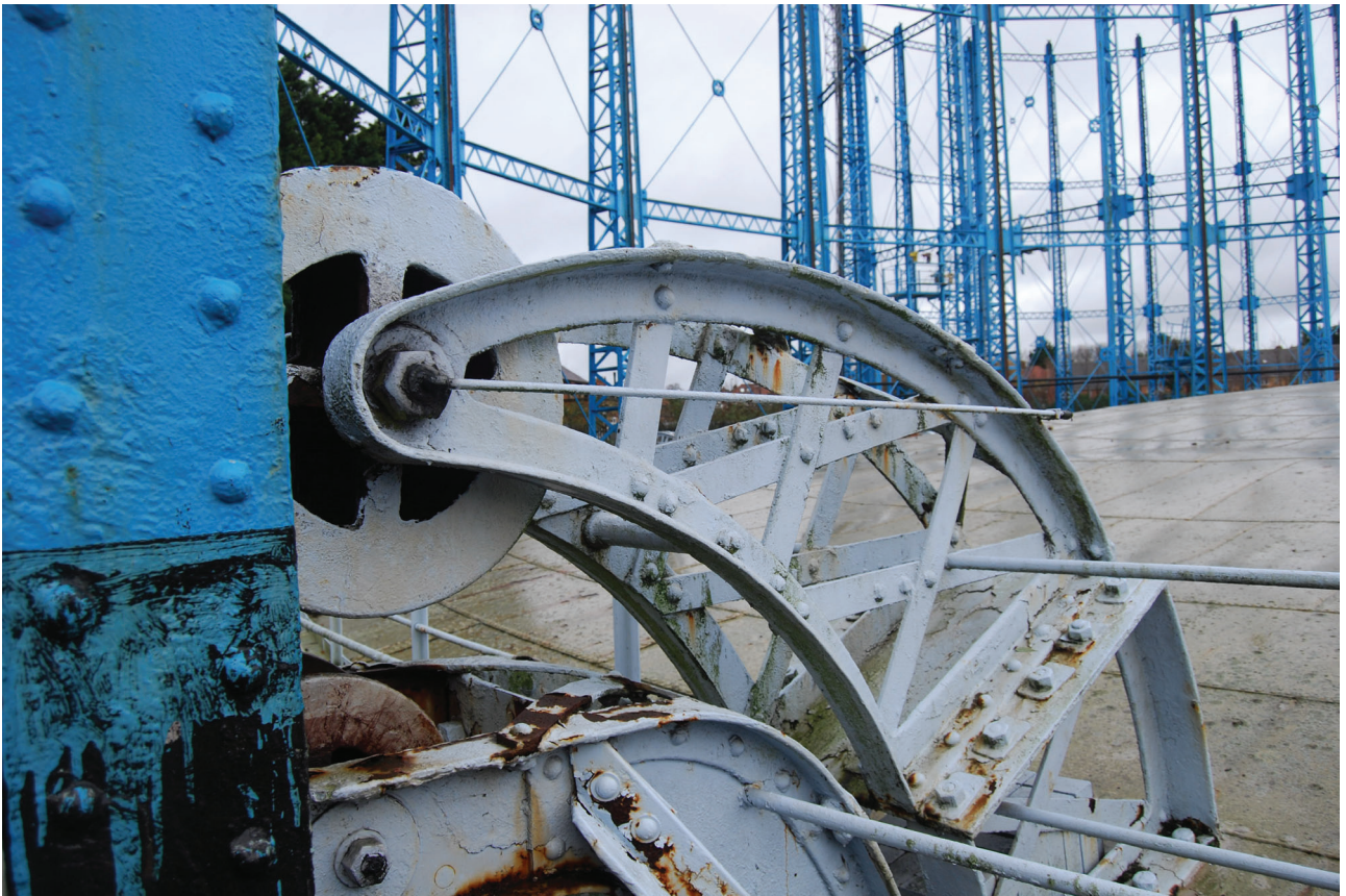
Plate 16: Bell Green, Sydenham, Gasholder No 7, detail of the guided rollers behind No 7 standard from the SSE
