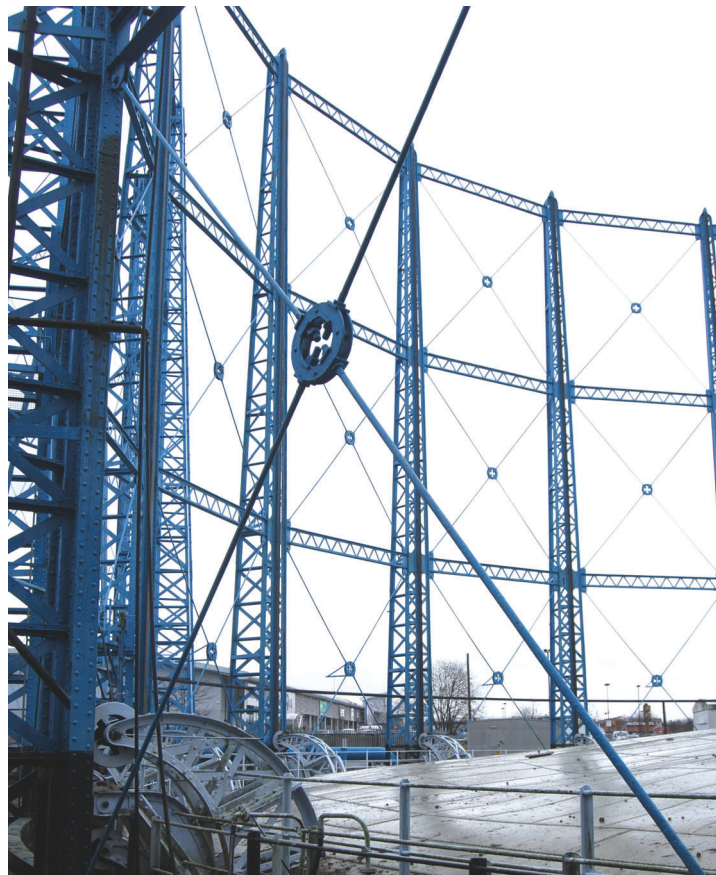
Plate 8: Bell Green, Sydenham, Gasholder No 7, detail of the diagonal bracing between the standards from the west
