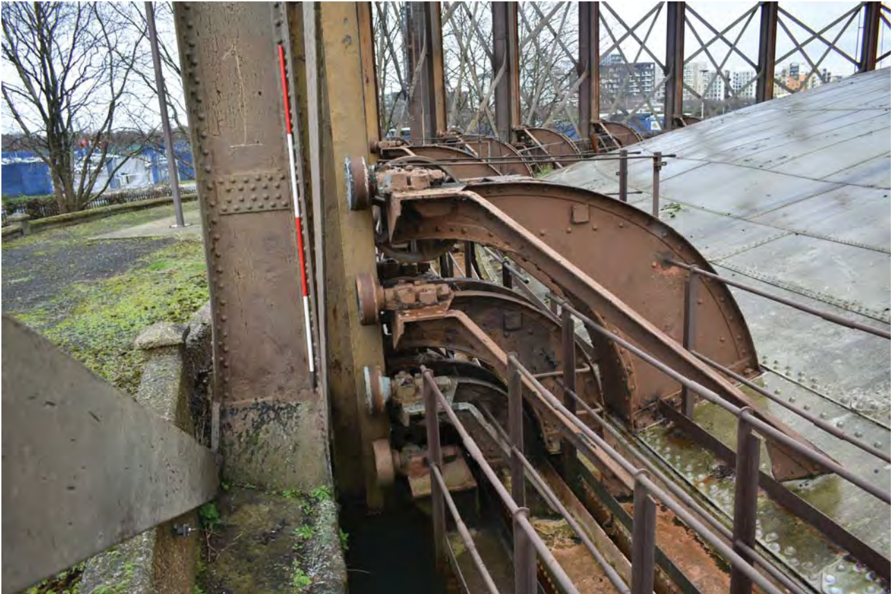
Plate 15: Gasholder No 1, detail of the guided rollers behind No 1 standard, from the WNW
