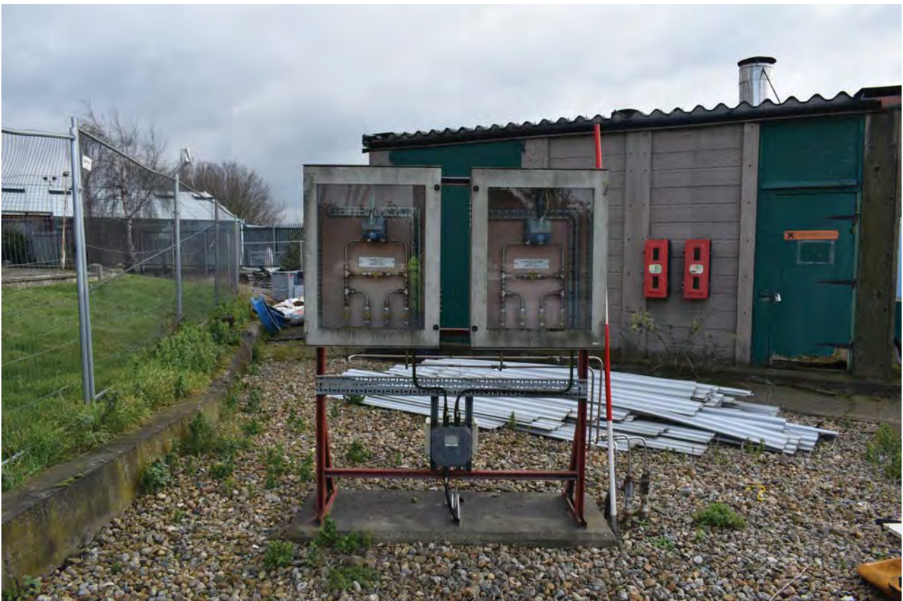
Plate 48: Hi (Holder Outlet Valve) and Hii (Volumetric Governor Overflow), general view from the NNW
