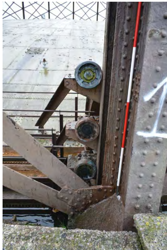
Plate 16: Gasholder No 1, detail of the guided rollers behind No 1 standard, from the NNW
