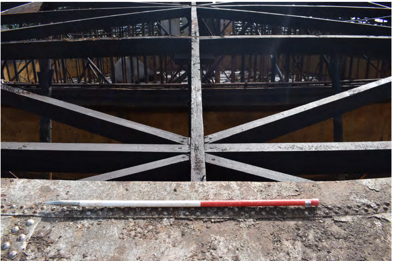
Plate 26: Gasholder No 1, detail of nailed joint, from the WSW
