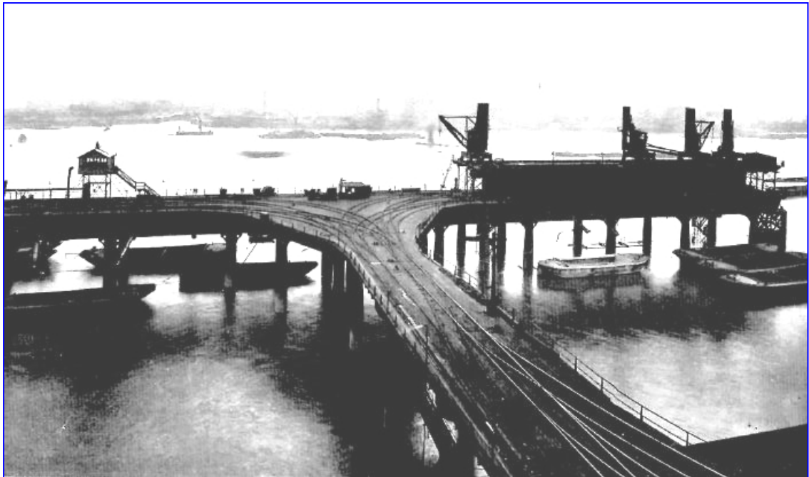
Figure 11: Archive photograph of the jetty from which coal would have been brought into the Blackwall Lane Gasworks, 1925, after Carpenter 1925, Figure 2 © National Gas Archive
