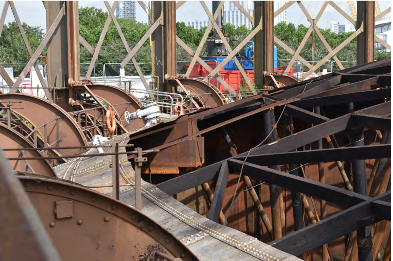
Plate 41: Gasholder No 1, general view of the outlet pipe with Livesey man-lid on the WSW of the gasholder, from the SSW
