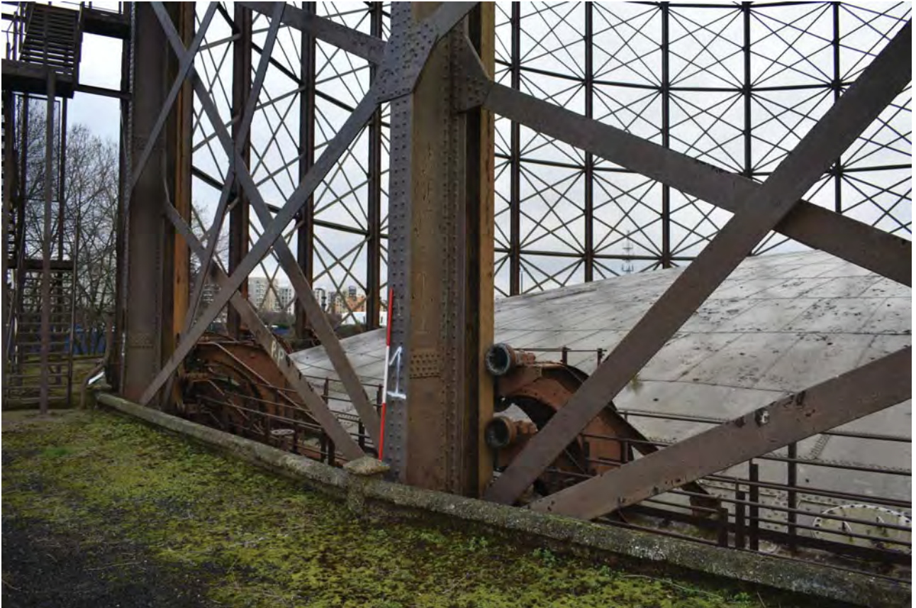
Plate 7: Gasholder No 1, detail of No 1 standard from the north
