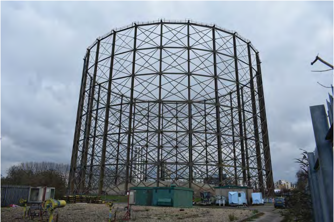
Plate 3: Gasholder No 1, general view from the south-west
