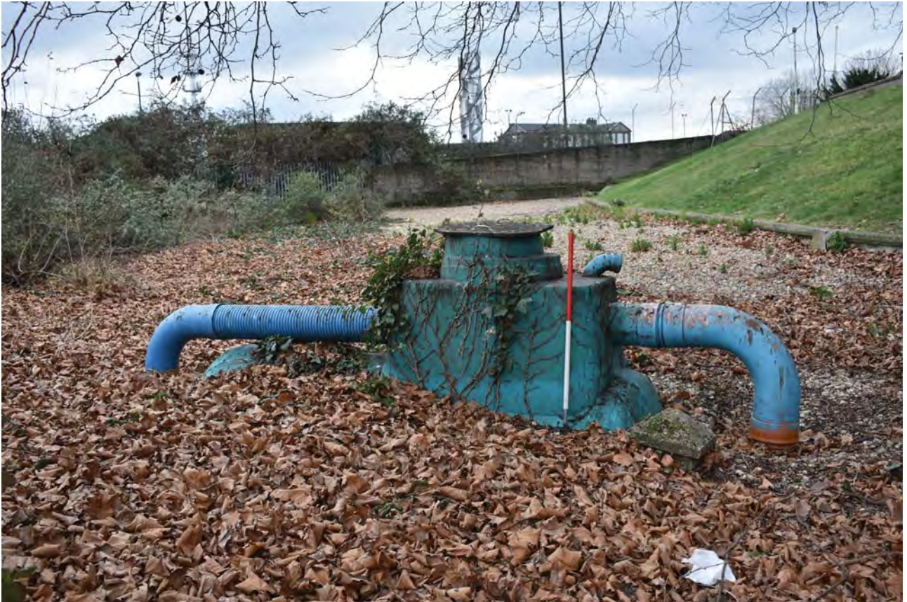
Plate 51: Pipework P, general view from the north
