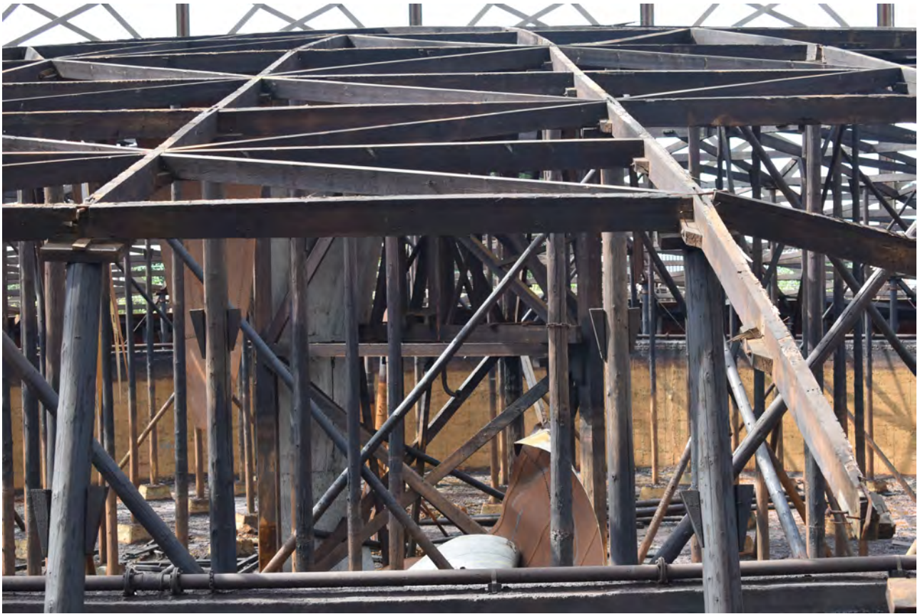
Plate 39: Gasholder No 1, detail of central triangular support framework, from the NNE
