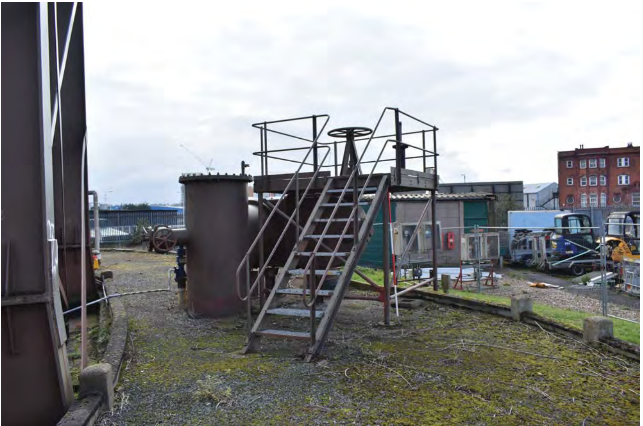
Plate 20: Gas Main, general view from the north-west
