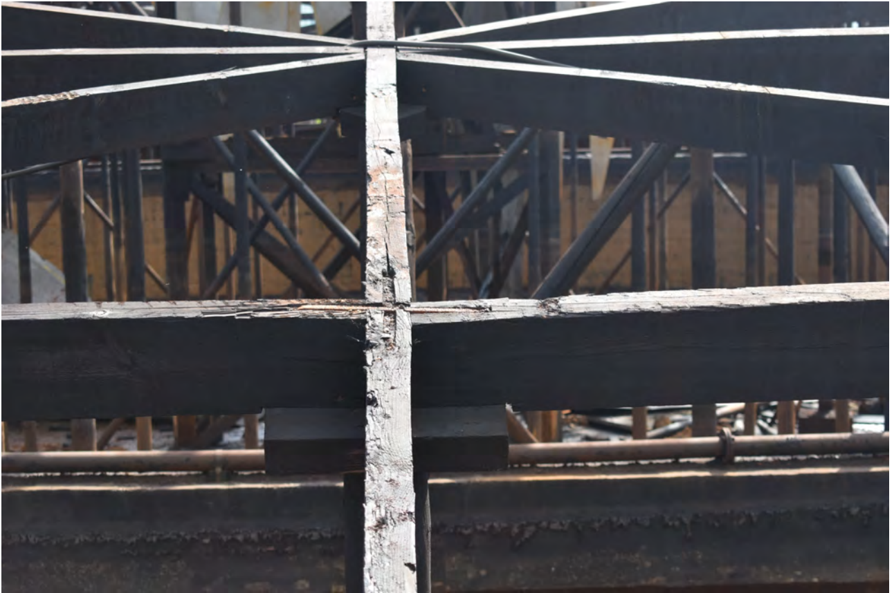
Plate 25: Gasholder No 1, detail of metal joint between spoke and ring timbers, from the WSW
