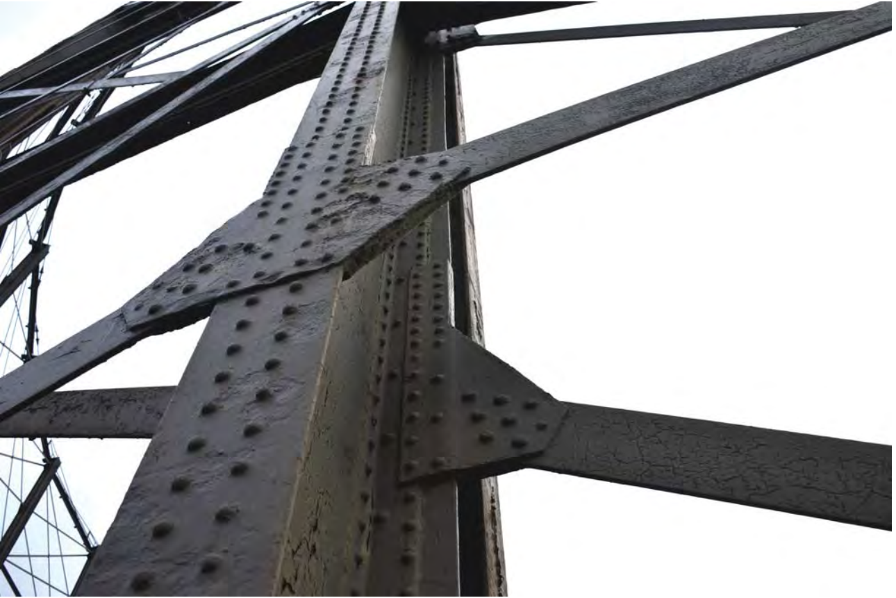
Plate 9: Gasholder No 1, detail looking up at No 1 standard from the north-west
