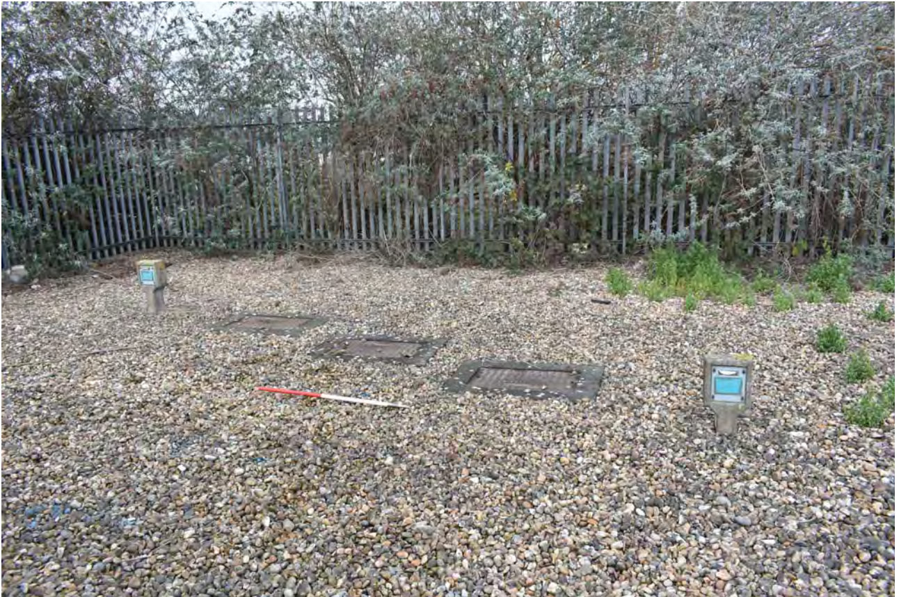
Plate 45: Manholes Ci, general view from the south
