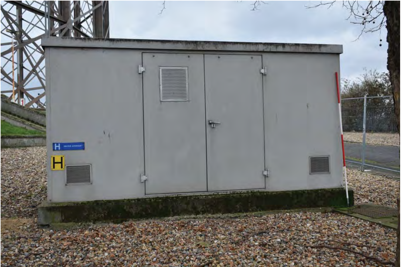
Plate 43: Building A, general view from the west
