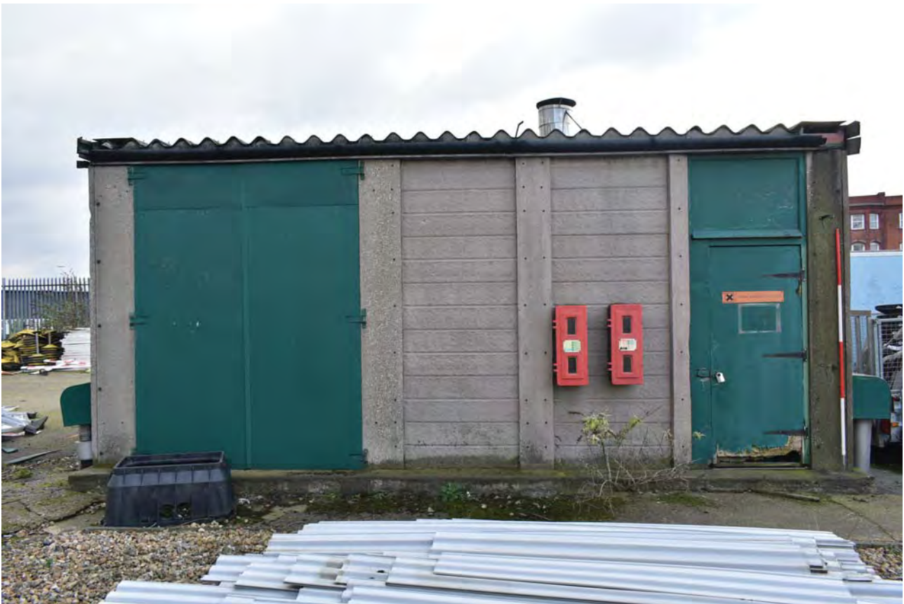
Plate 47: Building G, general view from the NNE
