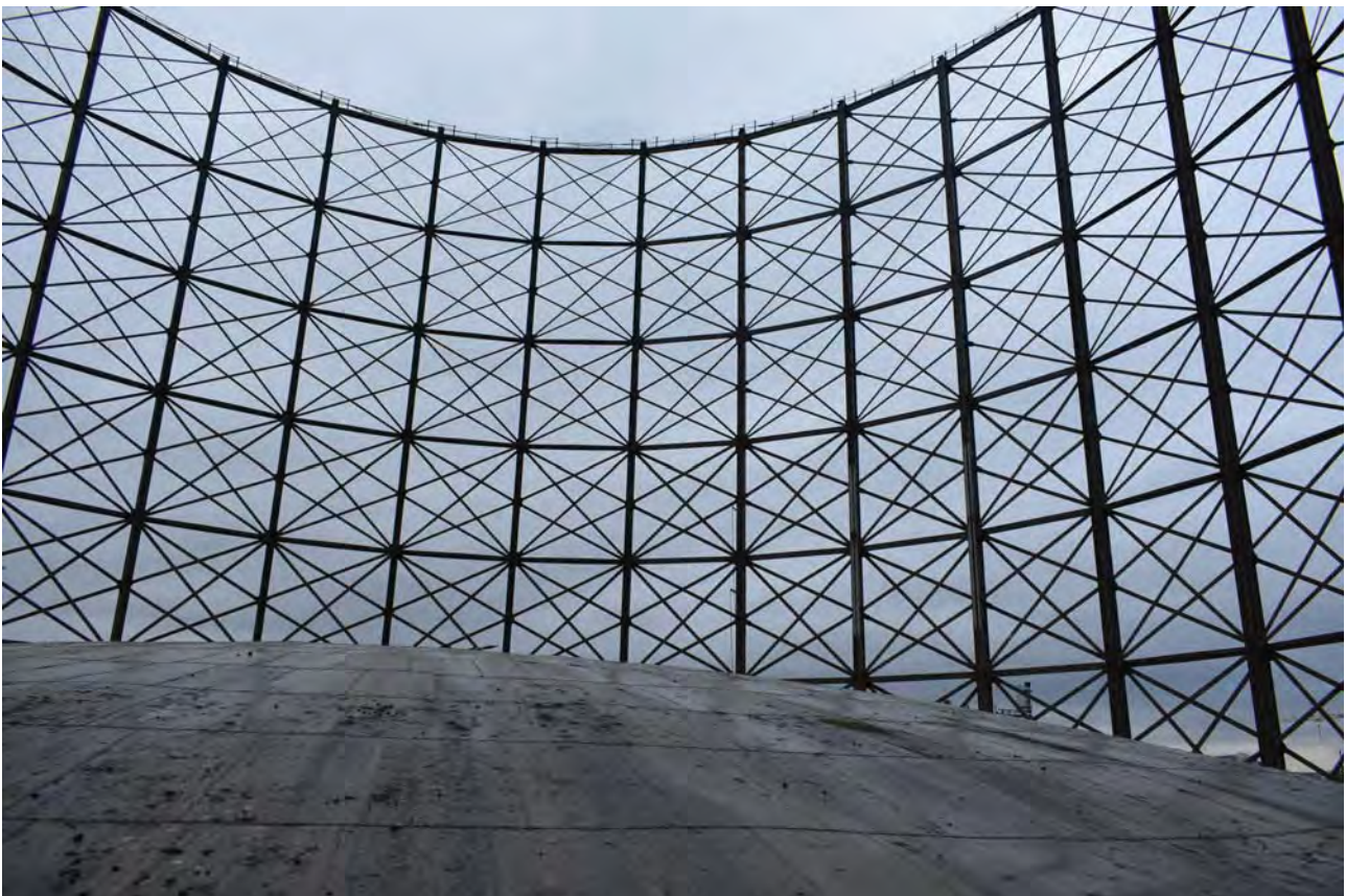
Plate 4: Gasholder No 1, detail of the frame from the NNE
