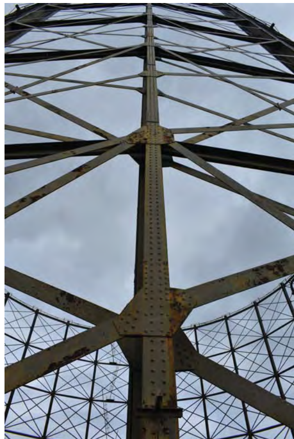
Plate 10: Gasholder No 1, detail looking up at No 17 standard from the south
