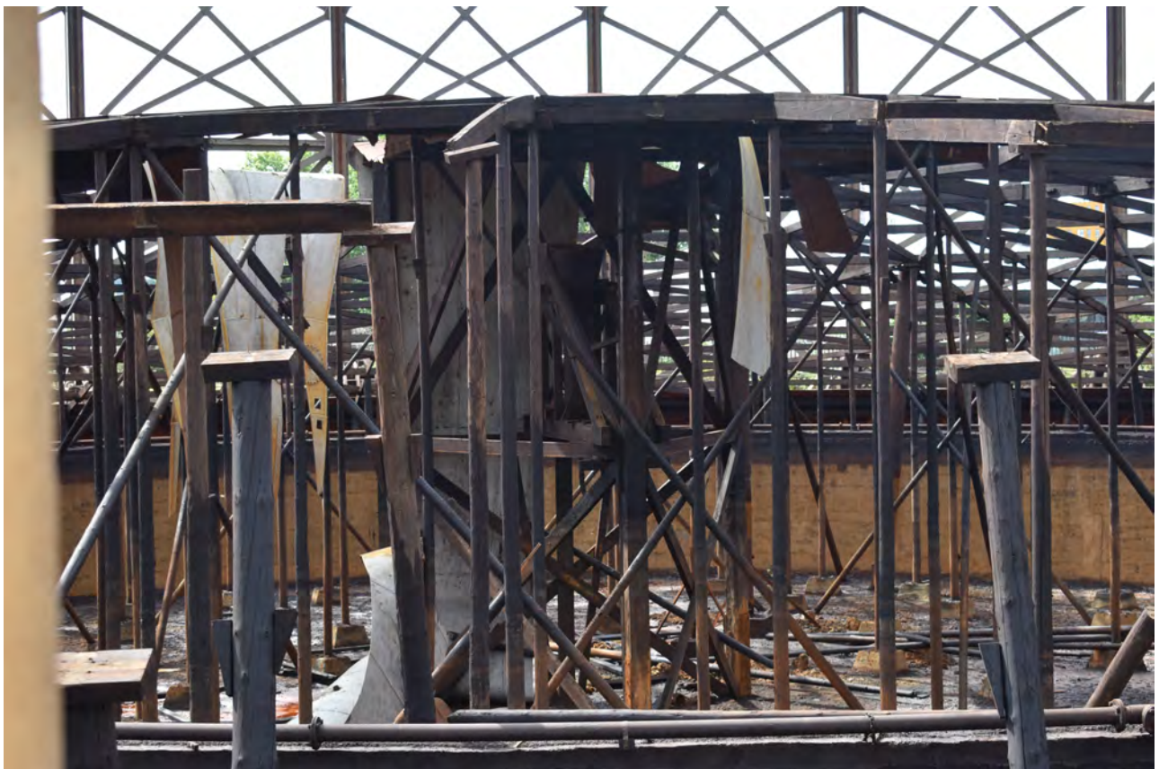
Plate 40: Gasholder No 1, detail of central triangular support framework, from the north
