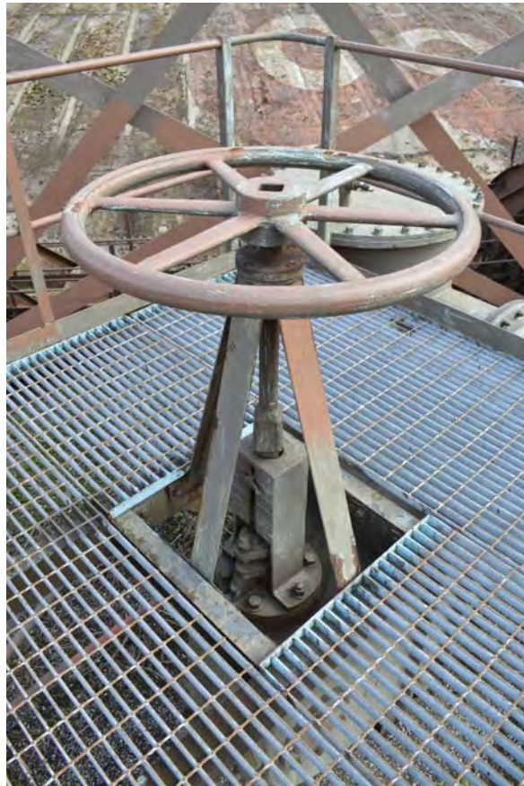
Plate 21: Gas Main, detail of the wheel from the west
