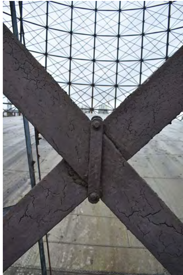
Plate 5: Gasholder No 1, close detail of the diagonal bracing from the NNE
