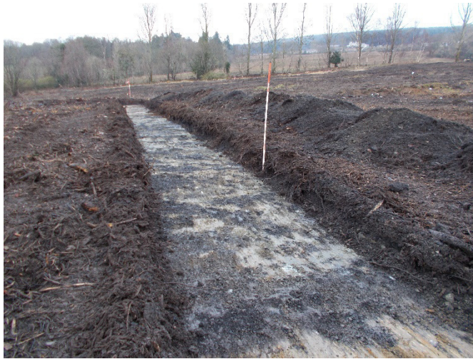
Plate 3: Post-excitation shot of Trench 1
