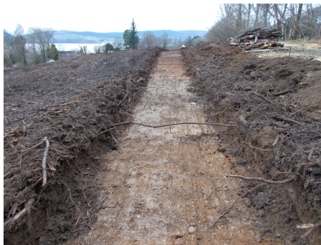
Plate 5: Post excavation shot of Trench 4
