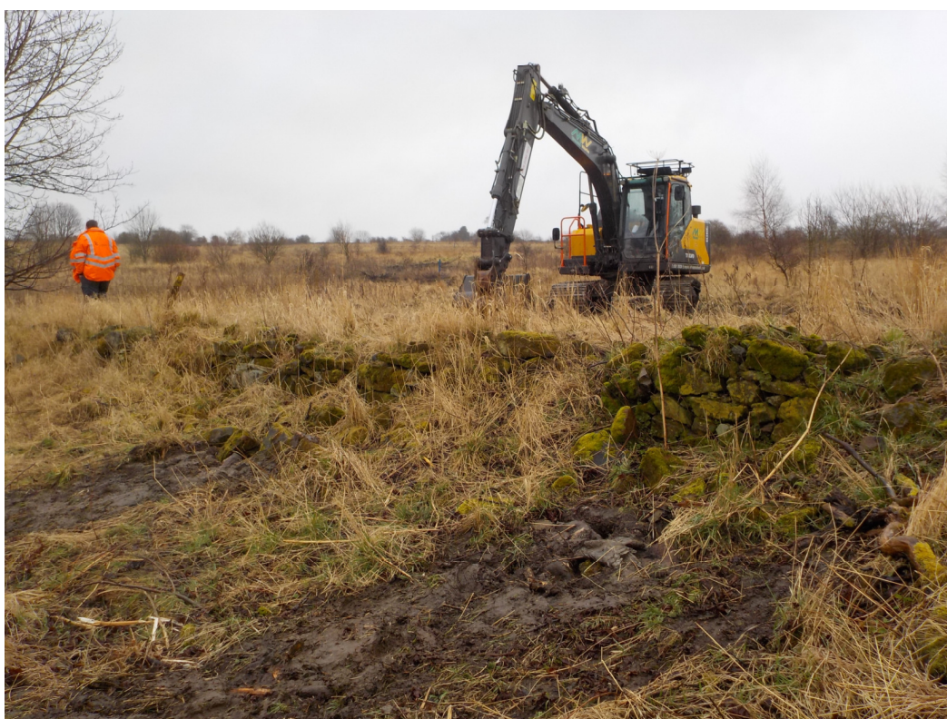
Plate 7: Demolition of section of historical wall [003]
