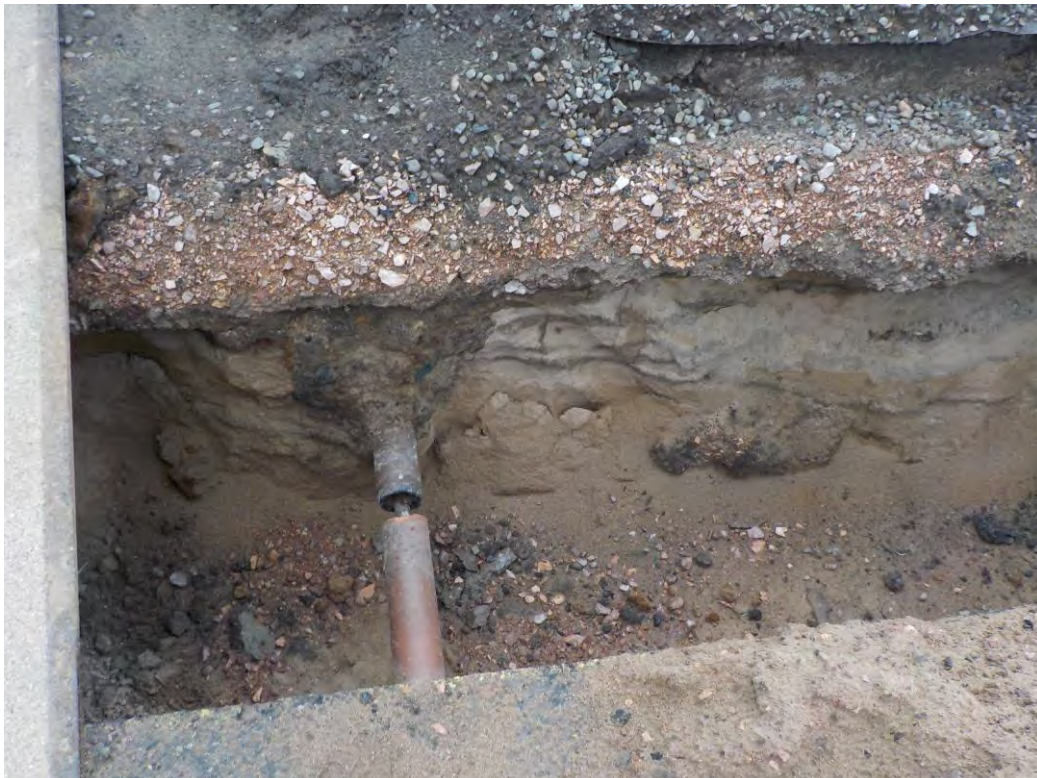
Plate 1 Existing service and new service track
