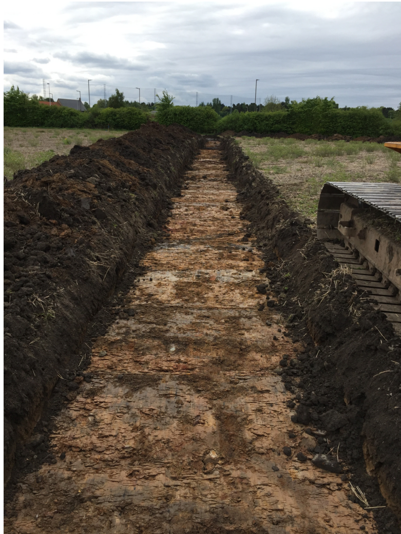
Plate 1 Trench 4 post excavation
