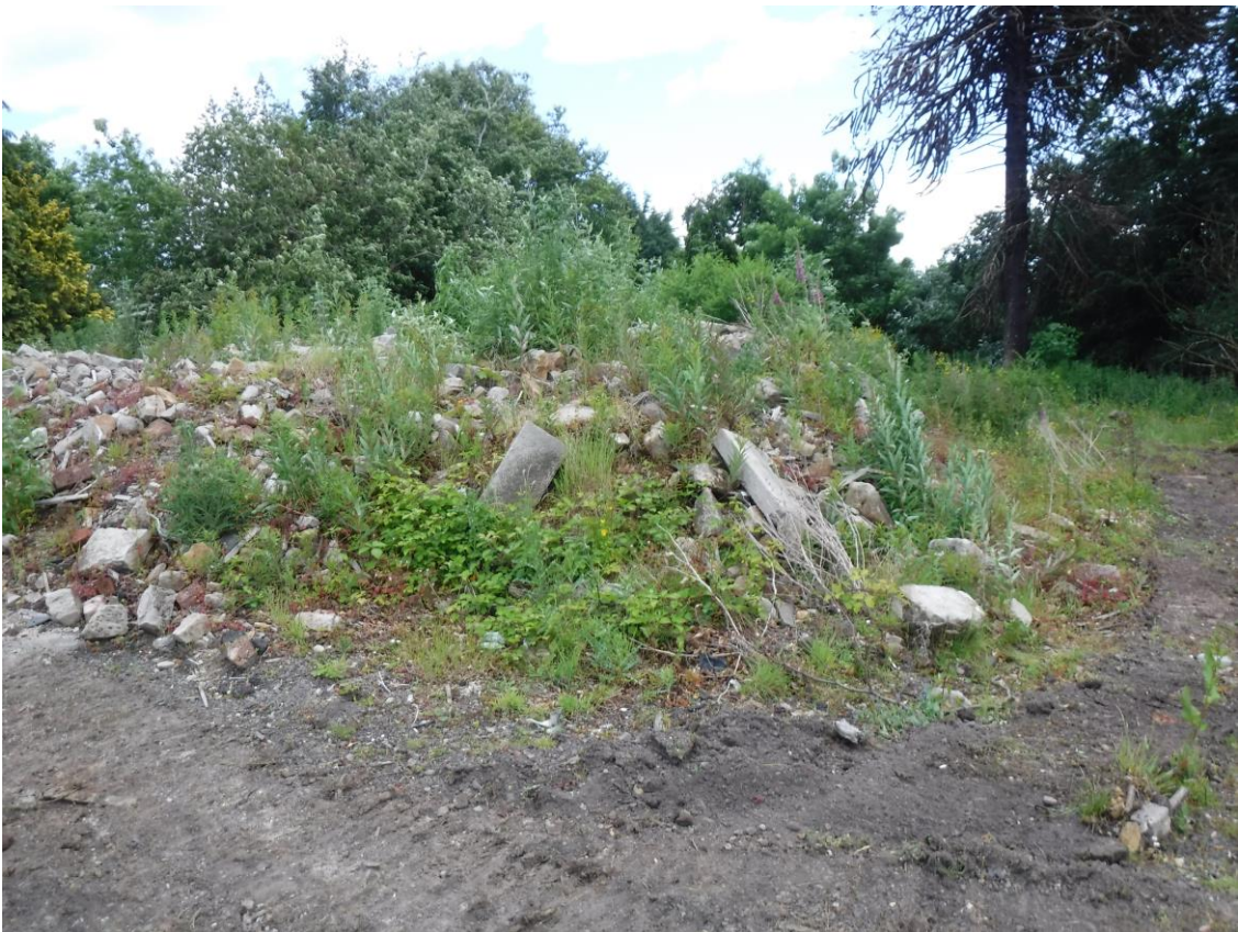
Plate 1 Demolition rubble over Mayshade/Ashgrove House
