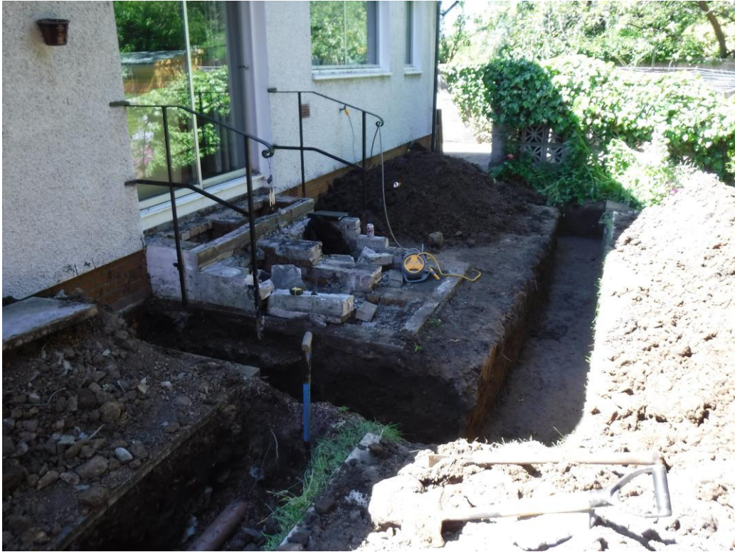
Plate 1 View of foundation trench from West
