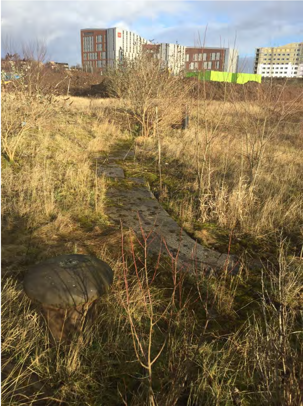
Plate 2: View of dry dock in situ with development in background
