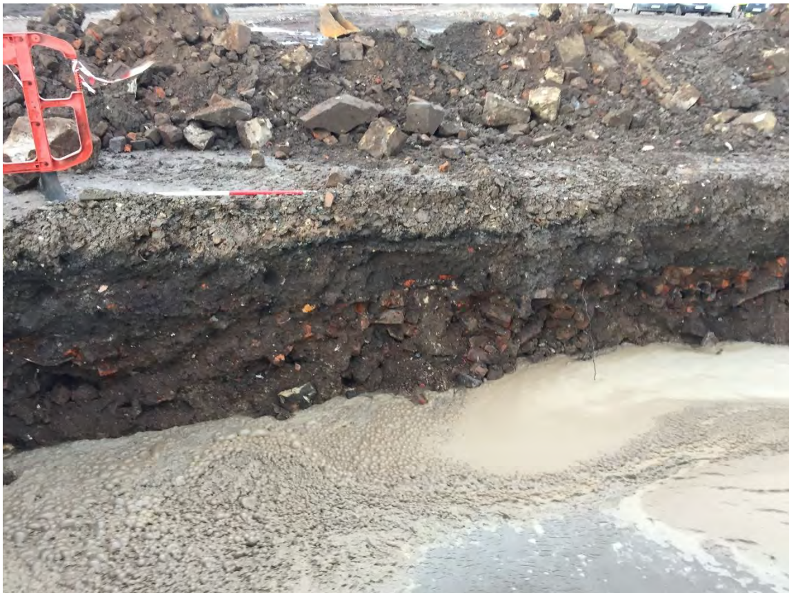
Plate 1: View of Excavation for Septic Tank
