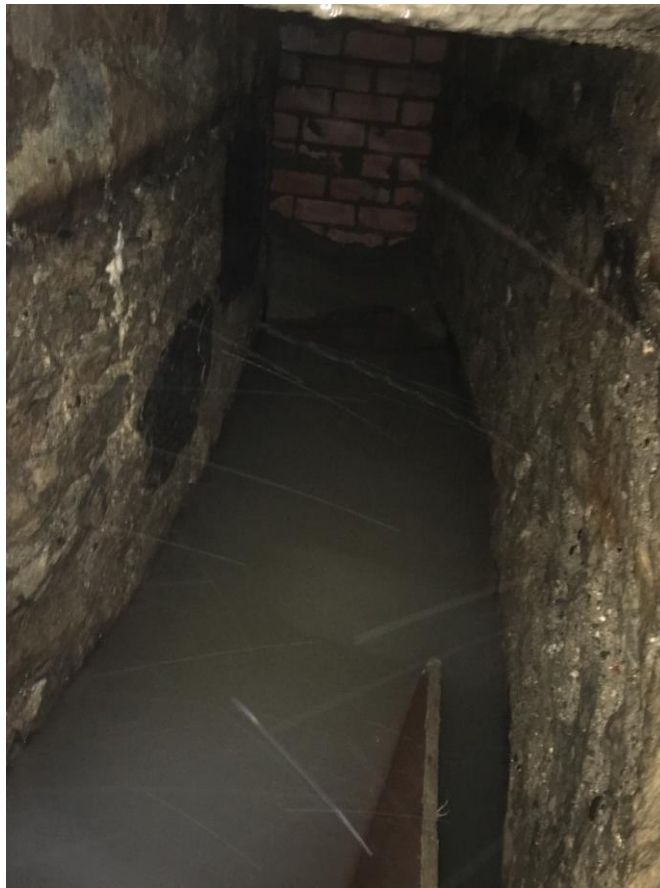
Plate 5 – Detail of Culvert [008] showing brick manhole
