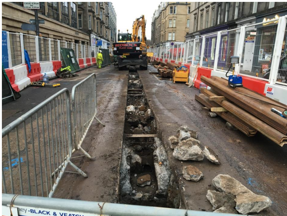
Plate 1 – N-S Metal beams encased in concrete
