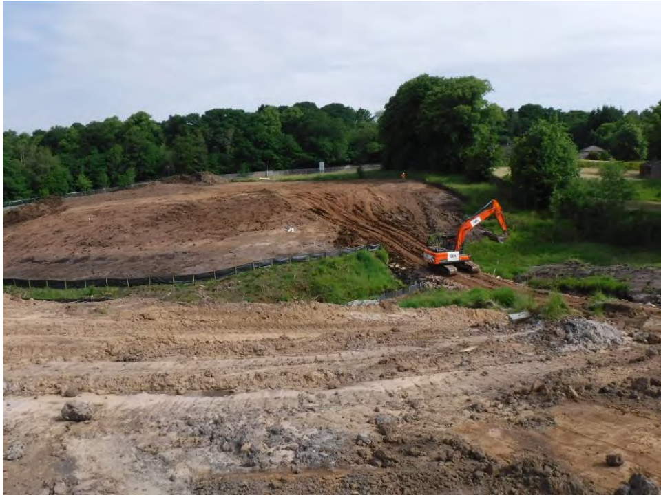
Plate 6: General shot of northern area stripped
