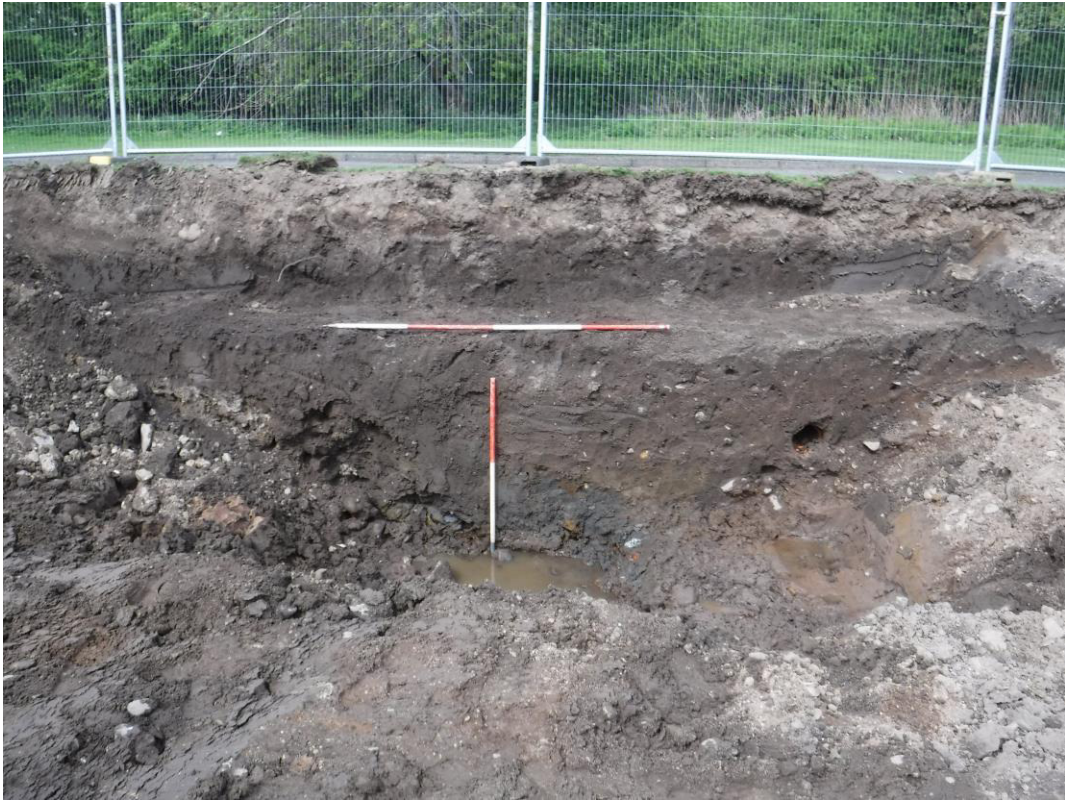
Plate 2 View of section through mill lade [004] from S
