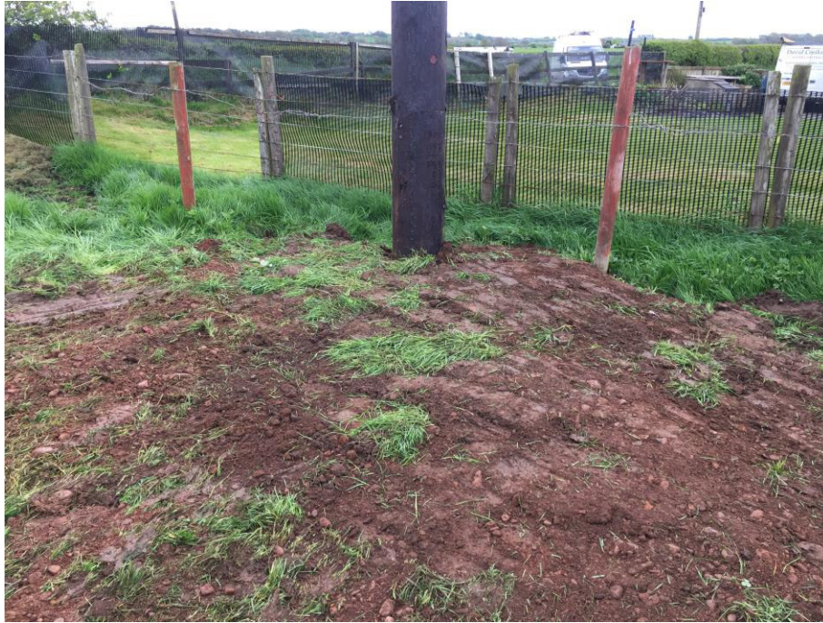
Plate 1 – View of new power pole after excavation
