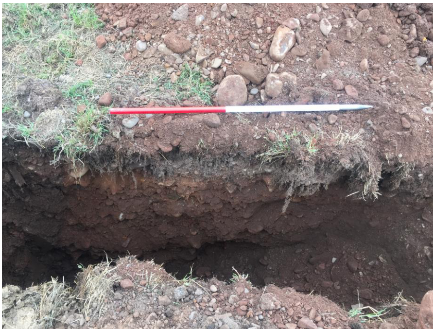
Plate 2 – Trench for the removal of redundant power pole
