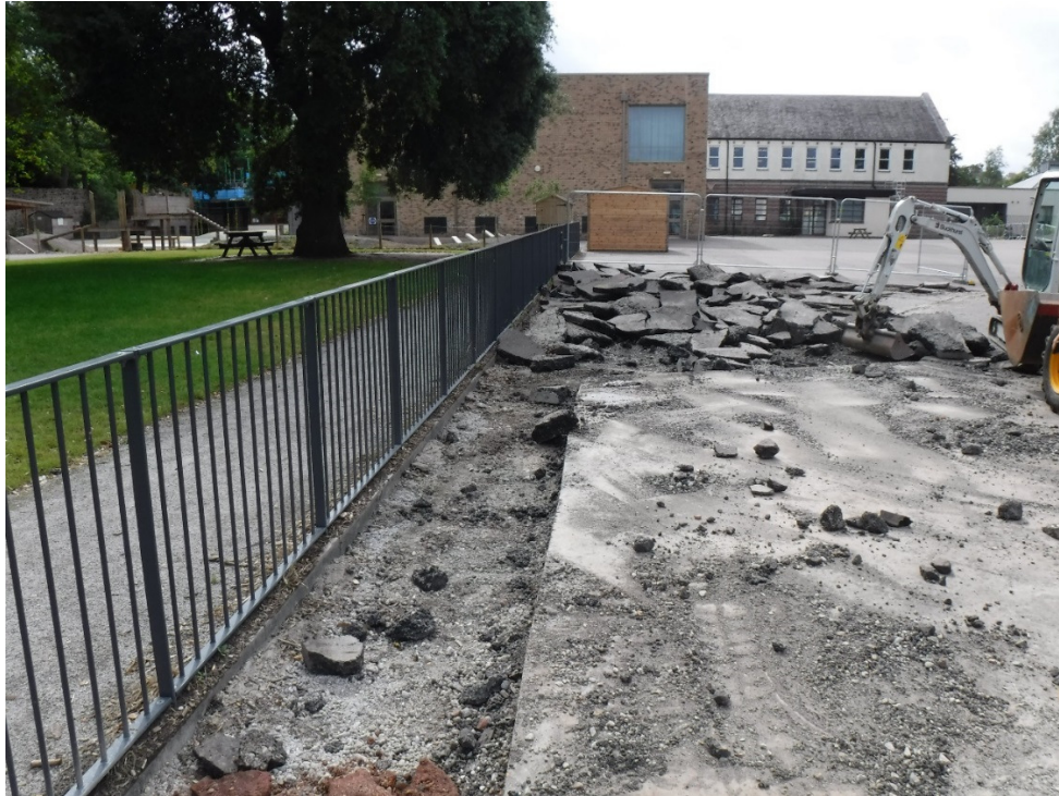
Plate 1: General view of service track
