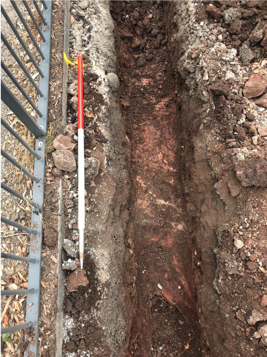
Plate 2: Exposed brick path within service track
