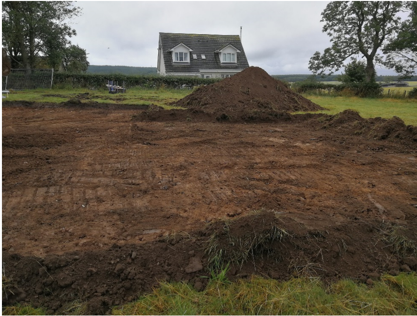
Plate 3: Post excavation shot facing South
