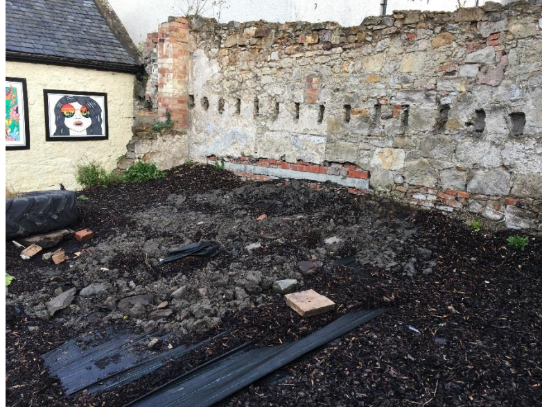
Plate 2: Pre-excitation shot of site east showing ground floor beam slots of former building
