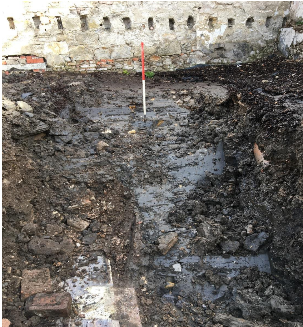
Plate 4: Trench 1 showing boulder clay and overlying made ground
