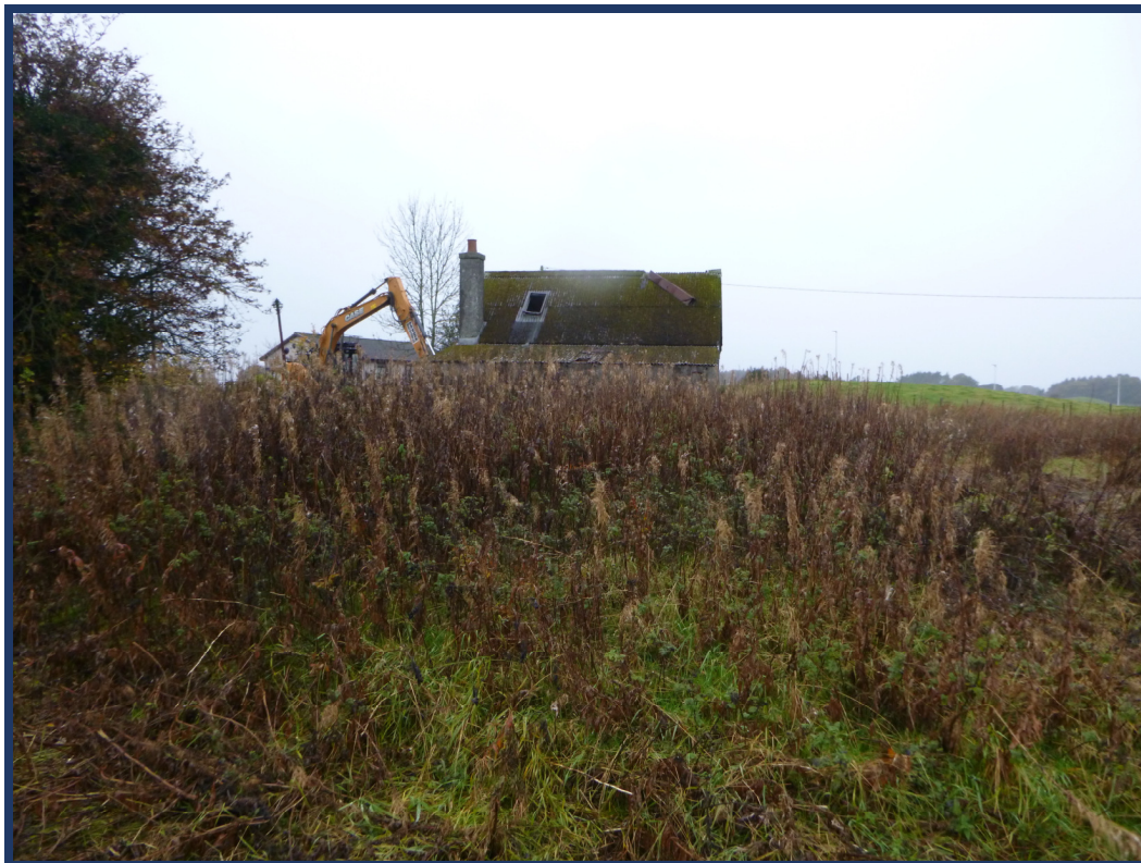
Plate 1: General view of site conditions
