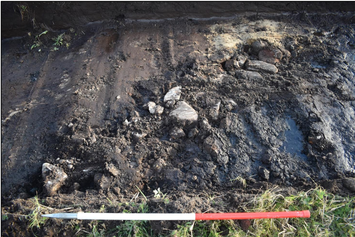
Plate 4: Trench 6 example of rubble drain, facing south-south-east
