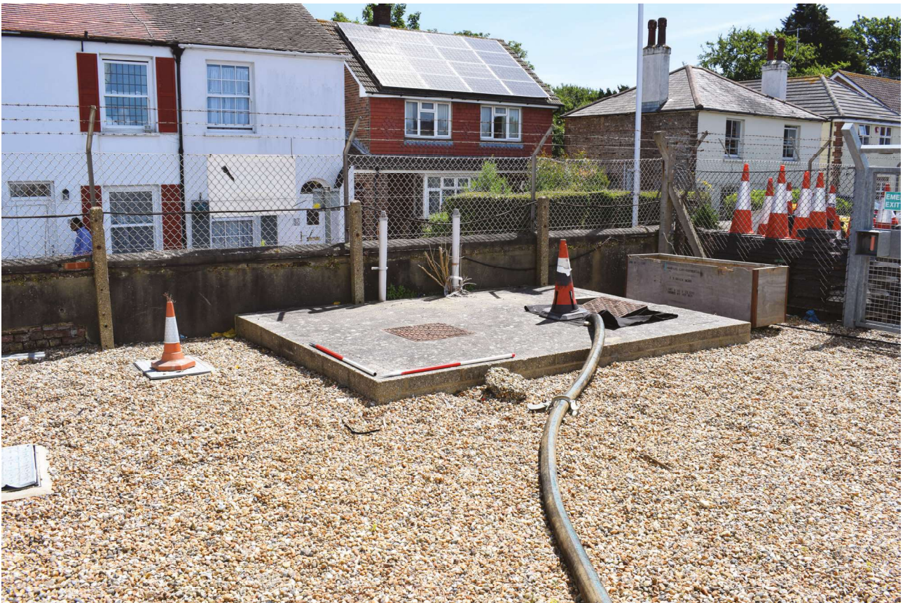
Plate 25: Park Road, Worthing, Structure 2, general view from the south-west
