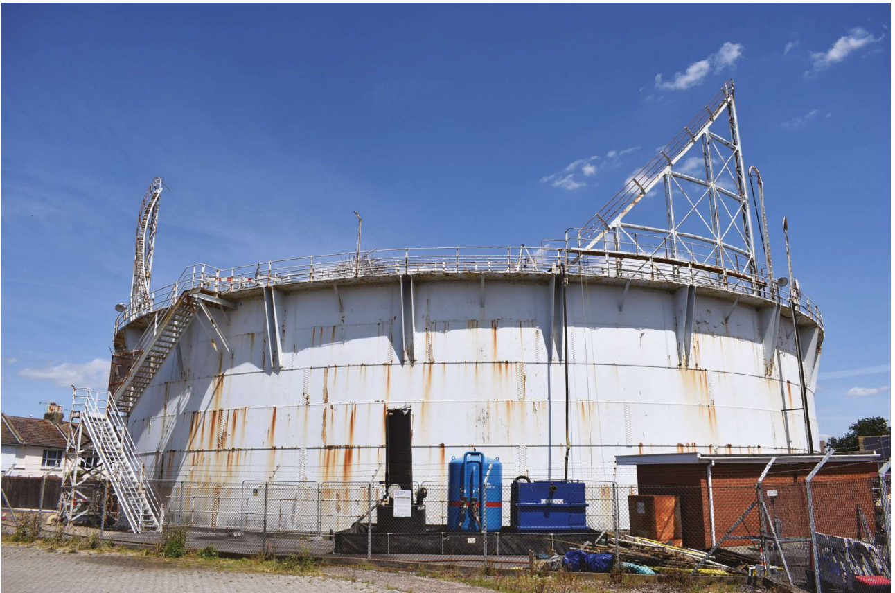
Plate 4: Park Road, Worthing, general view of the gasholder from the WSW
