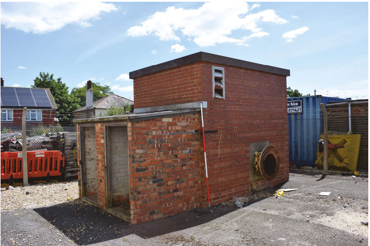
Plate 26: Park Road, Worthing, Structure 3, general view from the south-west
