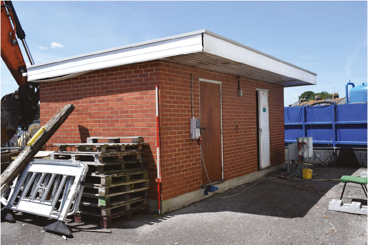
Plate 27: Park Road, Worthing, Structure 6, general view from the east
