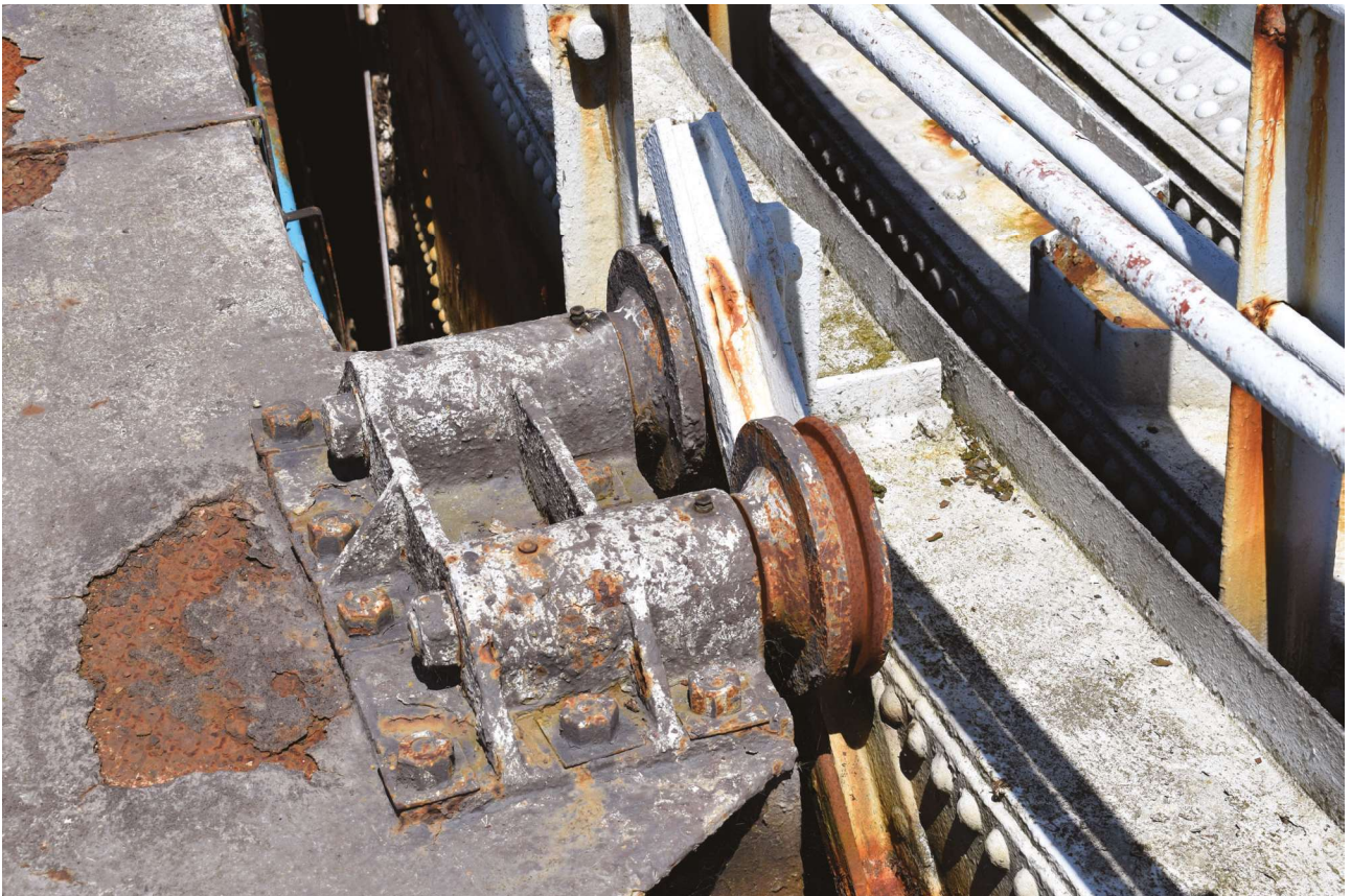
Plate 18: Park Road, Worthing, detail of guided rollers from the south-west
