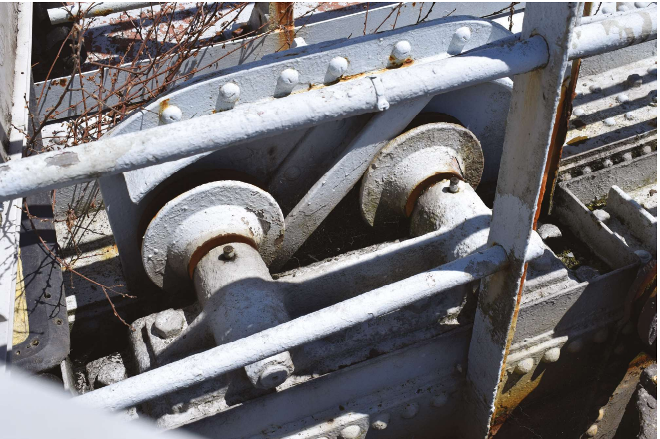
Plate 20: Park Road, Worthing, detail of guided rollers from the north-west
