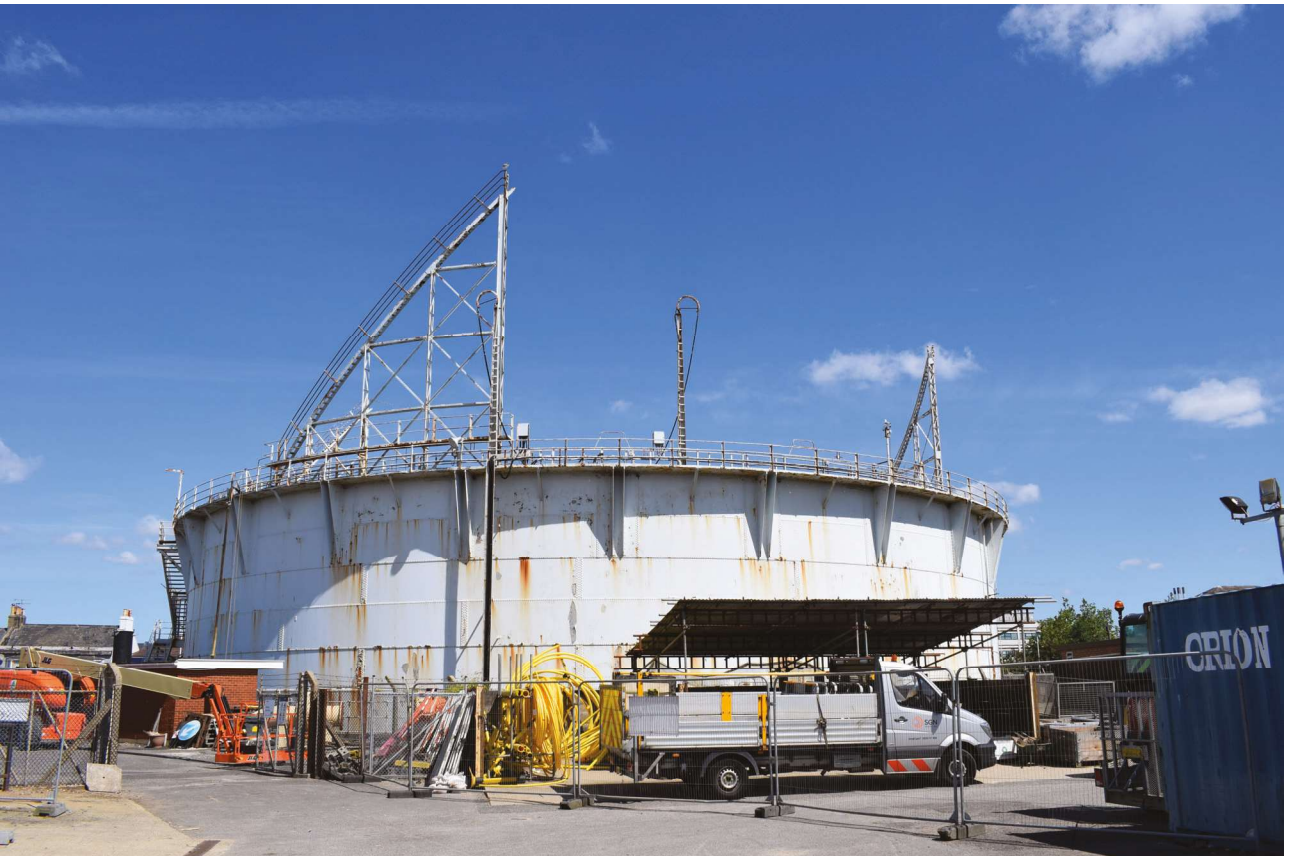
Plate 2: Park Road, Worthing, general view of the gasholder from the south
