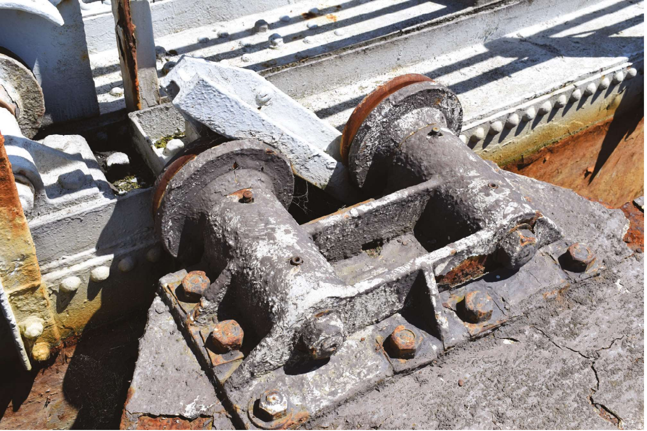
Plate 19: Park Road, Worthing, detail of guided rollers from the north-west
