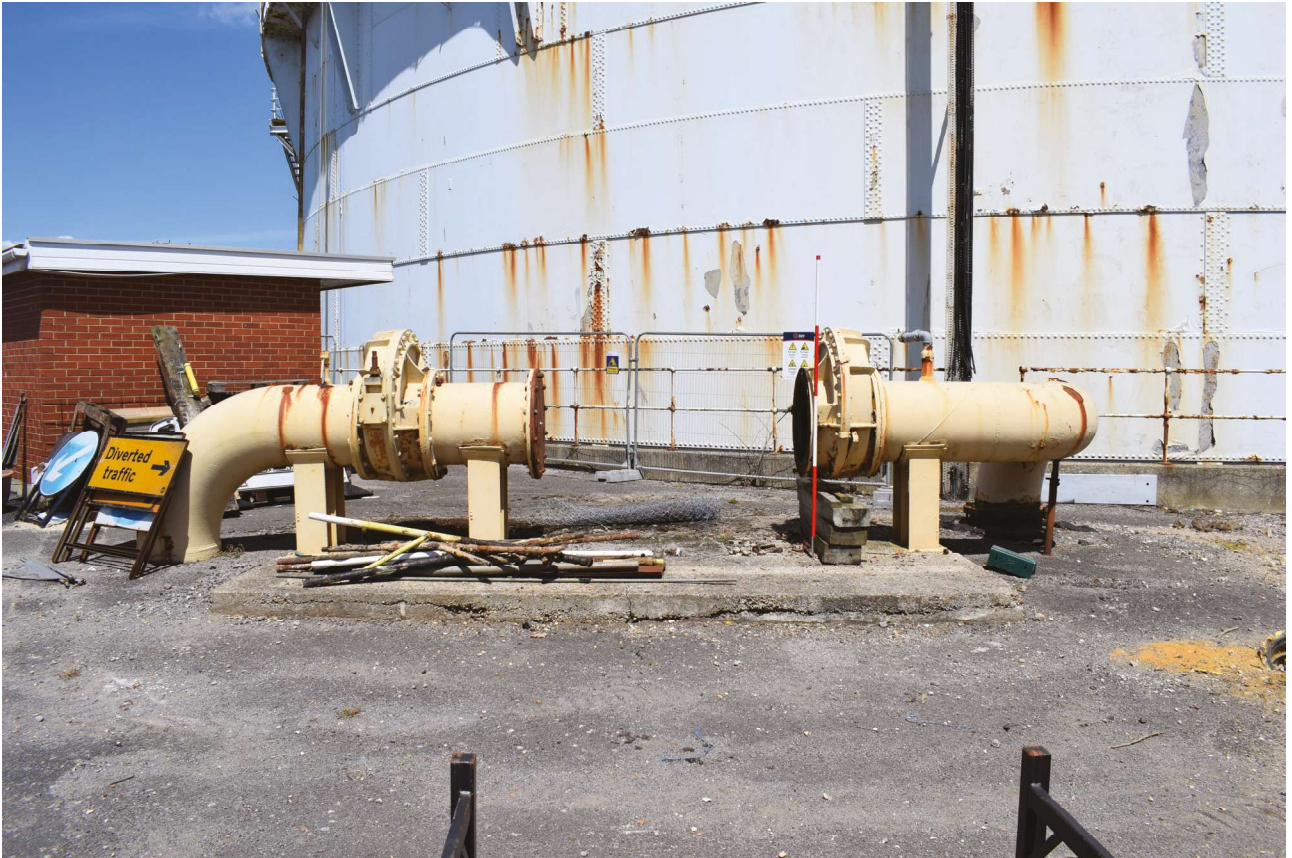
Plate 15: Park Road, Worthing, Structure 5, general view of pipework from the south
