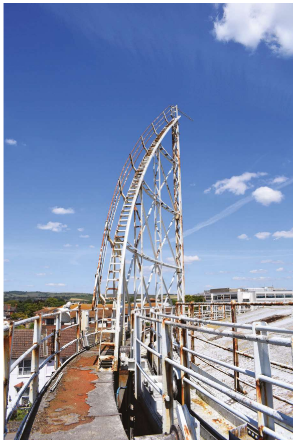
Plate 22: Park Road, Worthing, detail of the stair from the south
