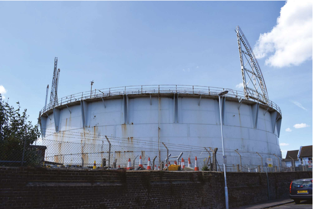
Plate 1: Park Road, Worthing, general view of the gasholder from the south-east
