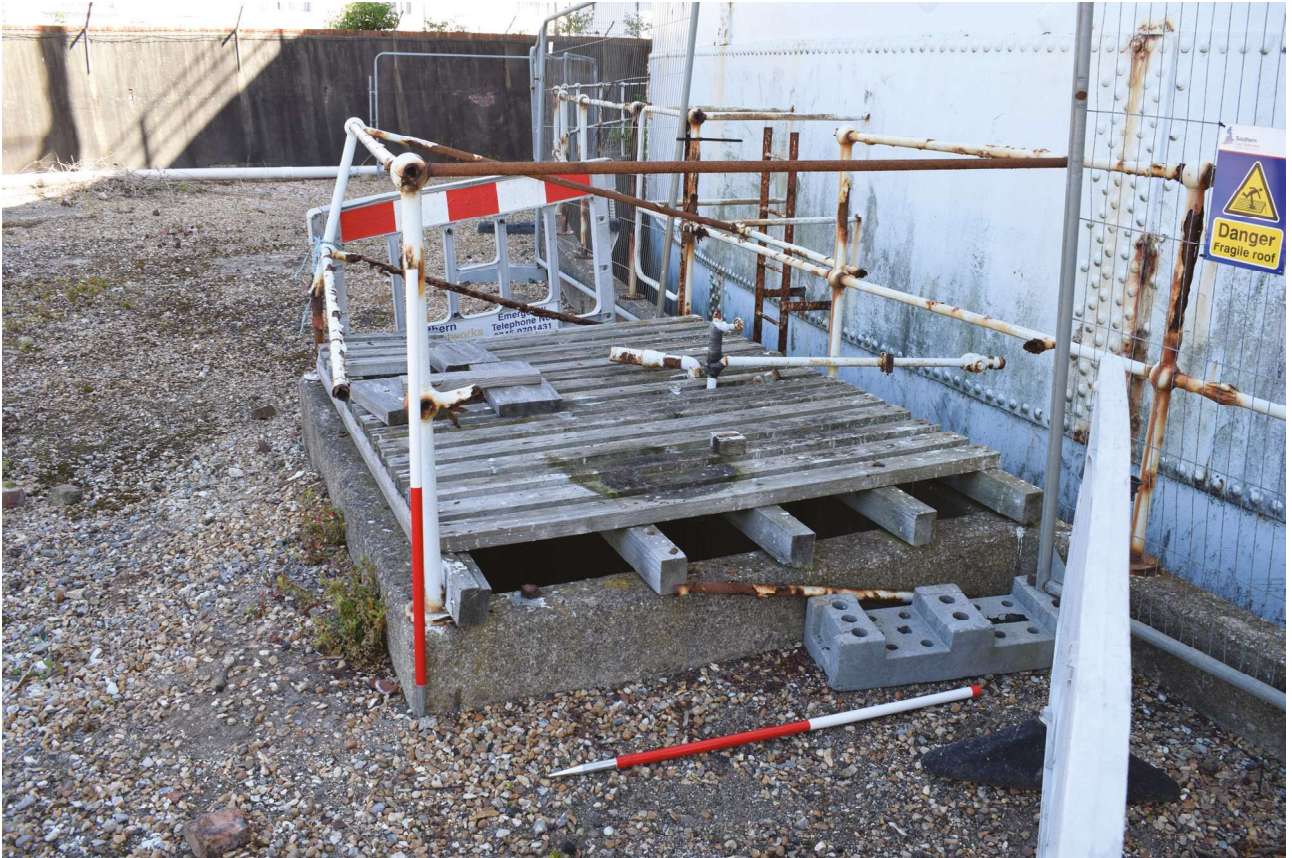
Plate 17: Park Road, Worthing, Structure 7, general view from the south-west
