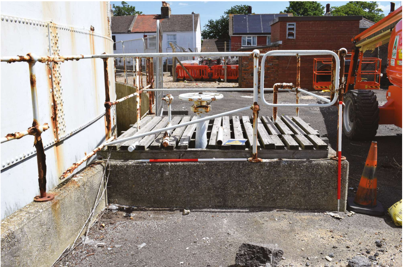
Plate 12: Park Road, Worthing, Structure 4, general view from the WSW
