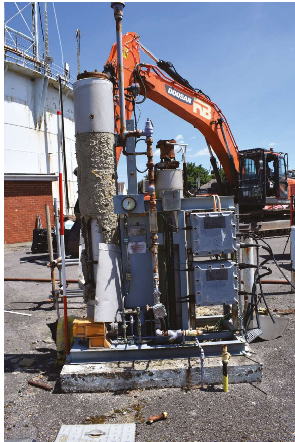
Plate 33: Park Road, Worthing, Structure 12, general view from the SSE
