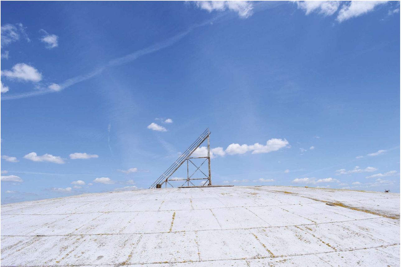
Plate 21: Park Road, Worthing, general view of the stair from the south-west
