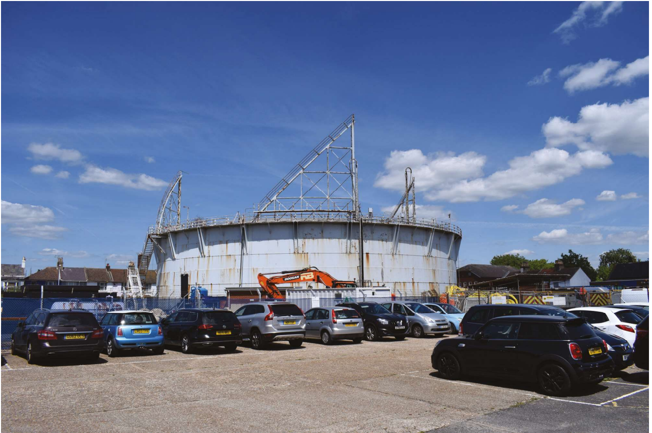
Plate 3: Park Road, Worthing, general view of the gasholder from the south-west
