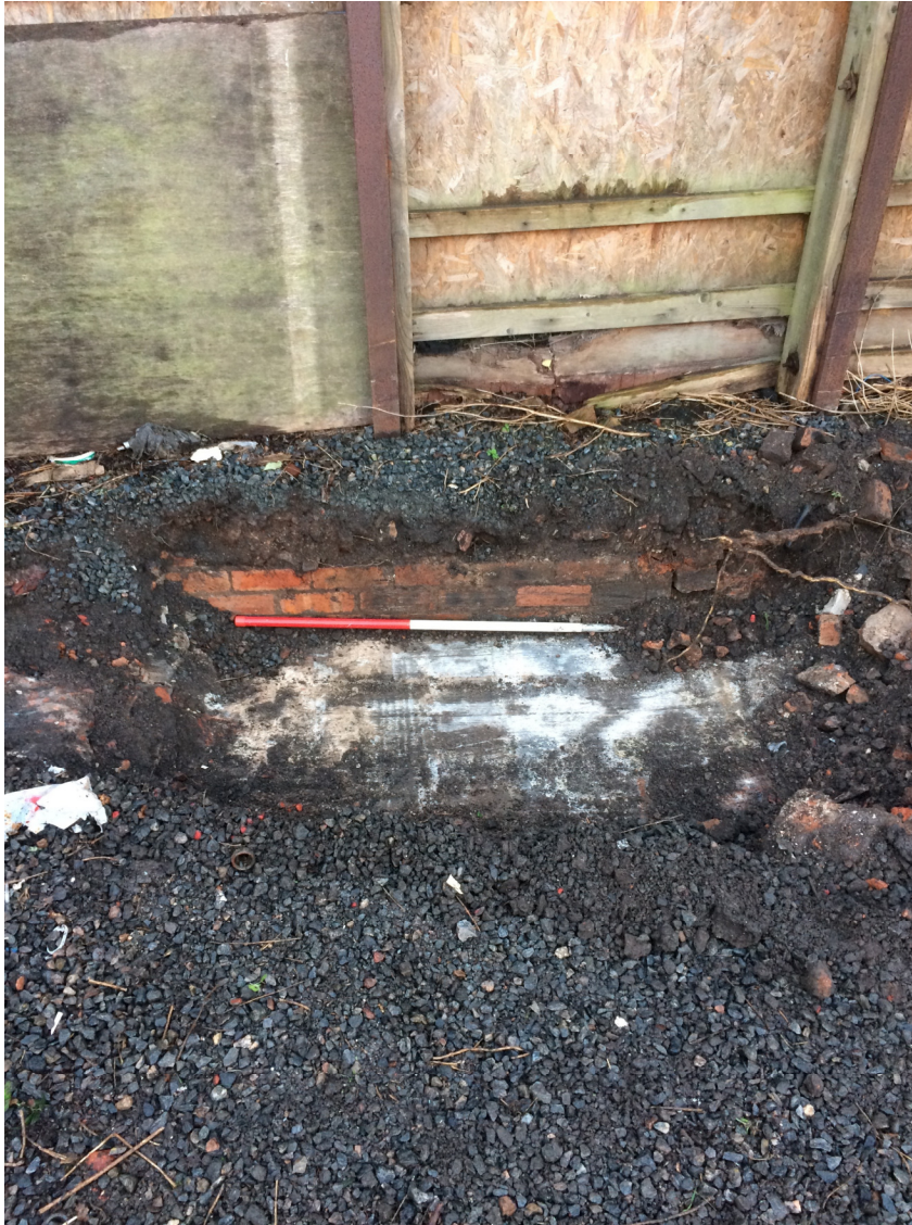
Plate 2 Brick wall and concrete floor fragment
