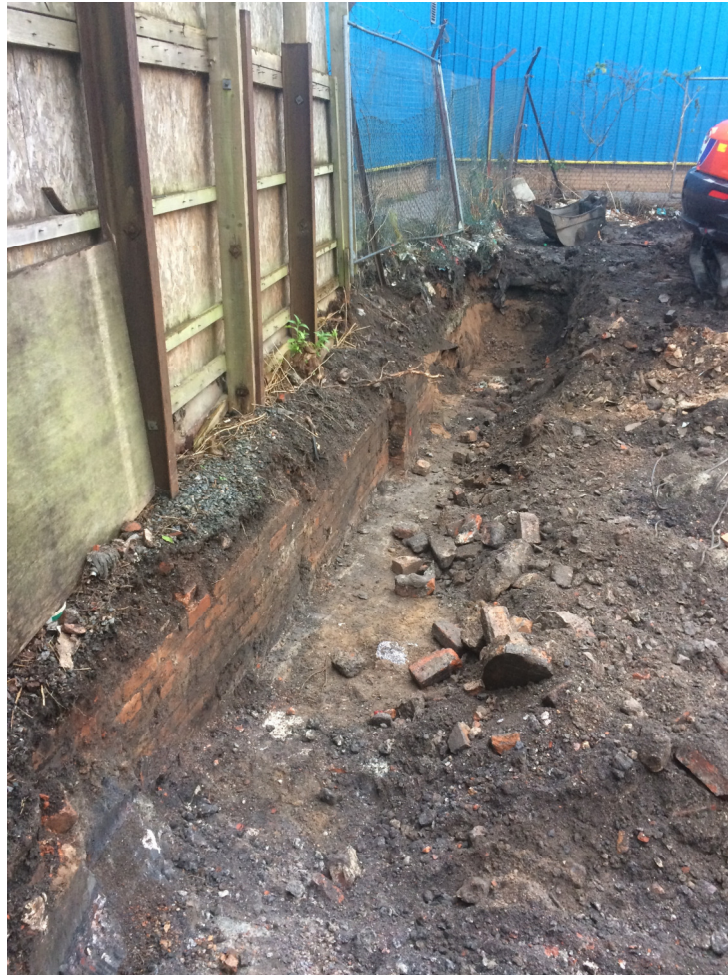
Plate 1 Brick Boundary Wall fragment
