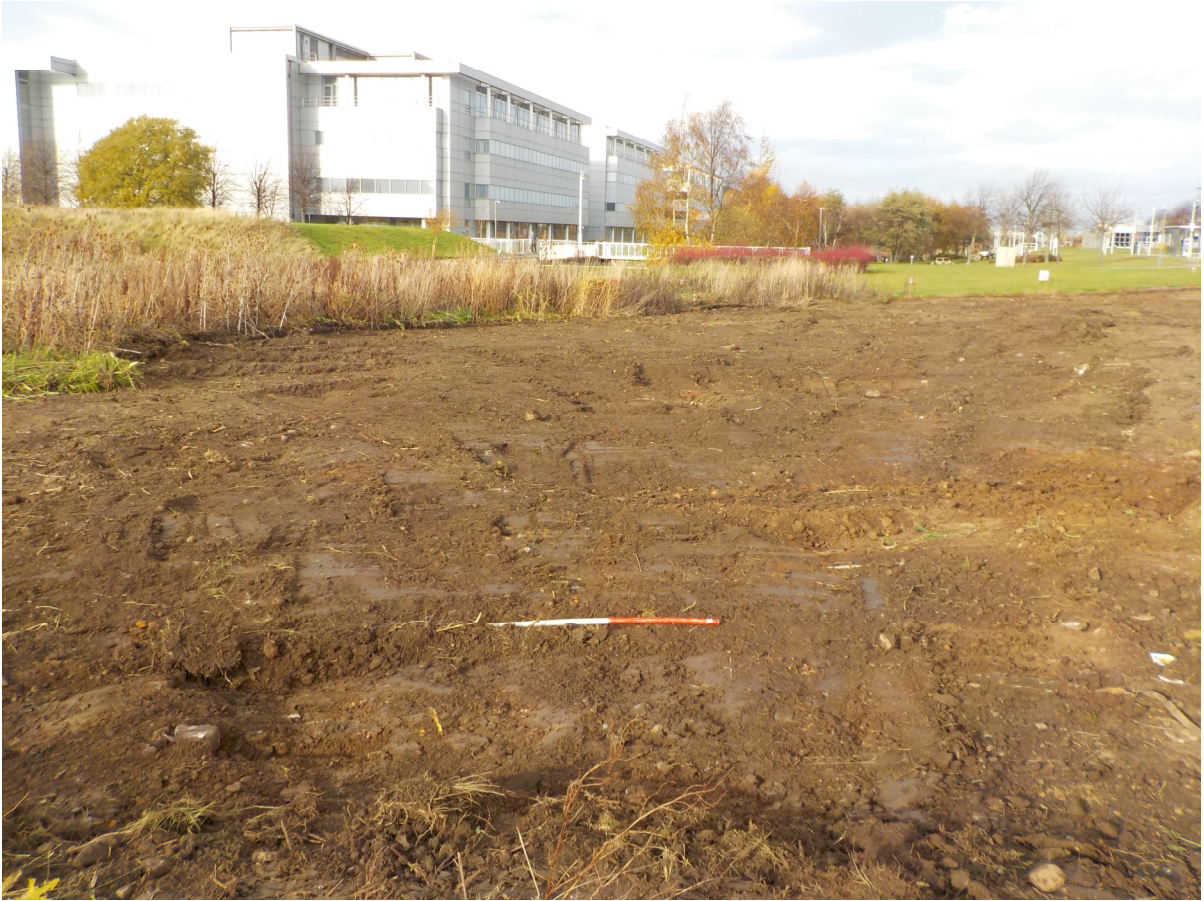
Plate 1: General view of the Area 1 after it had been stripped.
