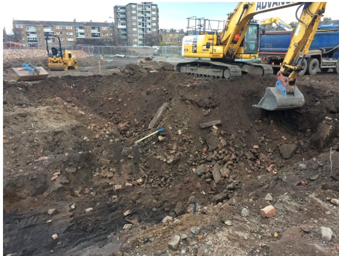
Plate 1 SUDS Area under excavation
