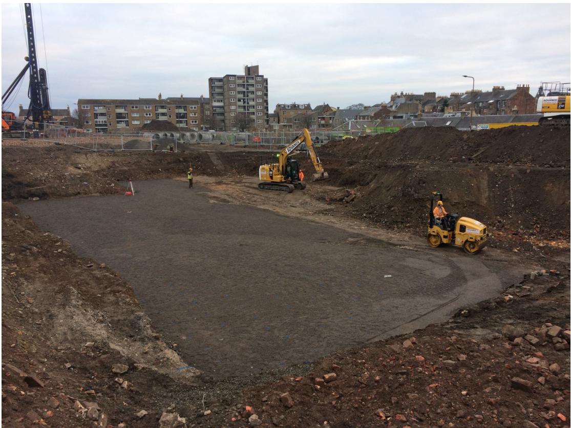
Plate 4 SUDS Area post excavation
