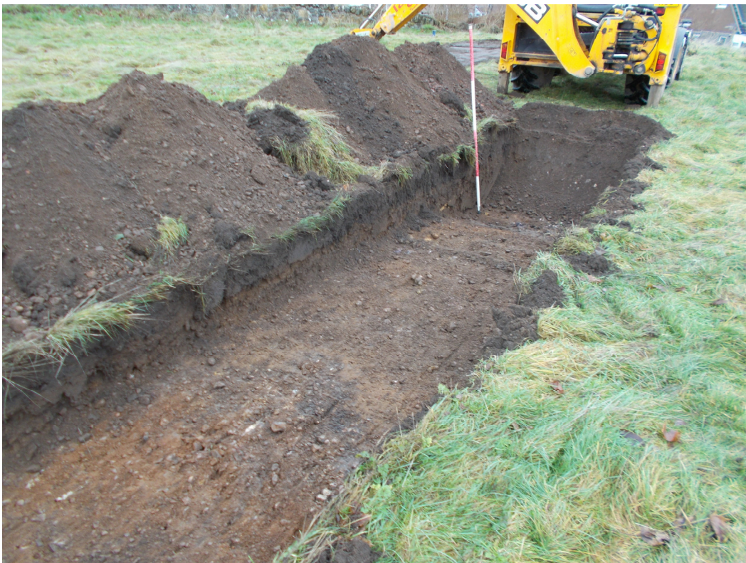
Plate 3 Trench 3 showing natural slope at north-western end
