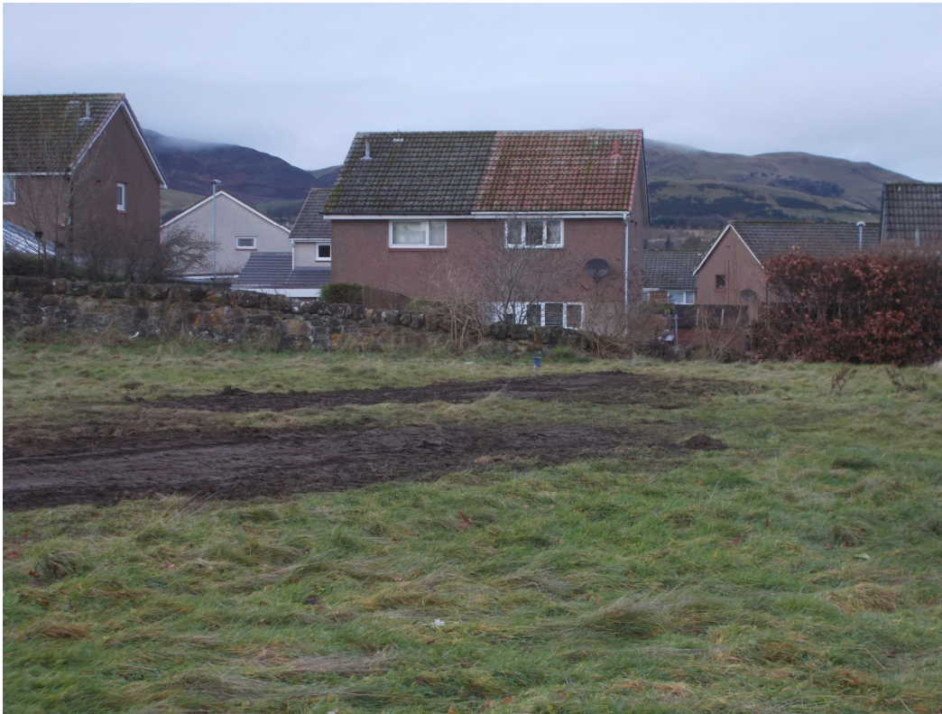
Plate 6 backfilled trenches 2&3 showing built up level of playing field against natural slope.
