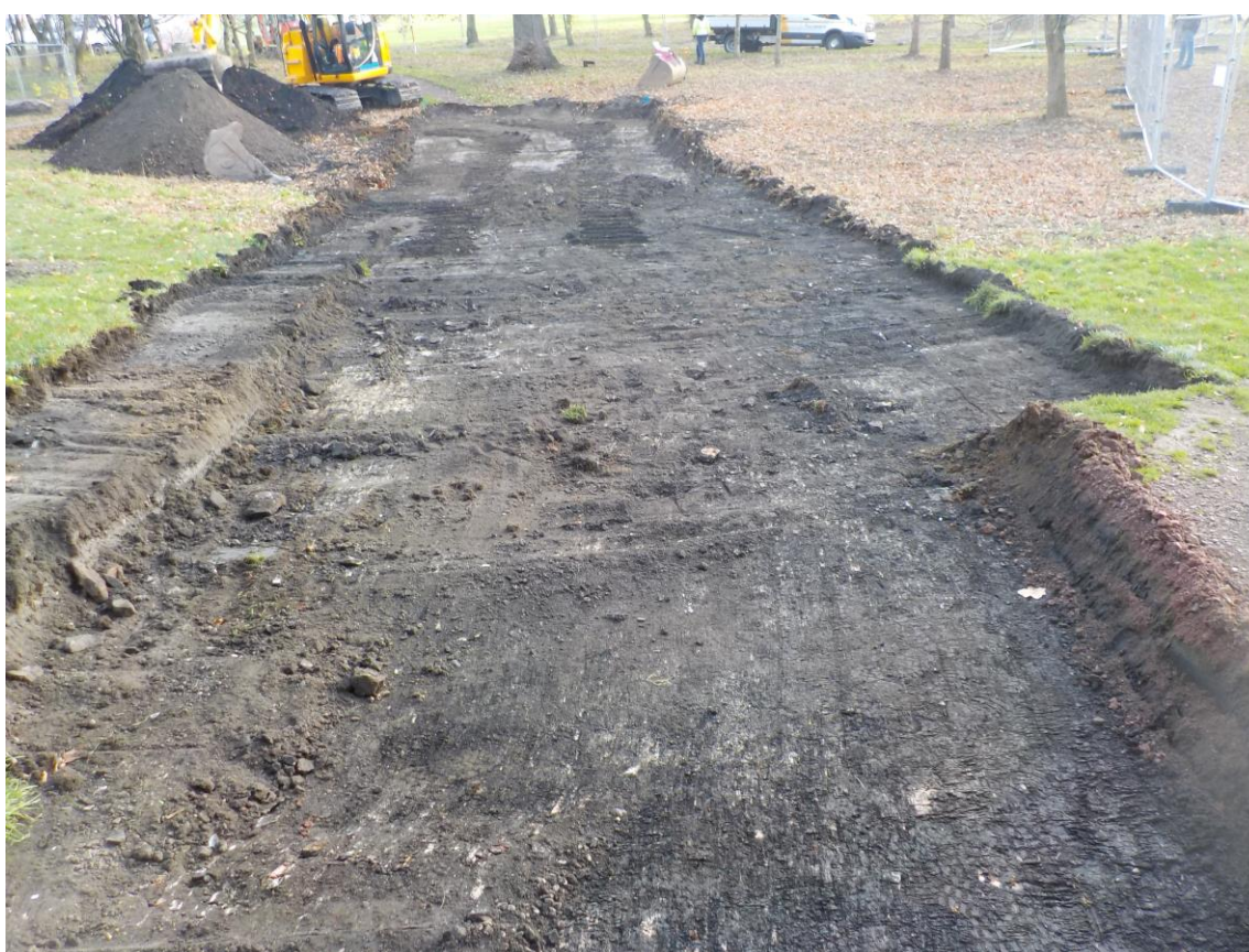
Plate 1 View of section pipe trench during topsoil stripping
