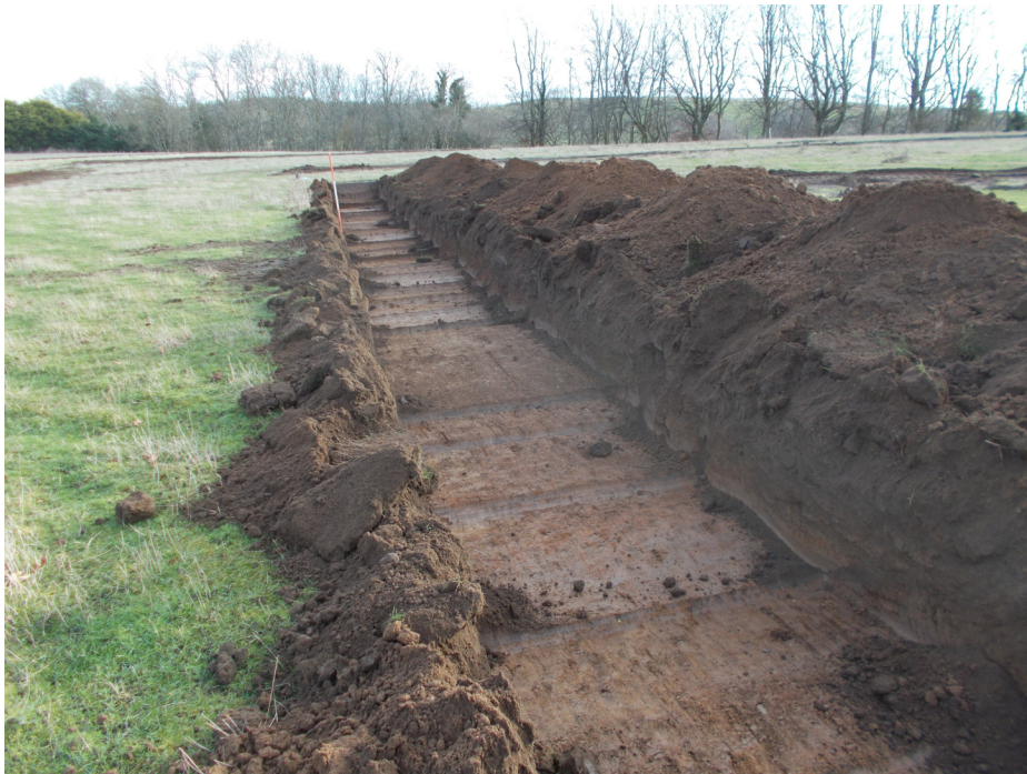
Plate 4 Trench 8 post excavation
