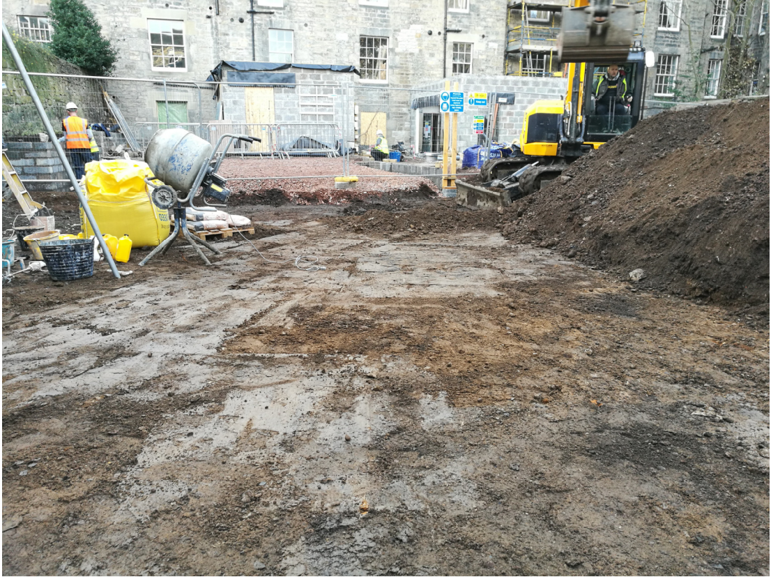
Plate 1 The site under excavation
