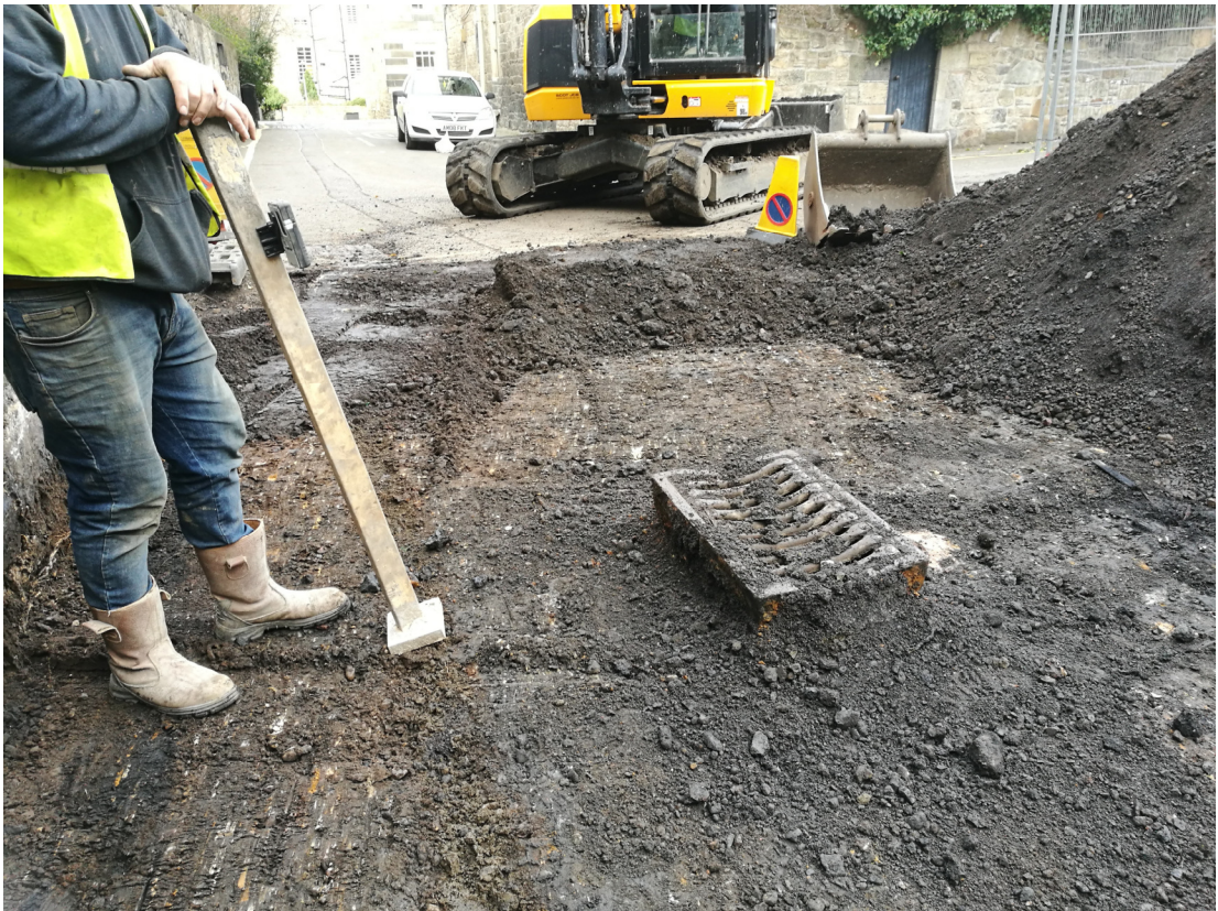
Plate 2 Exposed modern drain
